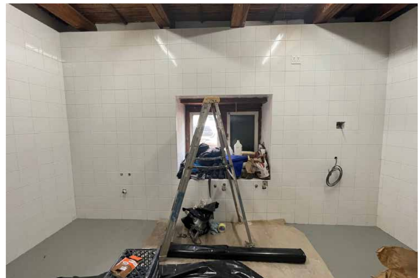
Figure 14. Kitchen and Scullery (RSA, 2022)
