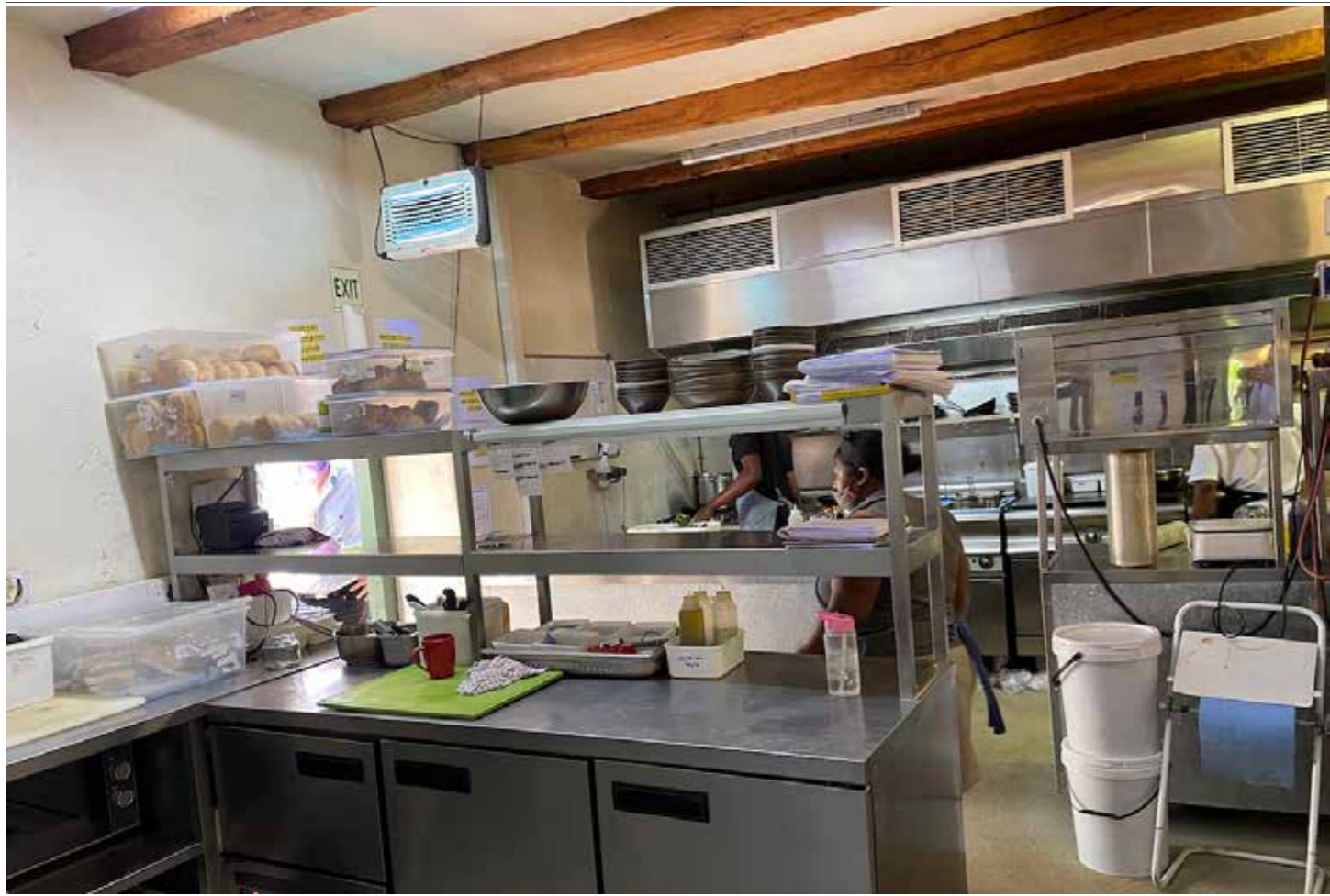
Figure 7. Kitchen and Scullery (RSA, 2022)
