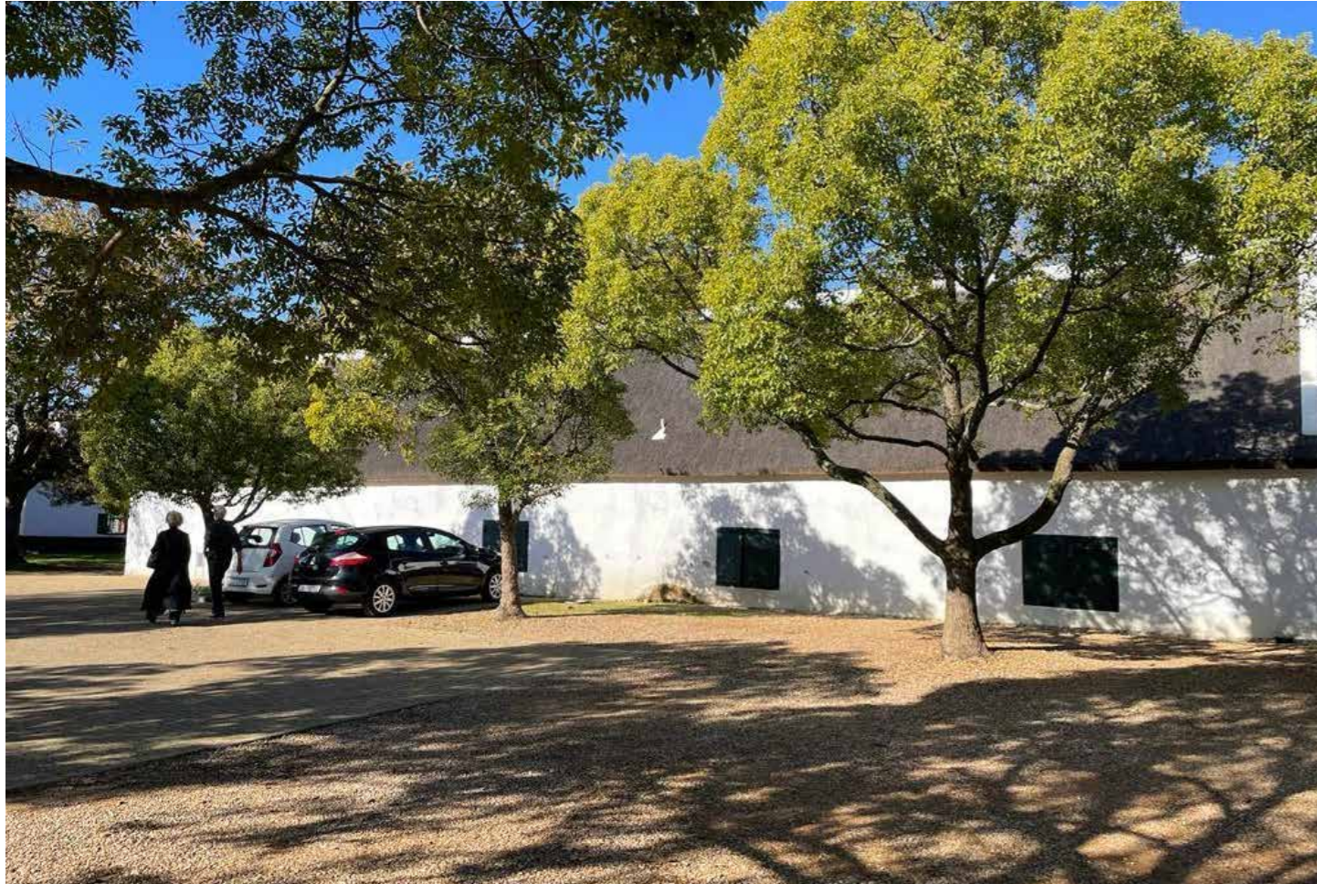
Figure 16. Rear facade of building, view to north east (Boschendal, 2022)
