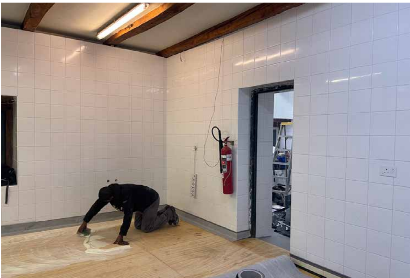
Figure 12. Kitchen and Scullery (RSA, 2022)
