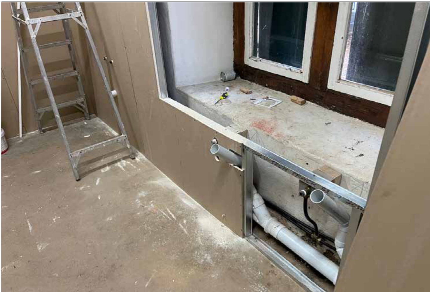
Figure 11. Kitchen and Scullery (RSA, 2022)
