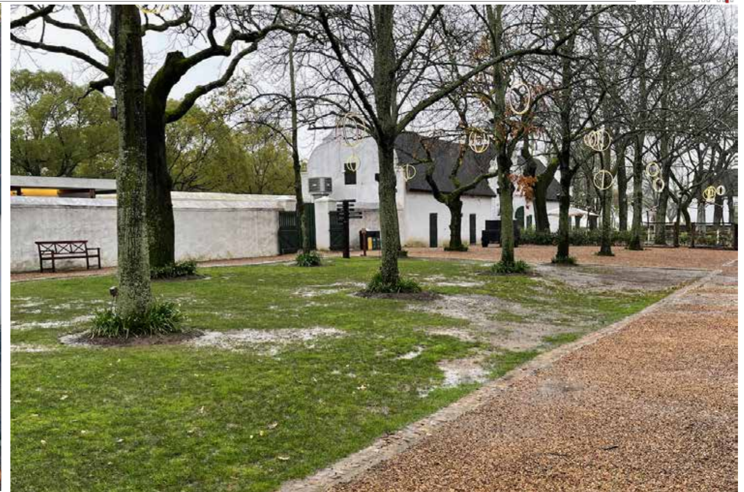
Figure 3. Exterior of building in context, view to north west (RSA, 2020)
