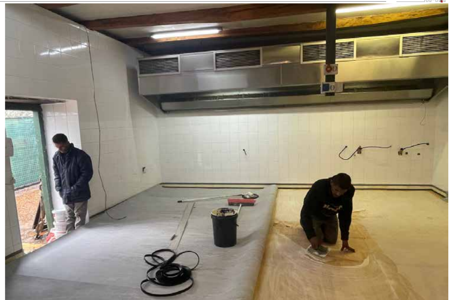
Figure 13. Kitchen and Scullery (RSA, 2022)
