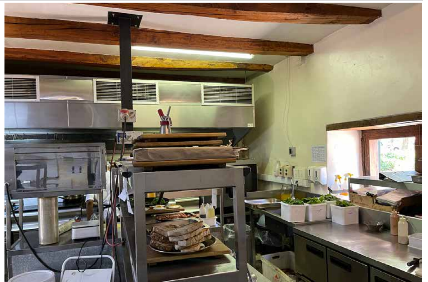
Figure 9. Kitchen and Scullery (RSA, 2022)
