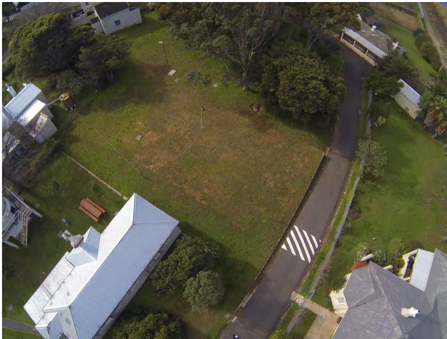
PHOTO 7: Aerial view of the site with surrounding structures
