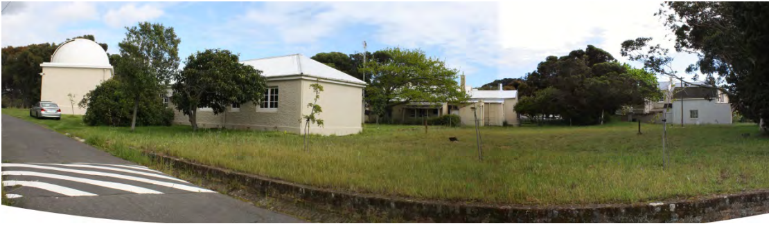
PHOTO 4: Levelled site of the proposed SAEON office with surrounding structures (left to right): Astrographic Telescope, RNA Building, Jacaranda House (rear) and Sidereal Clock House
