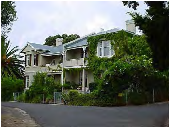
PHOTO 14: Houses 3 and 4 (13 and 14)
