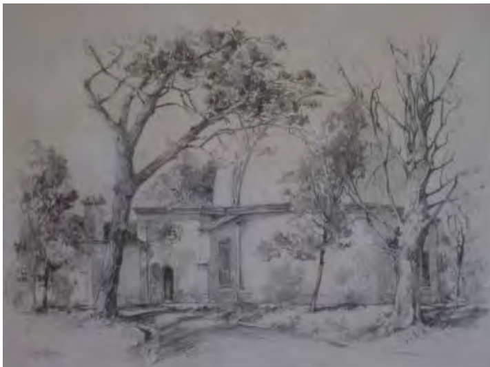
FIGURE 8: Lithograph of McClean dome, a Herbert Baker building, by artist and astronomer Charles E. Peers (c 1930) (SAAO Archives)
