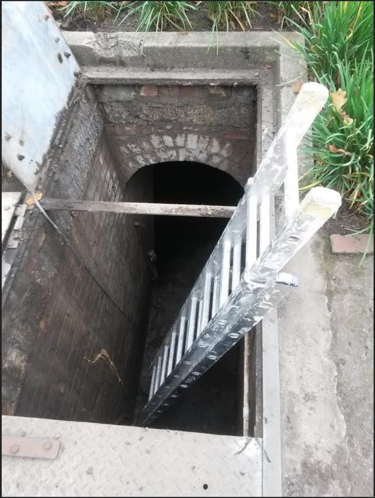
Figure 5 The brick drain.
