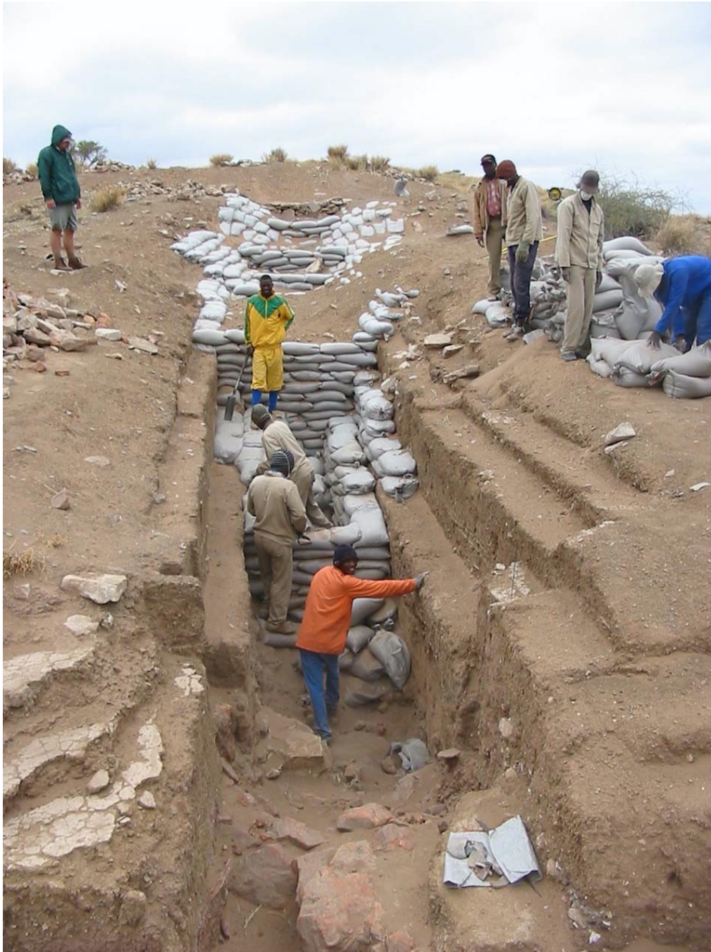
Figure 11: The sandbags being used to stabilise excavated walls.
