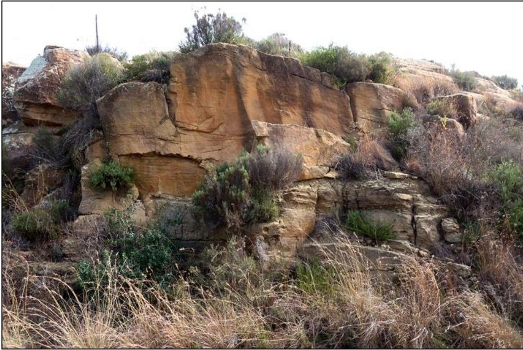
Figure 38: Deeply incised erosional base of a thick-bedded Molteno Formation channel sandstone package overlying khaki, thin- to medium-bedded mudrocks, road cutting on Farm Weltevrede 16/222 (SEF 4).
