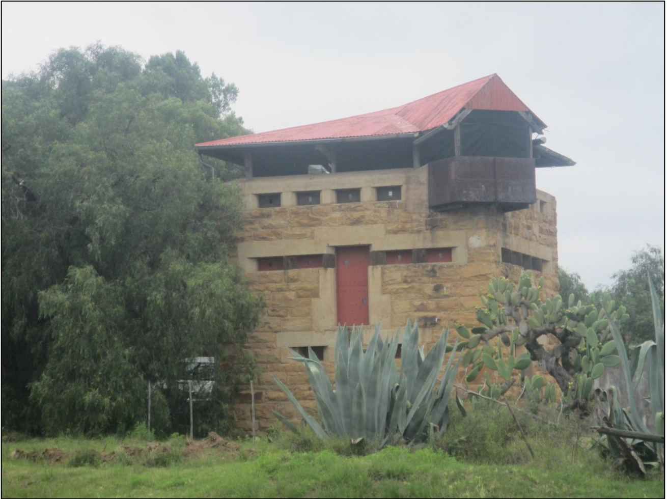
Figure 82: The southern blockhouse at waypoint 1659 which has been renovated for use as tourist accommodation.
