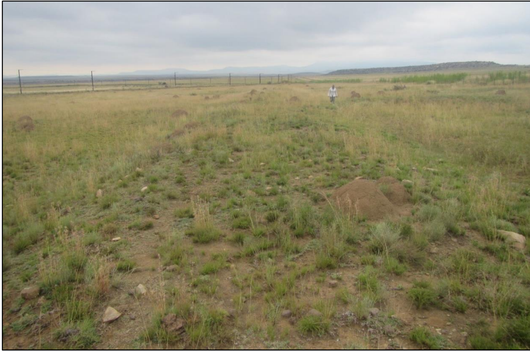
Figure 87: View along the historic and now abandoned railway berm at waypoint 1657. The new railway alignment is visible in the background.
