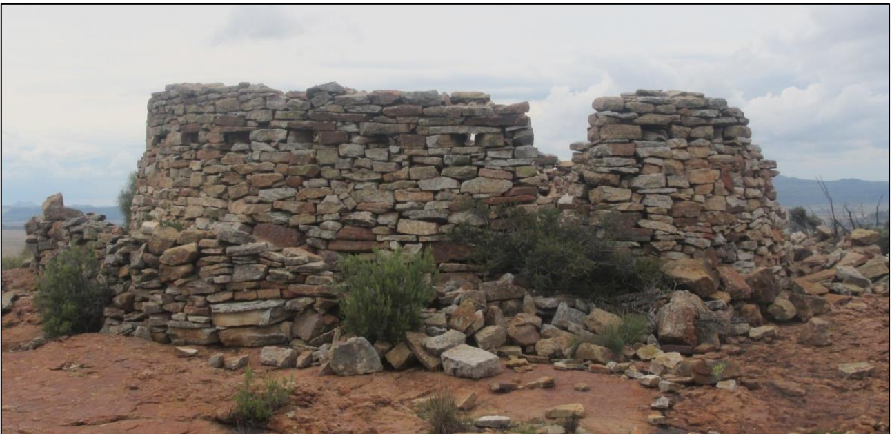
Figure 39: A proper fort built with drystone walling and including loopholes at waypoint 1683.
