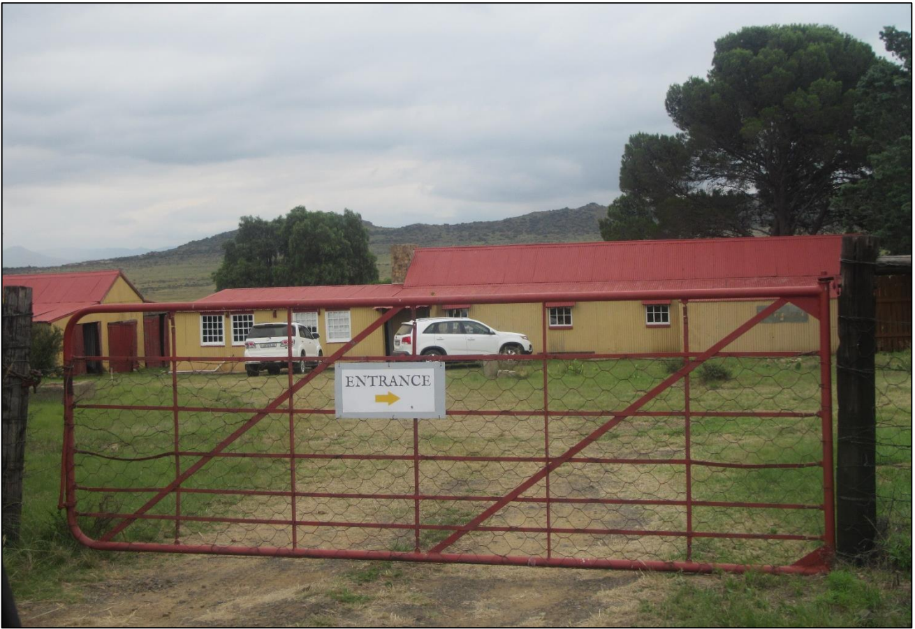
Figure 83: Structures at waypoint 1659 at the Stormberg Junction.
