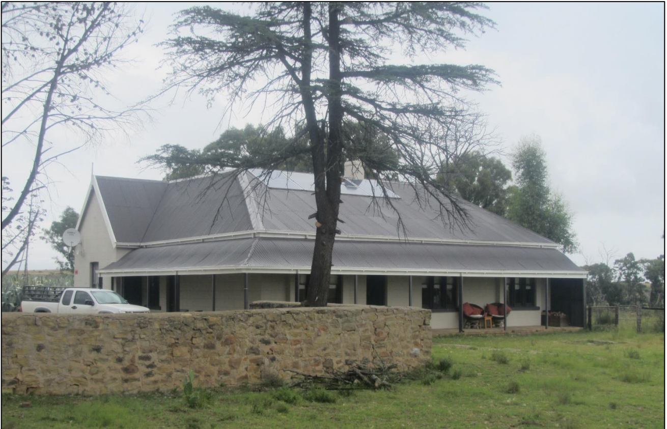
Figure 74: A restored and renovated Victorian farmhouse at waypoint 1690.
