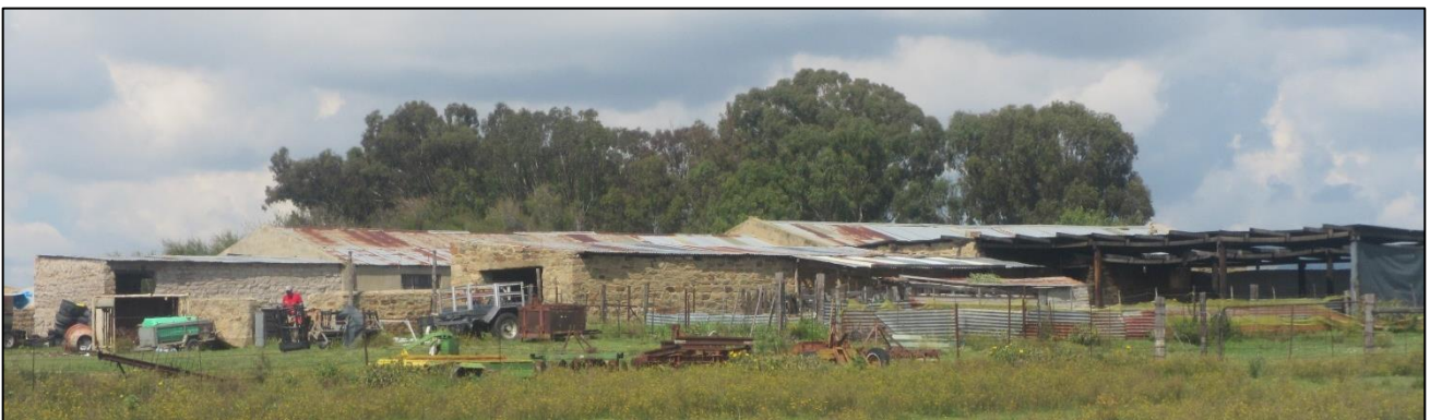
Figure 75: Stone-walled farm sheds with corrugated iron roofs at waypoint 1799.
