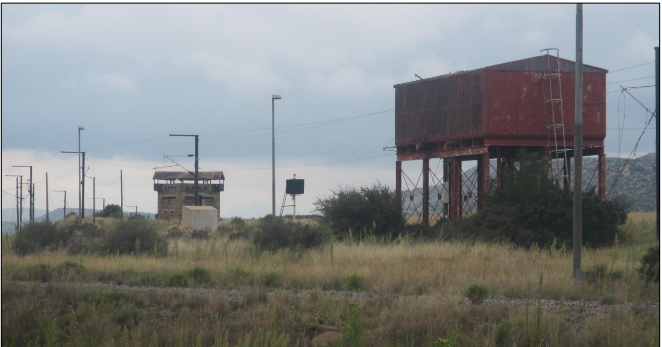
Figure 81: Infrastructure at the Stormberg Junction to the northeast of waypoint 1660. It includes a British Blockhouse (background; this is the northern blockhouse) and a raised metal structure that was probably a water tank (foreground).
