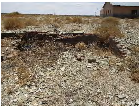
L-shaped foundations near the Visserskloof farmhouse (HST-002)
