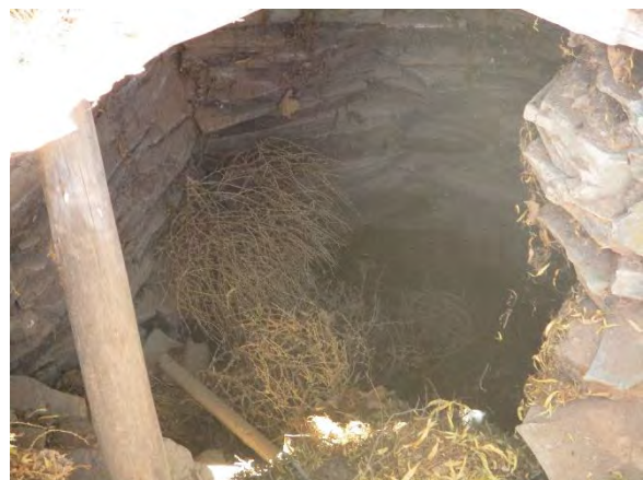
Historical well lined with slate and supported by timbers at HST-002
