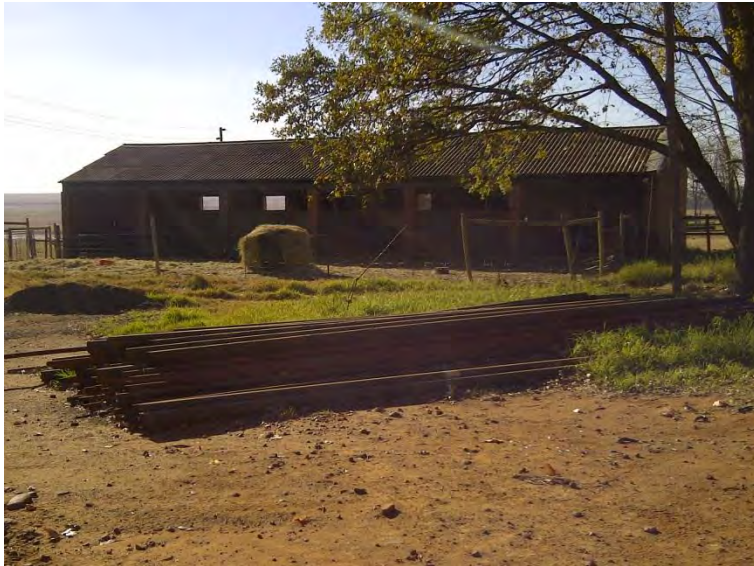
Figure 4-10: A work shed at Site S.34-003 that is part of the werf on Langsloot 99 IS.
