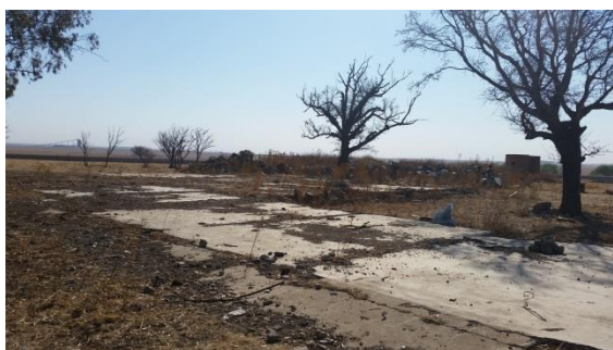
Figure 4-12: Foundations of structures at Wf001
