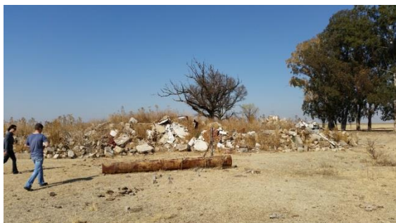
Figure 4-13: Rubble remains of built structure at Wf001
