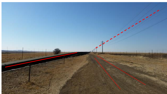
Figure 4-18: Existing servitude for the proposed pipeline. Note visible conveyor, road and transmission line within fence boundary
