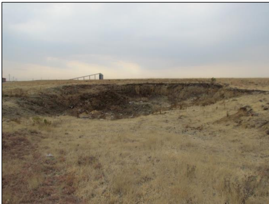
Figure 4-16: Borrow pit from where material was sourced to stabilize the pylons
