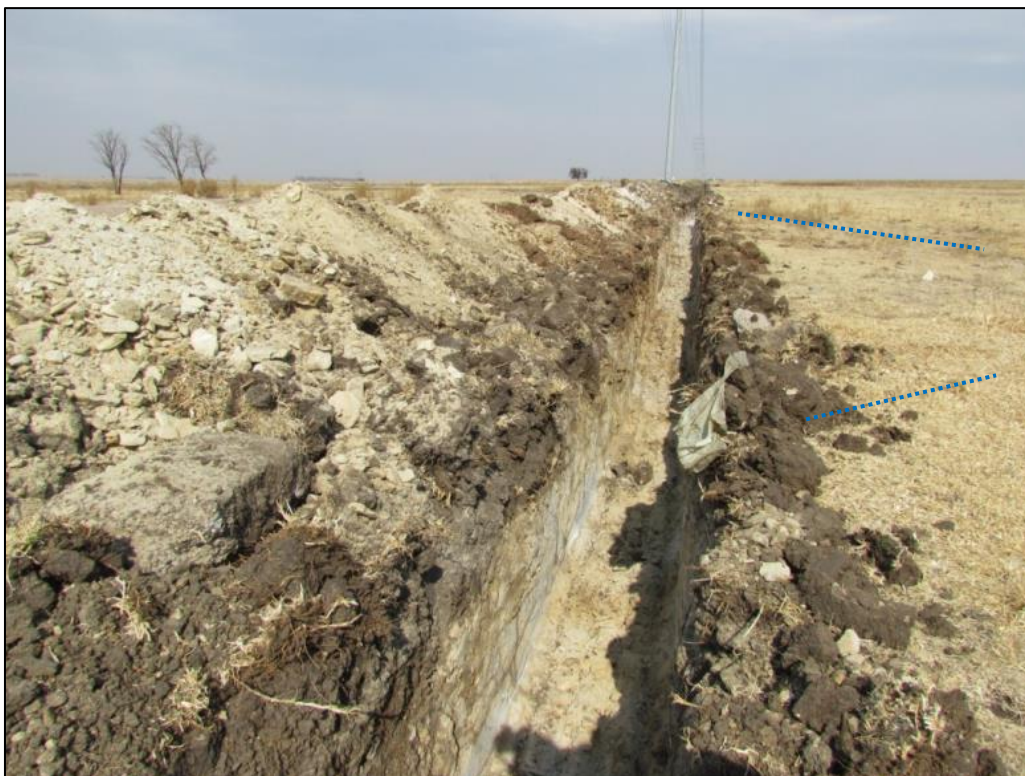
Figure 4-12: Completed excavation through the second foundation (blue)
