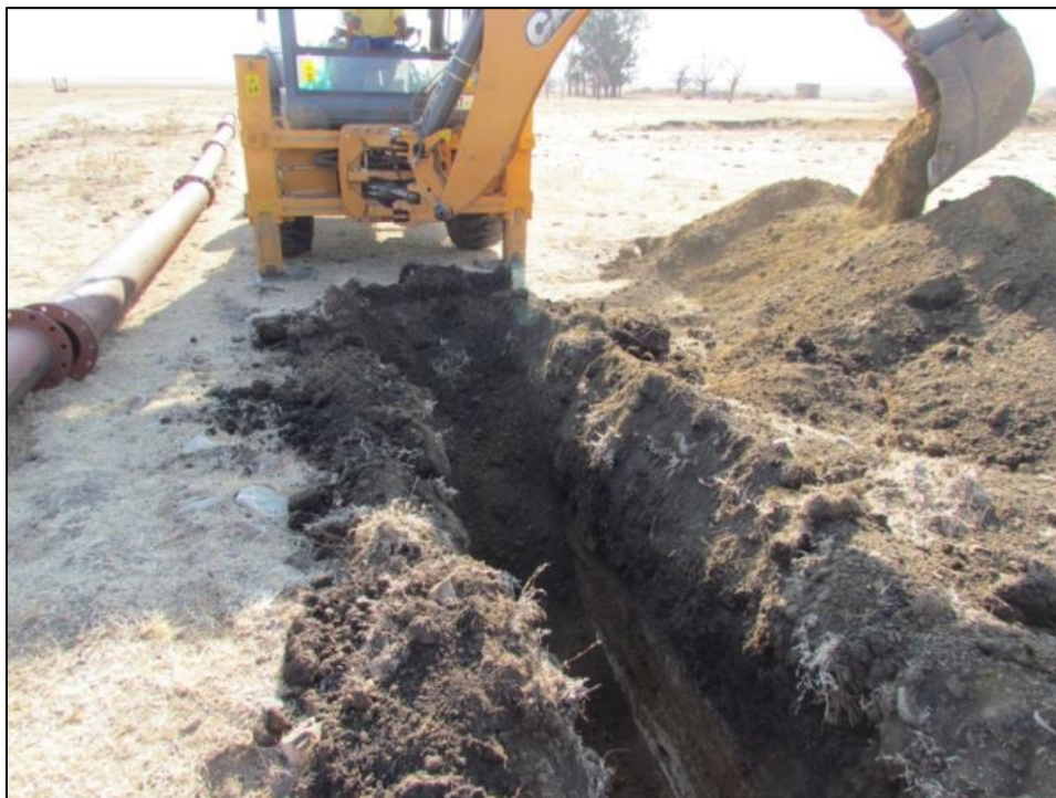
Figure 4-5: Completed excavation process through first stone foundation
