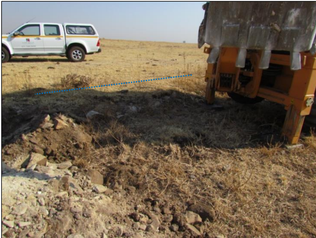
Figure 4-11: Starting excavating through the second foundation (blue)
