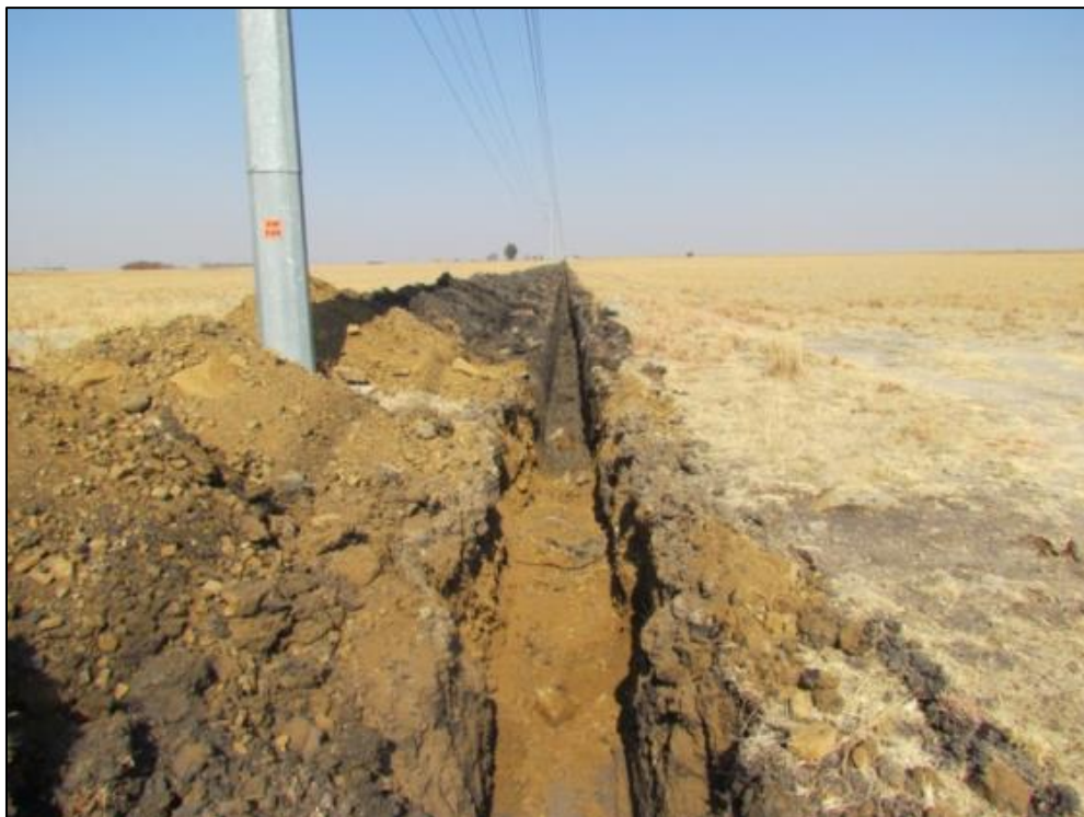
Figure 4-15: Orange brown soil around the base of the power line pylons
