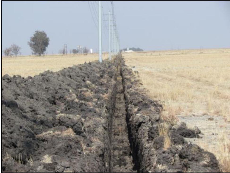
Figure 4-14: Dark clay soil excavated during week 3
