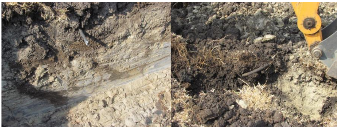
Figure 4-9: Electrical and plastic pipes uncovered by the excavator
