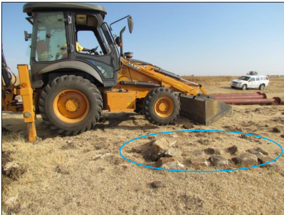
Figure 4-4: Excavation process through first stone foundation (blue)
