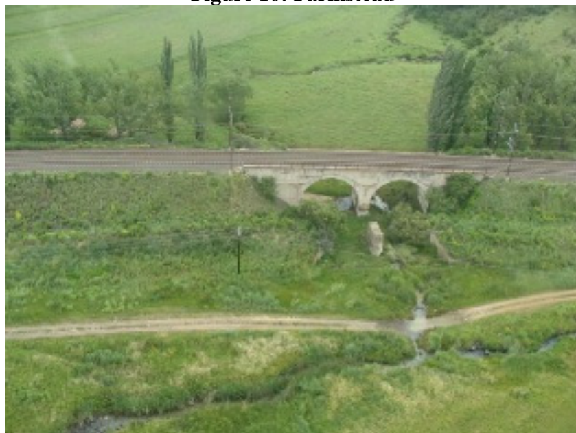
Figure 17: Old Rail Bridge
