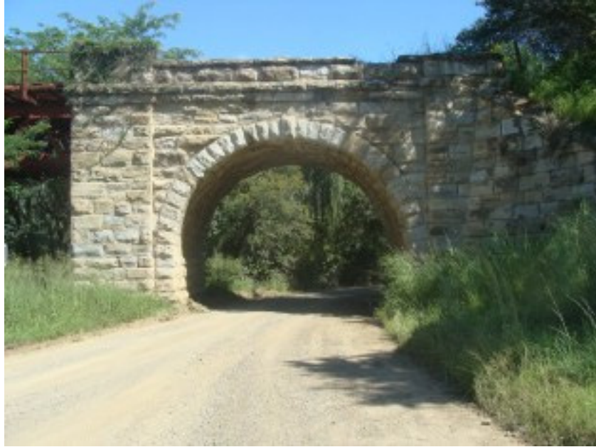
Figure 20: Historical railway bridge near Estcourt
