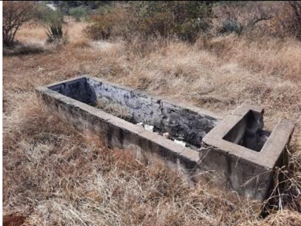
Figure 17 - Cement water trough at Site 1-3
