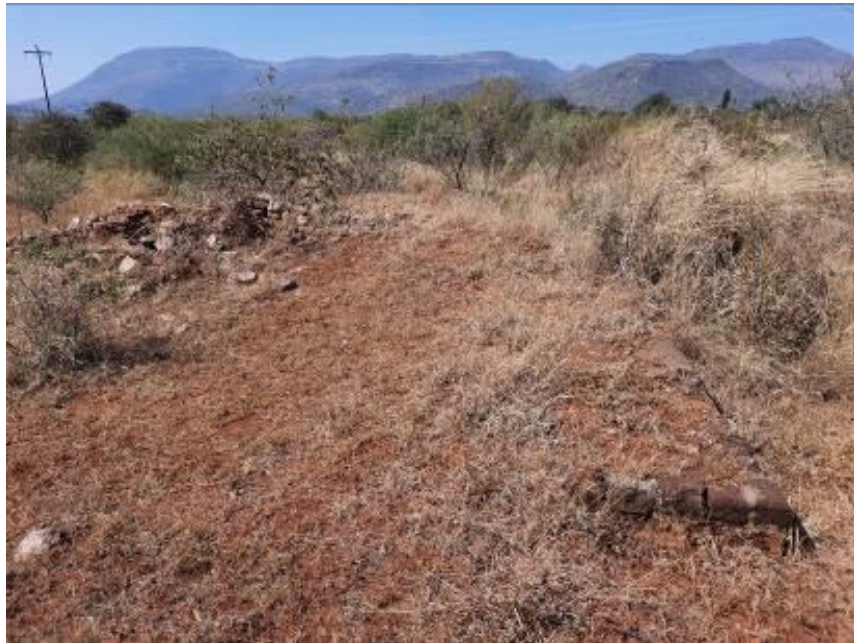
Figure 18 – A series of broken-down structure and foundations.
