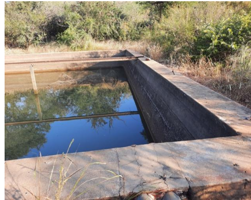
Figure 36 – Large cement water reservoir at Site 2-5
