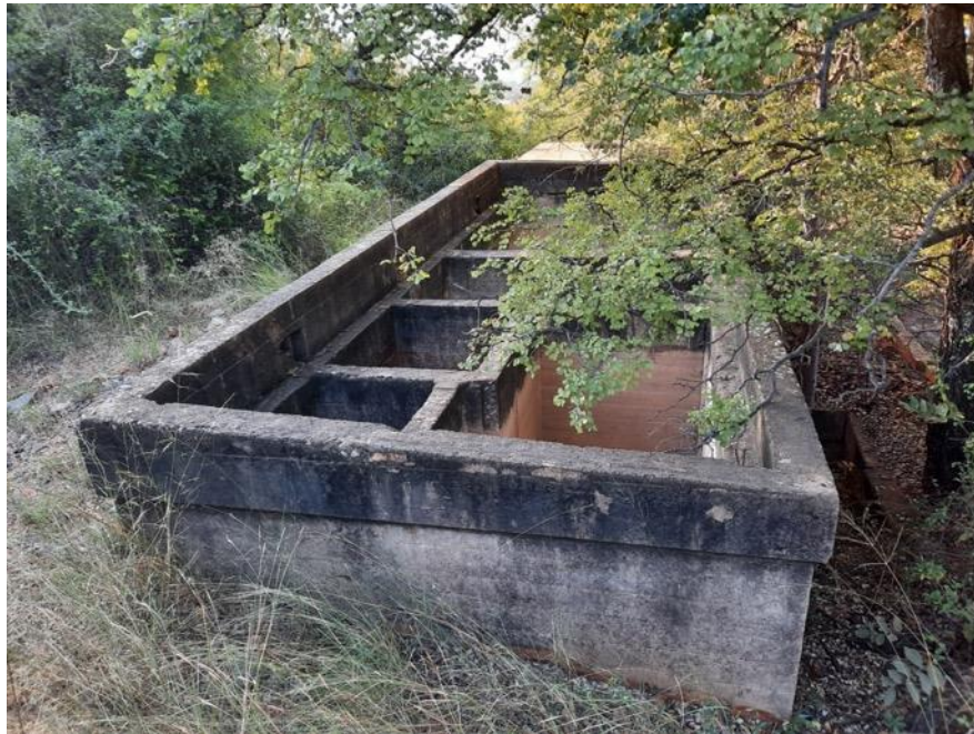
Figure 35 – Cement structure at Site 2-5
