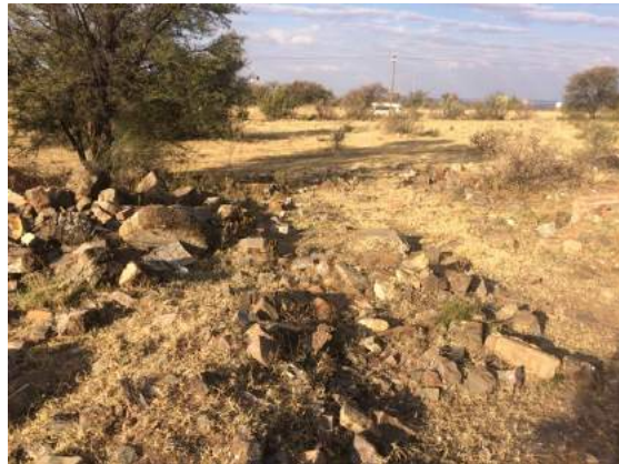
Figure 31 - Brick, stone, concrete and cement remains of the multi-roomed structure at site 020.
