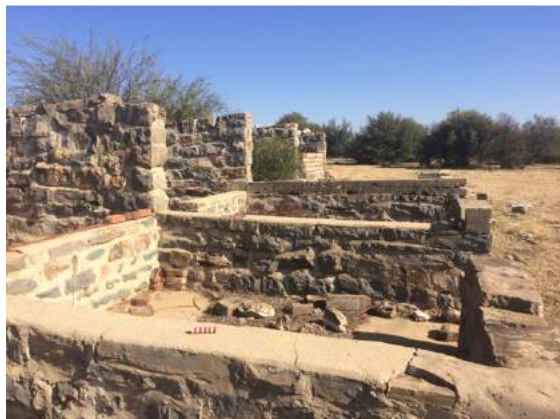
Figure 40 - Large multi-roomed stonewalled structure at site 026, likely used for keeping livestock. Note north and south sections of the building, with drinking/food troughs in the low-walled north sections. Also note a mix of construction materials (stone, cement and brick).
