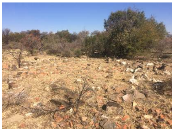
Figure 42 - Poorly preserved structure at site 028, showing presence of bricks, stone and cement.
