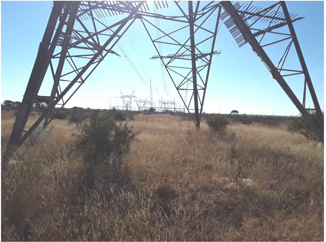
Figure 11: Mookodi Substation about 4.5km north of the project site. Note the characteristic flat-lying terrain with the vegetation cover of grassy thornveld. No outcrops are present
