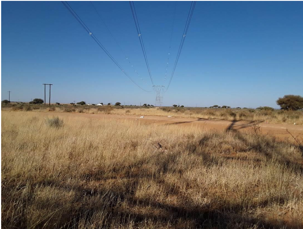
Figure 12: Flat topography of the proposed power line corridor near Vryburg
