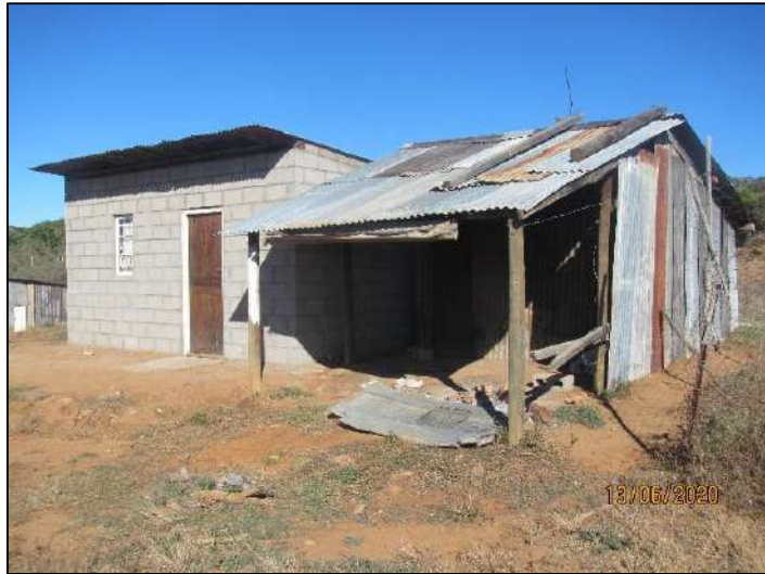
Figure 32 - View of the labourer house
