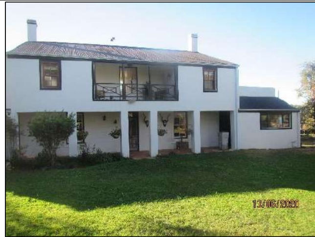
Figure 21 - Southern facade of the house
