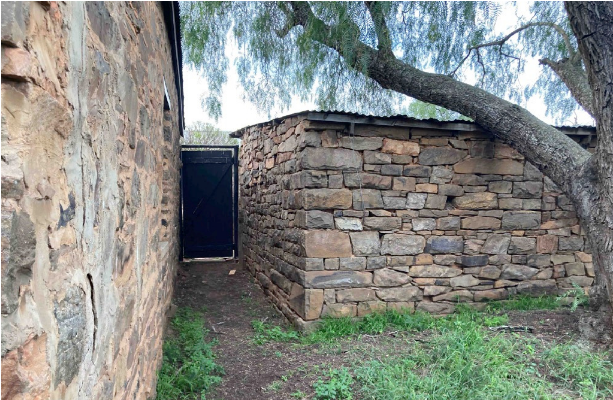
Figure 16: Outbuildings on Hounslow Farm in the north of the project site, showing use of local stone for construction.
