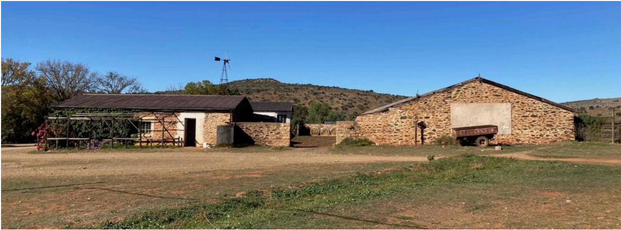
Figure 33: Historic stone structures on Table Hill Farmstead.
