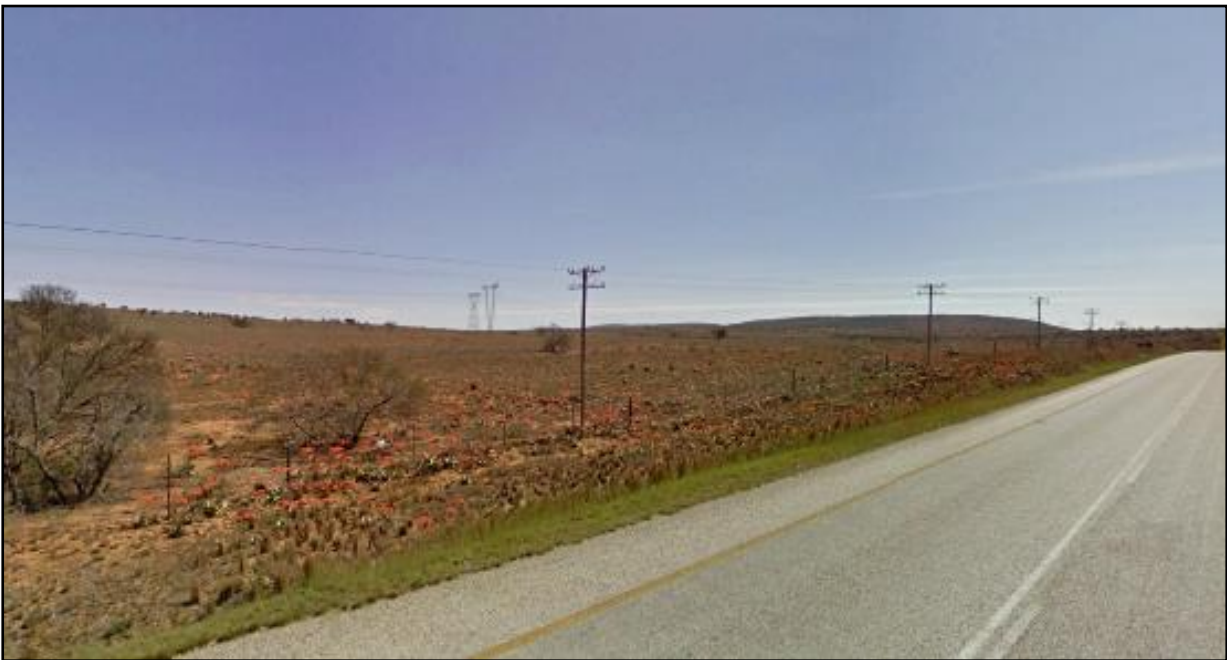
Figure 45 - View of the development site from the N10 national road (du Plessis, 2021).
