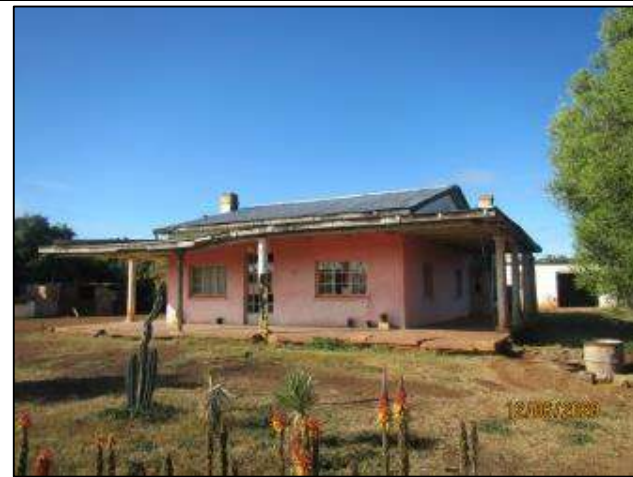
Figure 28 - View of the northern façade.
