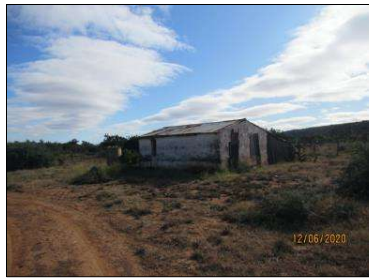
Figure 61 - View of the south-eastern corner of the shed at EWF1-09.
