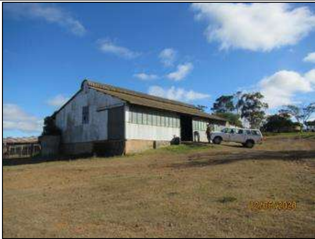
Figure 41 - View of the bigger shed.
