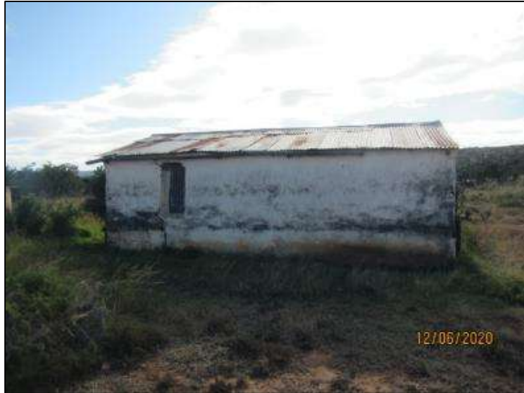
Figure 60 - View of the southern façade.
