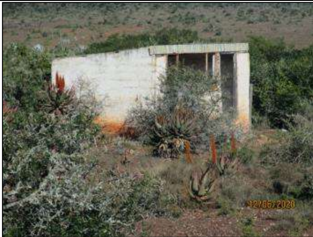
Figure 29 - View of the outbuilding.
