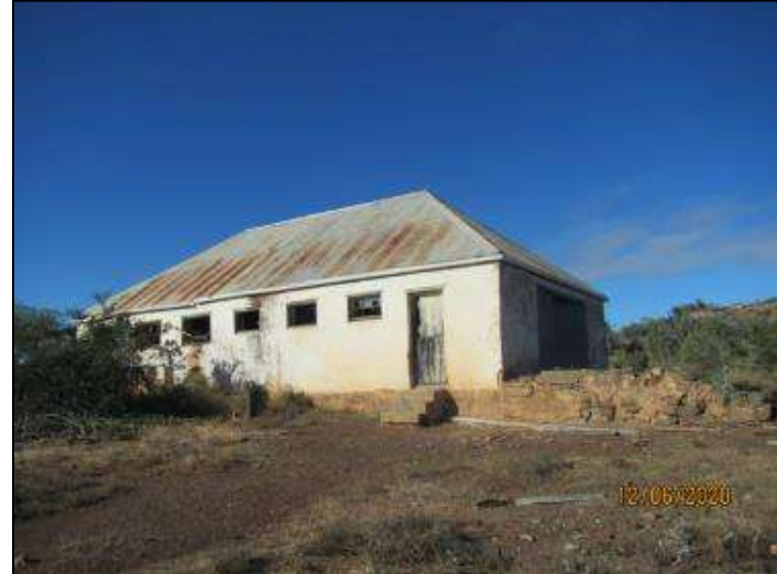
Figure 25 - View of the northern façade.
