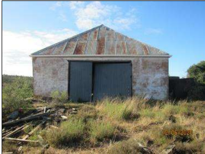
Figure 24 - View of the western façade.
