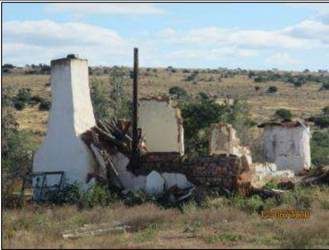
Figure 49 - Demolished labourer house.
