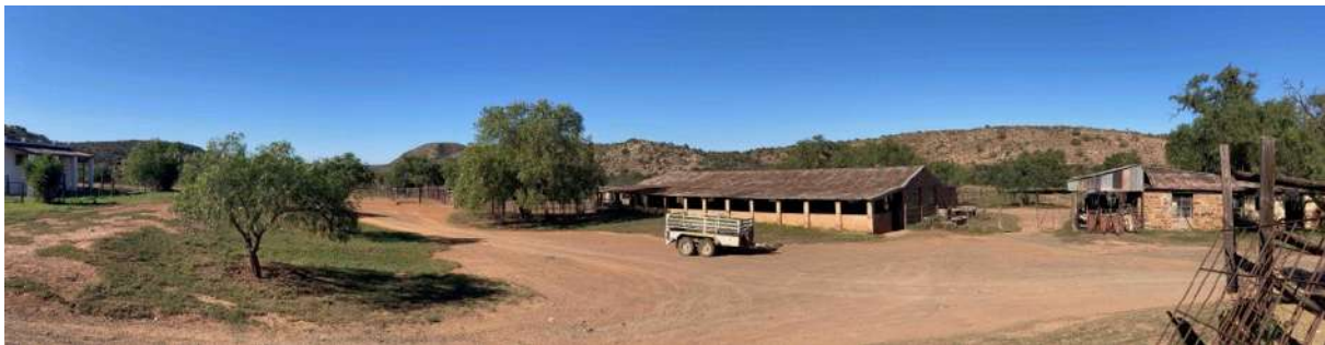
Figure 37: View of steep ridge to southeast from Hounslow farmstead with agricultural stone structures in the foreground. Two proposed turbines from the Wind Garden WEF would be visible above the ridge from this viewpoint.
