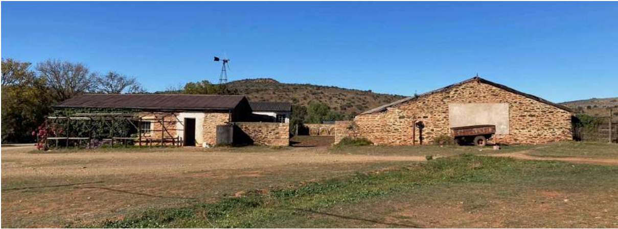
Figure 34: Historic stone structures on Table Hill Farmstead.
