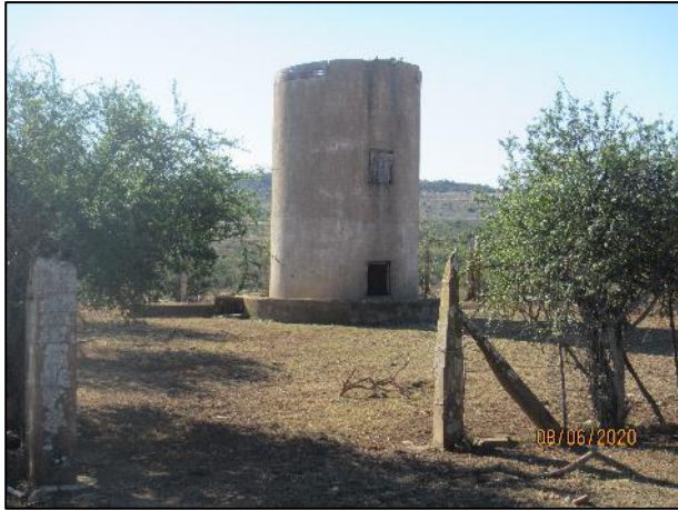
Figure 53 - Second storage silo identified (WWF1-08e).
