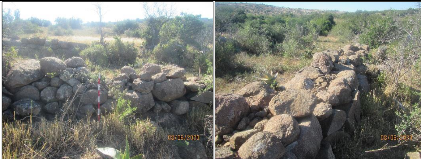
Figure 34 - The collapsed wall of the stone cattle kraal at site WWF1-03. The scale is in 10cm increments.
