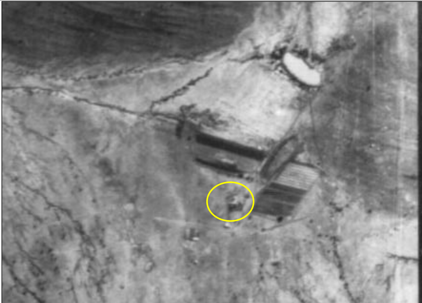
Figure 55 - Section of the 1949 photograph (230_005_00446) showing the main farmhouse (WWF1-08a) (yellow circle locate at WWF1-08).
