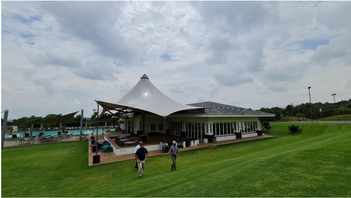
Figure 6 Existing pool pavilion facility
