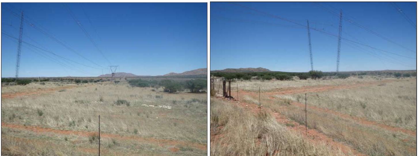
Figure 4.7: Contextual Images - existing electrical infrastructure
