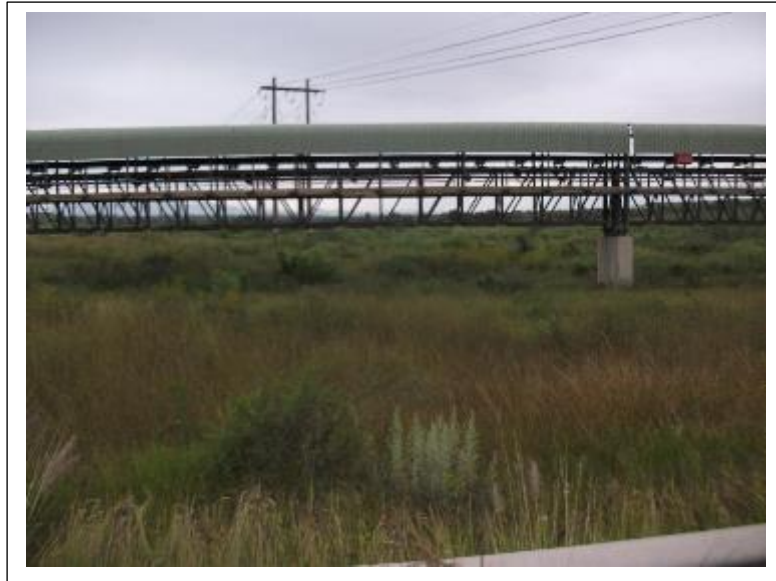
Figure 6- The northern edge of the project area borders on the Klipfontein River and some of Eskom's power lines (above).
