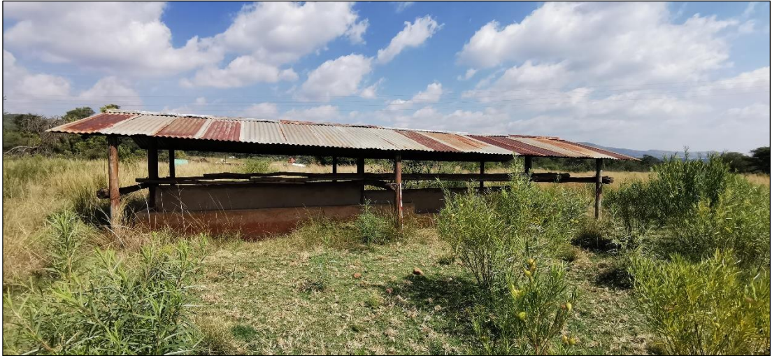
Figure 8 - Small structure that serves as a feeding trough located in the Development Footprint.
