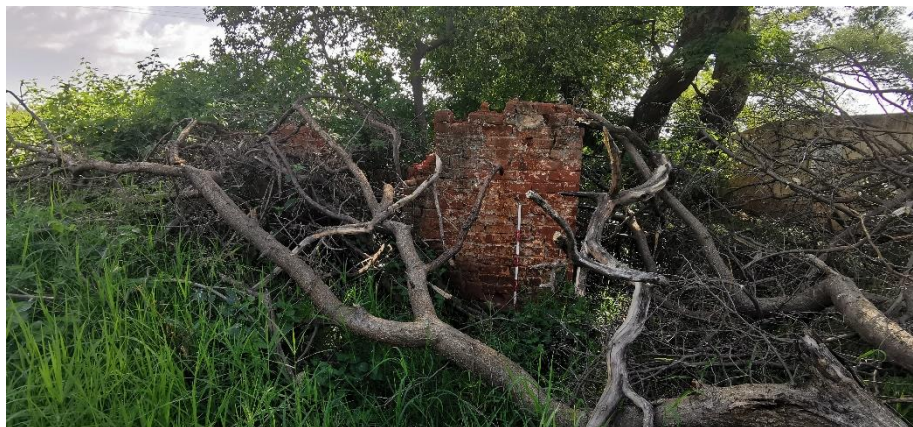
Figure 53 – General view of the small brick structure located at site BFP-08. The scale is in 10cm increments.
