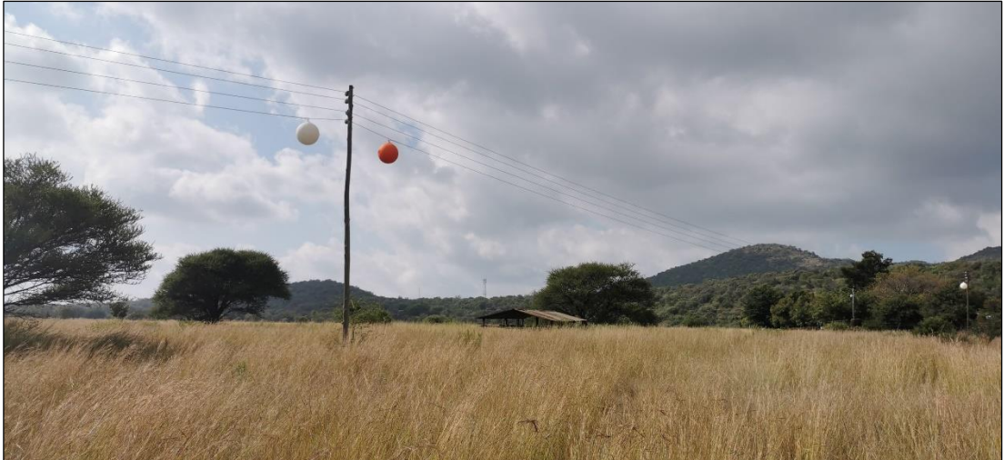
Figure 14 - Powerlines located in the proposed Development Footprint.
