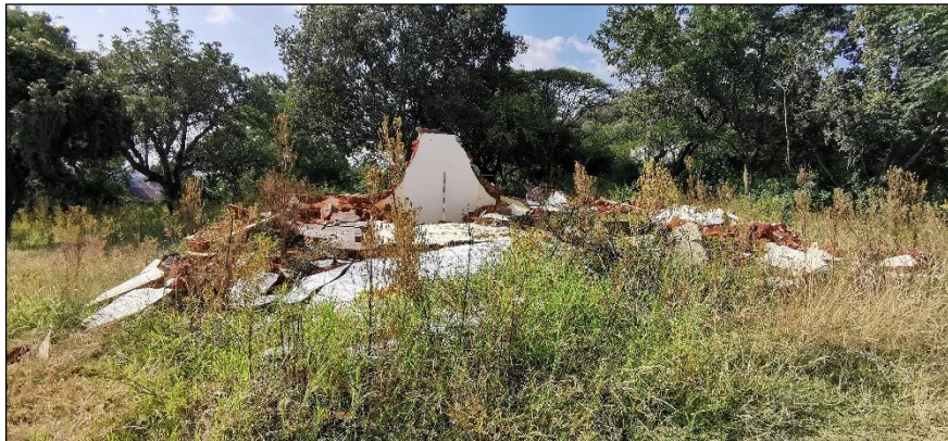
Figure 53 – General view of the broken-down structure located at site BFP-07. The scale is in 10cm increments.
