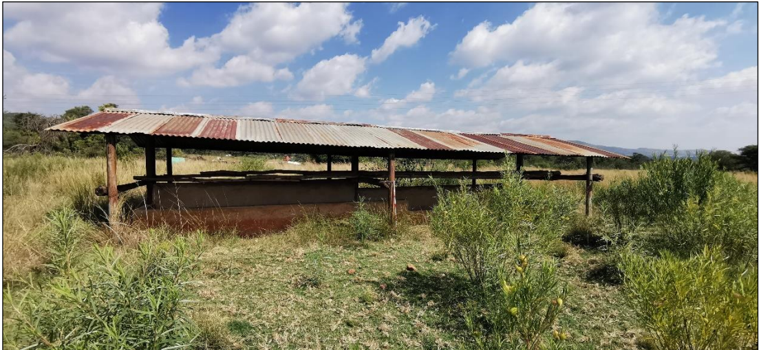
Figure 9 - Small structure that serves as a feeding trough located in the Development Footprint.
