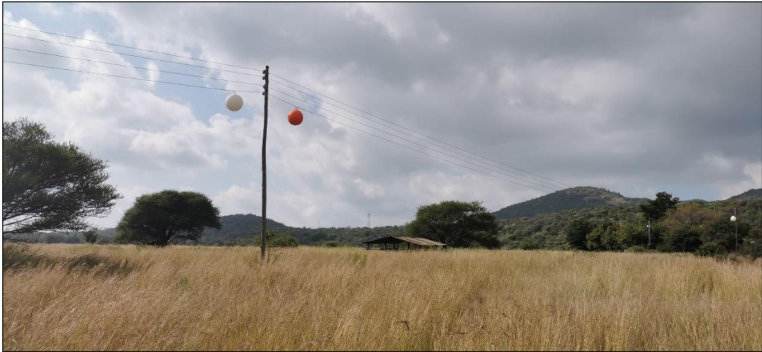
Figure 15 - Powerlines located in the proposed Development Footprint.
