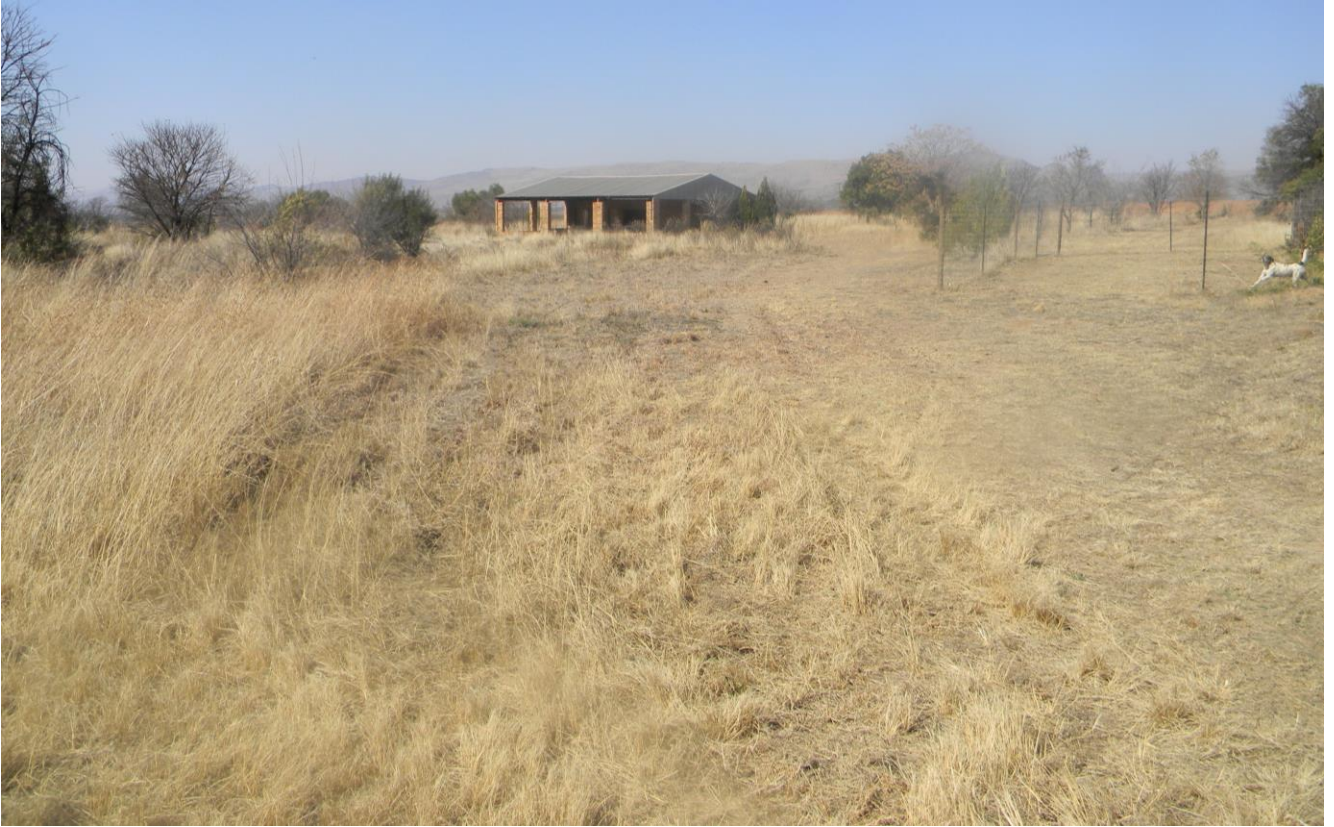
Plate 5: Photo 5: View of abandoned farm structures within the proposed development site (Photograph © by Author 2017).
