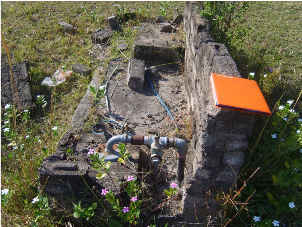
Figure 6: An old water supply in the development area.
