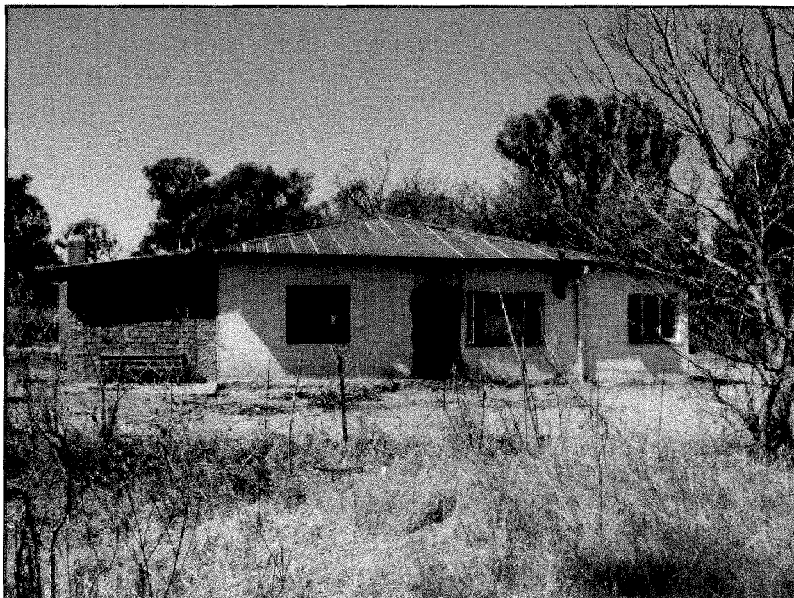
Figure 16 - View of farmhouse
