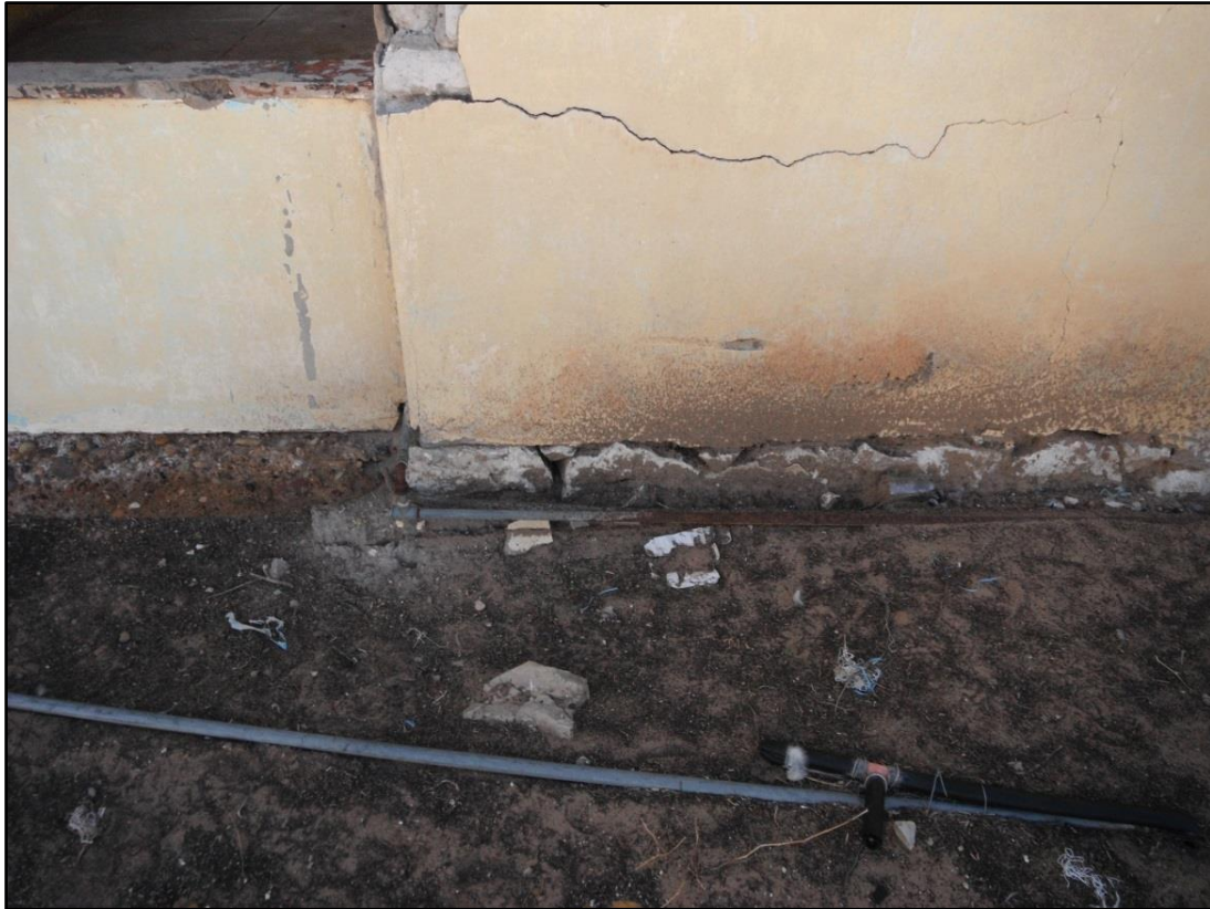
Figure 42 – Foundation constructed from locally sourced calcrete (WES1)
