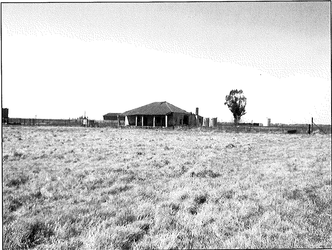
Figure 6. Sandstone farmstead at WCB 003
