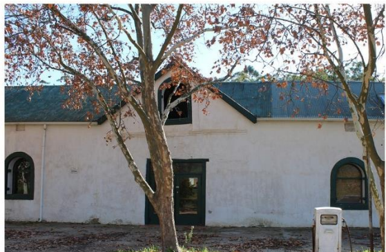
Viewpoint 5: Facade of historic Cellar building from adjacent access road
