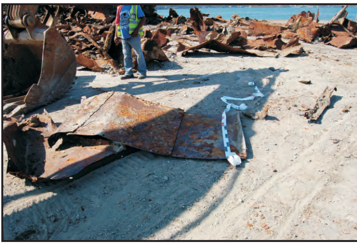
Figure 35: Joggled plating, this method of constructing the side plating did not require liners and was cheaper and lighter than previous methods (Pursey 1950: 82; Photo: Maitland)
