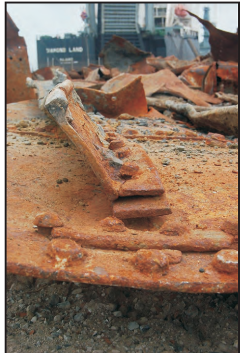
Figure 38: Close-up of bulb angle frames, they are stronger than frame-and-reverse, corrode less and require less riveting, they are also more suitable for joggled plates (Pursey 1950: 50; Photo: Maitland)
