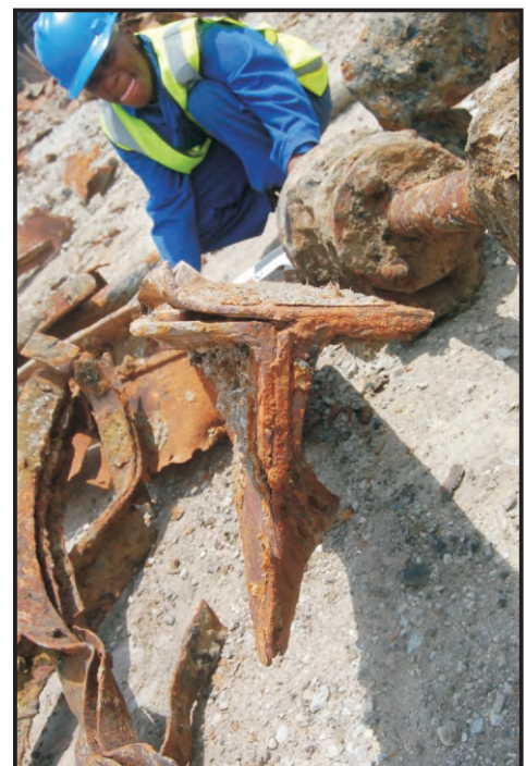
Figures 45 - 46: Double angle bar beam, possibly a deck support structure (Photo: Maitland)
