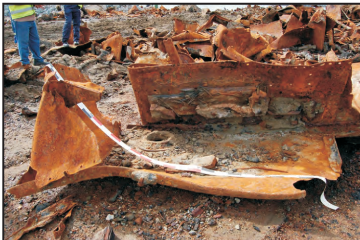
Figure 62: Bulwark with mooring pipe and deck plating with wooden base plate, the proximity of these items indicates bollards may have been attached to the base plate (Photo: Maitland)
