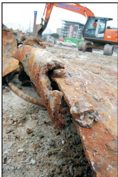
Figure 60: Close-up of the bulwark main rail (Photo: Maitland)
