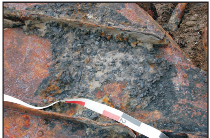
Figure 76: Plating with coal embedded in the corrosion, this section of plating is probably part of the coal bunkers, the Karin carried 85 tons of bunker coal (Appendix A: 3; Photo: Maitland)
