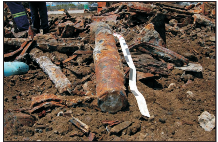
Figure 106: This 'mast' is constructed of solid steel therefore may actually be the eduction pipe from the condenser (Photo: Maitland)
