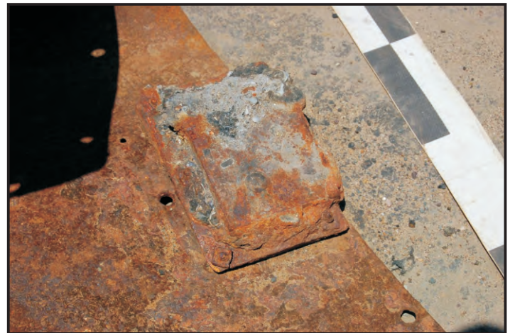
Figure 112: Close-up of lock (Photo: Maitland)
