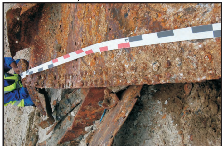
Figure 40: Hull plating with double riveting (Photo: Maitland)
