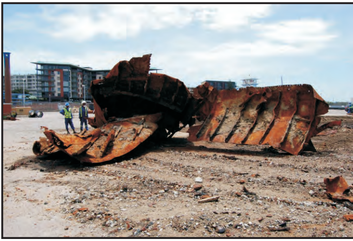
Figure 29: The largest section of hull plating removed intact, showing frames and stringers (Photo: Maitland)
