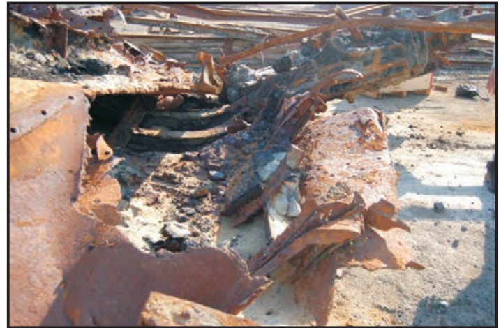
Figure 335: Turn of the bilge showing frames and riveted hull plating (Paasch 1890: Plate19; Photo: Maitland)
