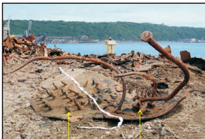
Fire box stays Boiler stays
