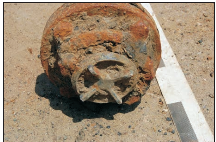
Figure 189: Cooling water inlet valve (Renda 2010; Photo: Maitland)
