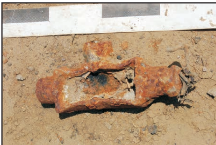
Figure 225: Electric junction box (Branch 1910:154; Photo: Maitland)
