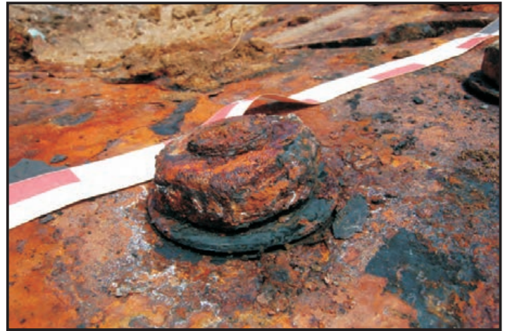
Figure 145: Close-up of a boiler stay nut and gasket on the outer surface of the boiler's back end plate (Photo: Maitland)
