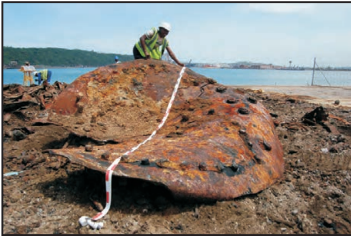
Figure 144: The outer surface of the boiler's back end plate (Photo: Maitland)
