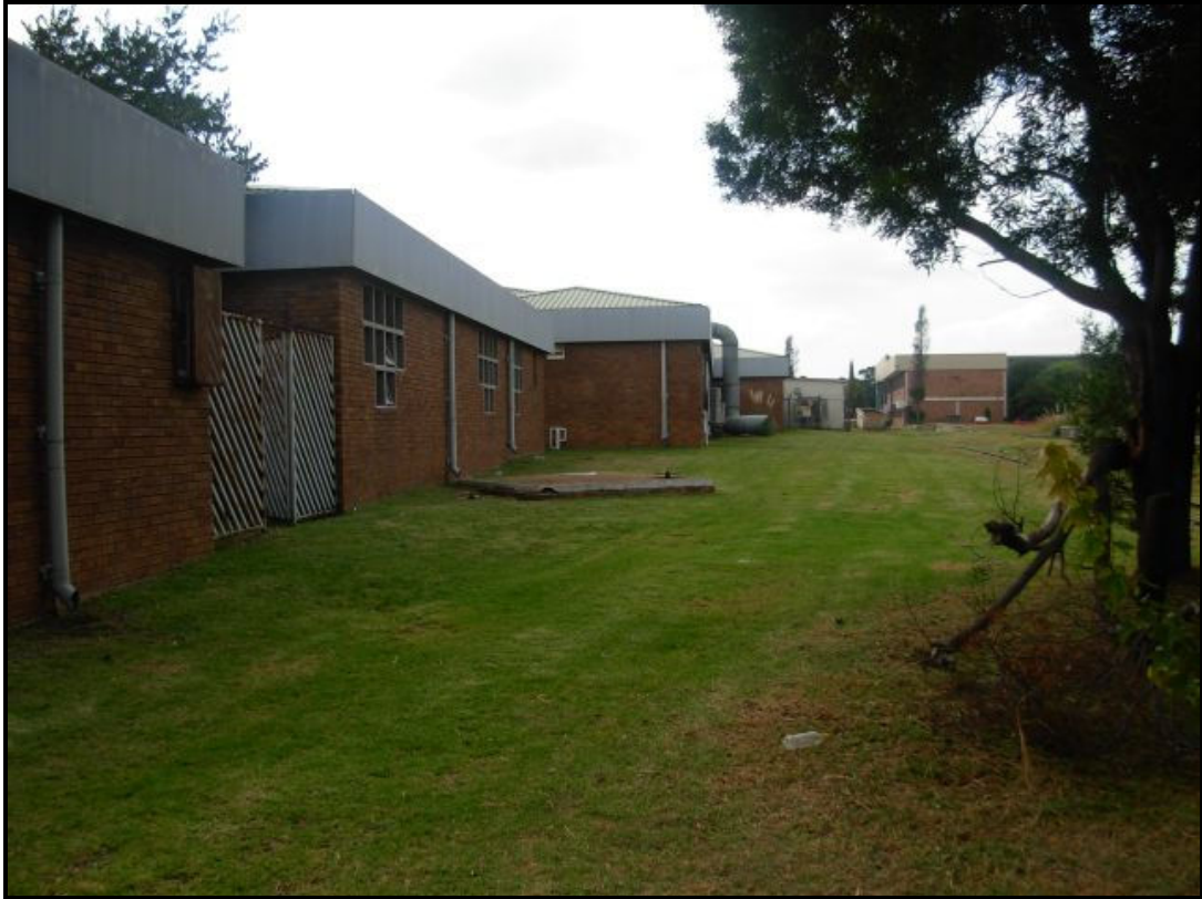
Figure 4 – Main valve inside Telkom yard in Factoria
