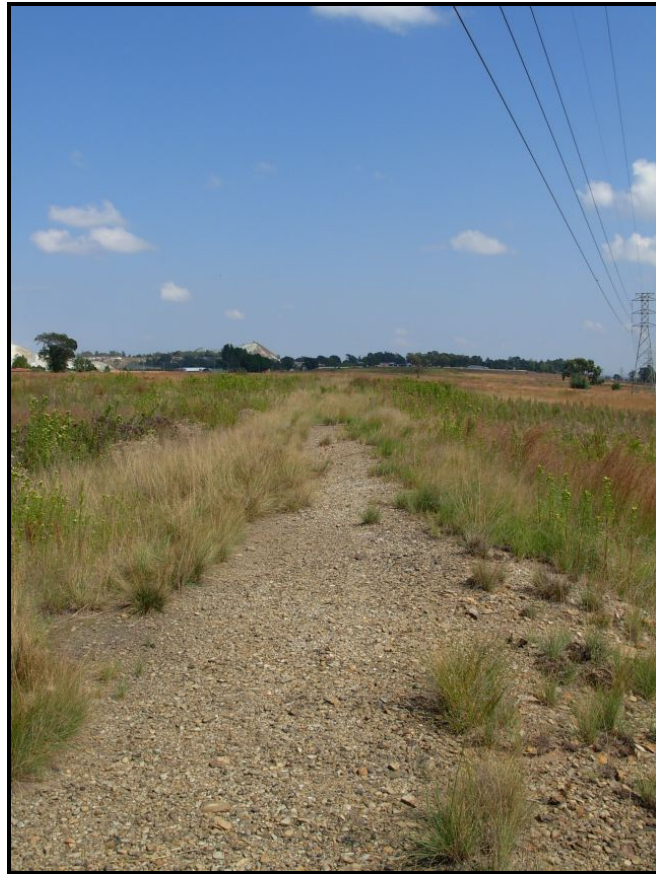
Figure 8 - Old rail foundation
