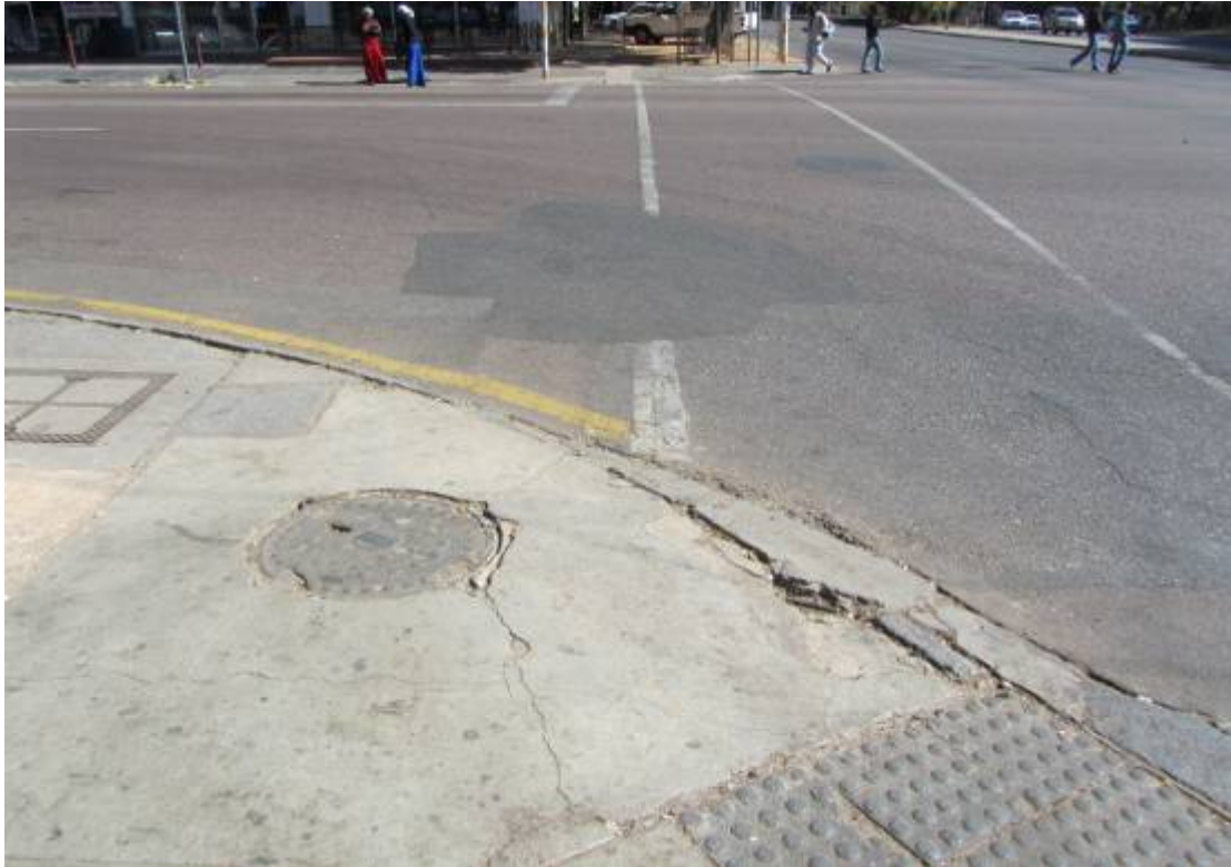
Figure 267. Variety of paving material. Note Granite curbing. (P 1064)
