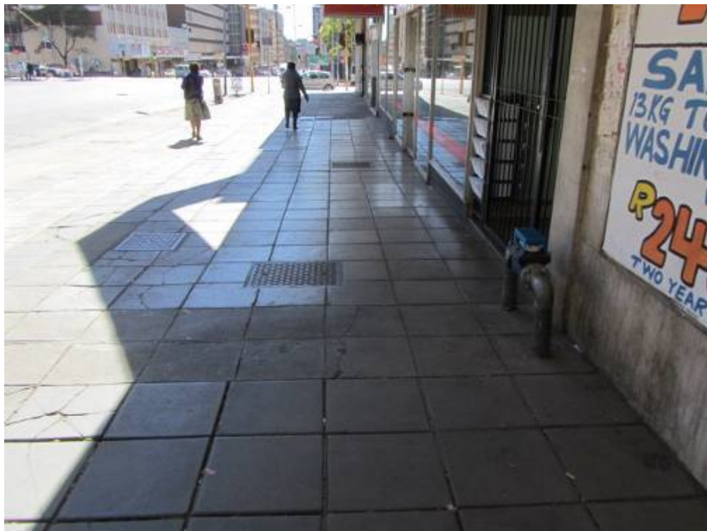
Figure 264. Variety of paving materials. Note that the cement blocks also date from different eras. (P 1061)
