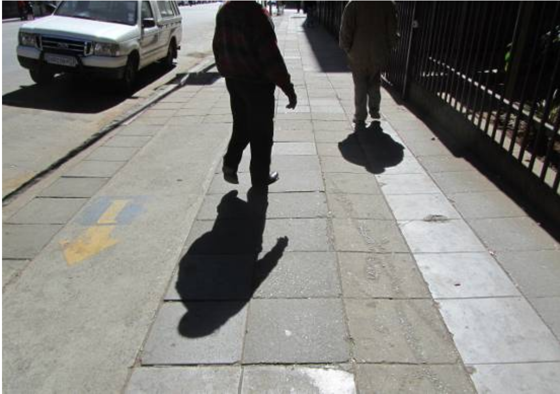
Figure 258. Variety of paving material. Note granite curbing. (P 1057)
