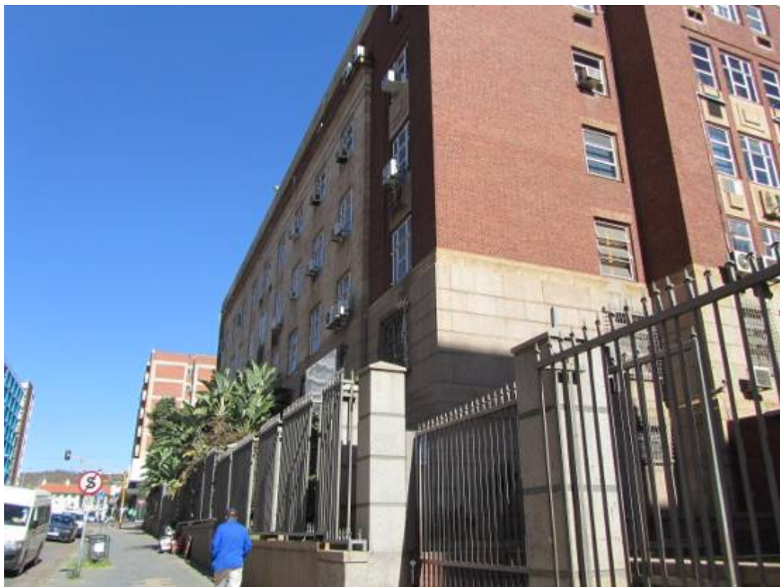
Figure 300. Protected building with wrought iron fence and stone pillars for definition of private domain. (P 1127)
