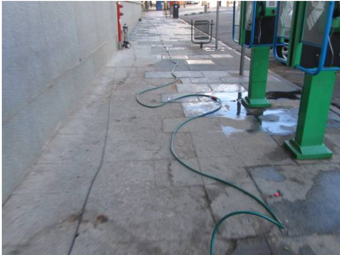
Figure 155. Cement paving adjacent to historical building. (P 958).
