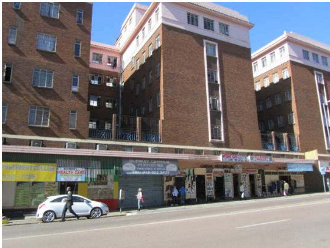
Figure 302. Protected building. (P 1130)
