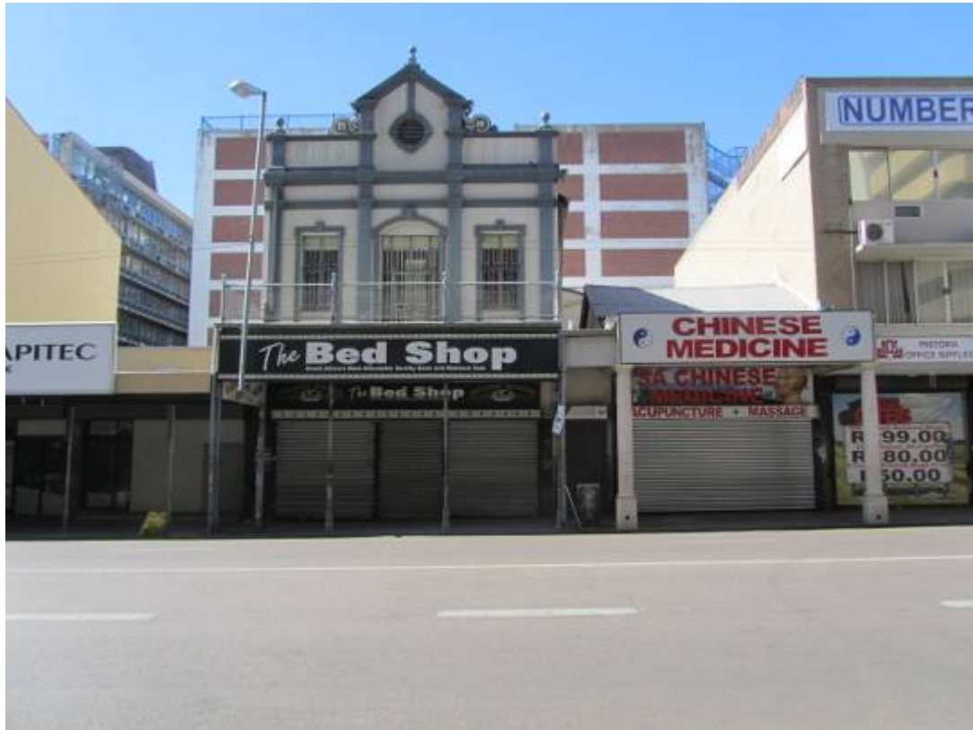
Figure 219. Protected buildings. (P 1018)
