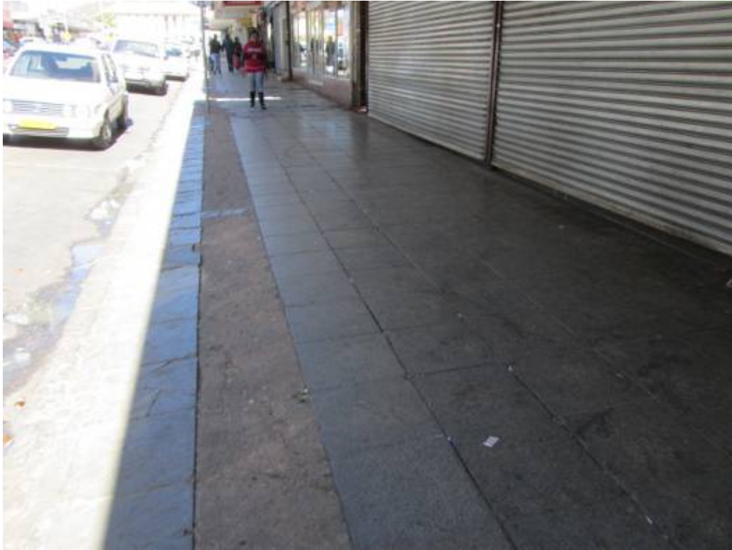
Figure 323. Cement block paving. (P 1096)
