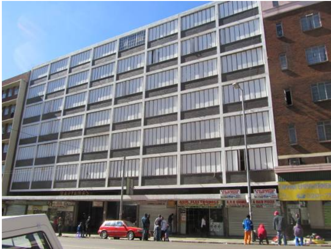
Figure 301. Provisionally protected building. (P 1129)
