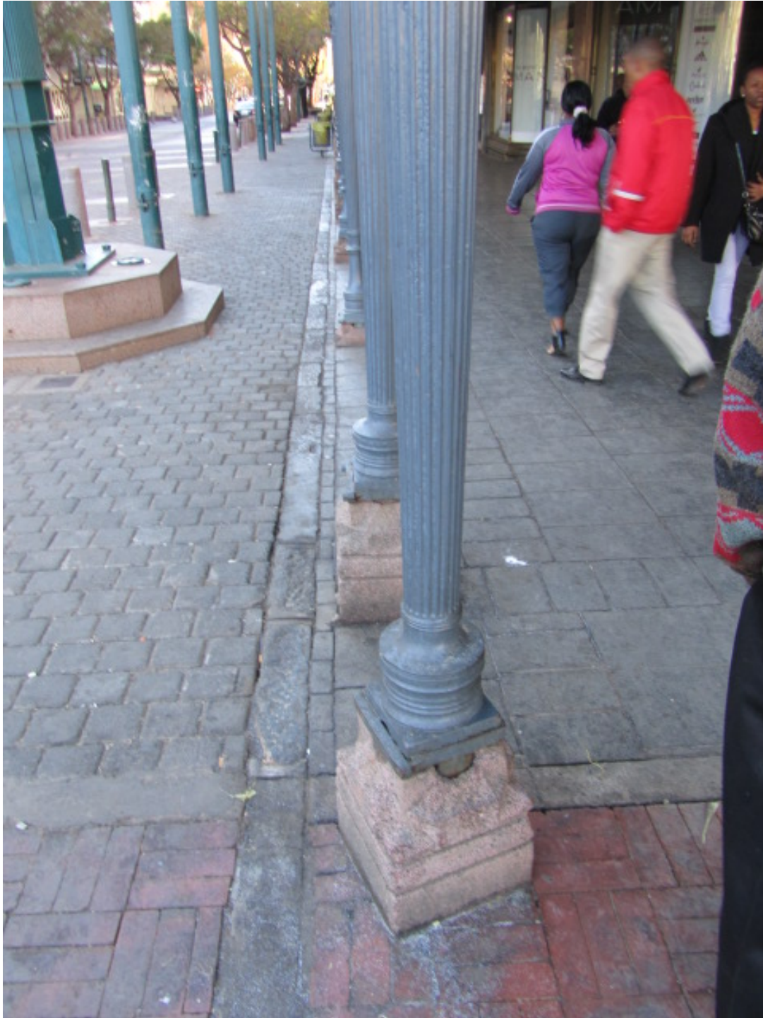
Figure 161. The refurbished paving in the Church Street Boulevard is excellent. Note the retention of the original granite curbing stones as the 'memory' from the past. (P 964).
