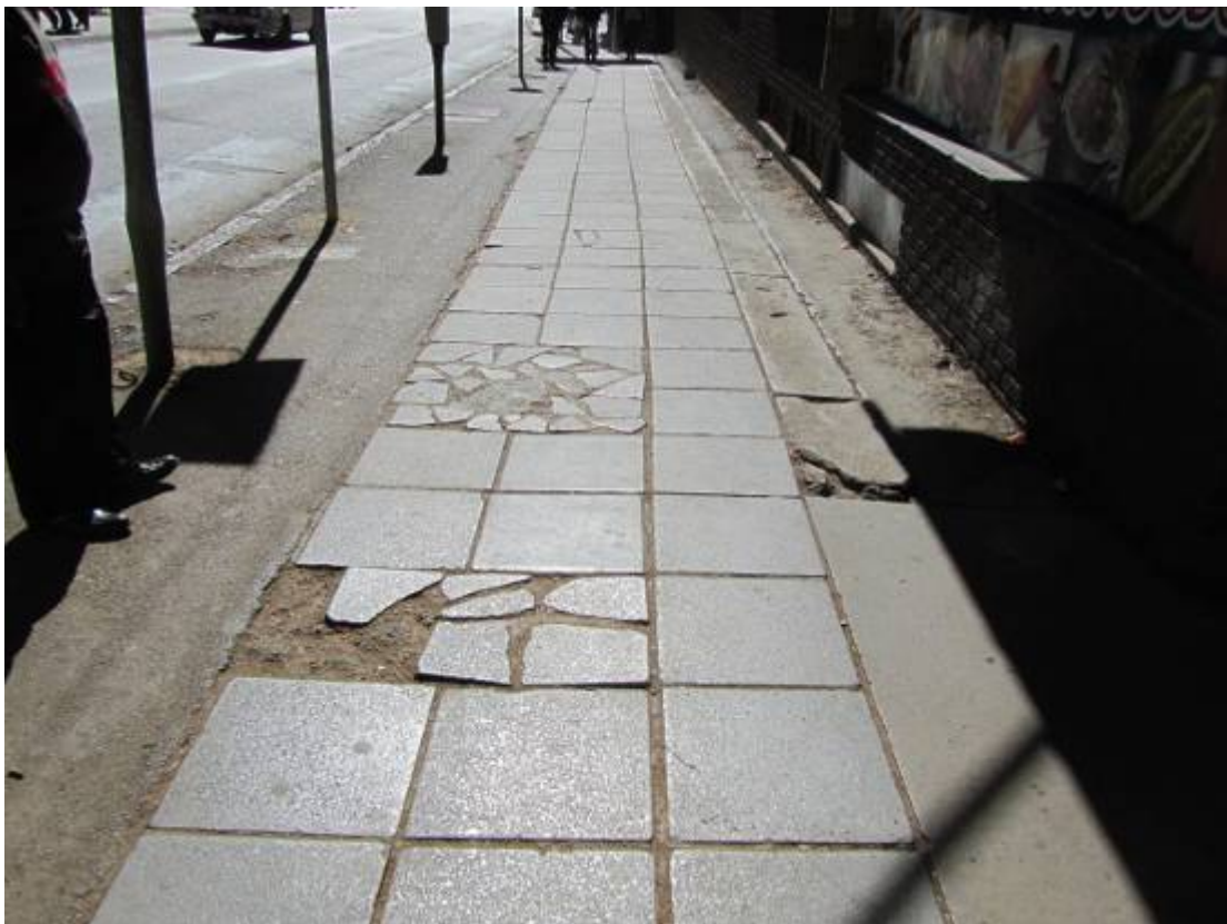
Figure 308. Another combination of paving surfaces. (P 1136)
