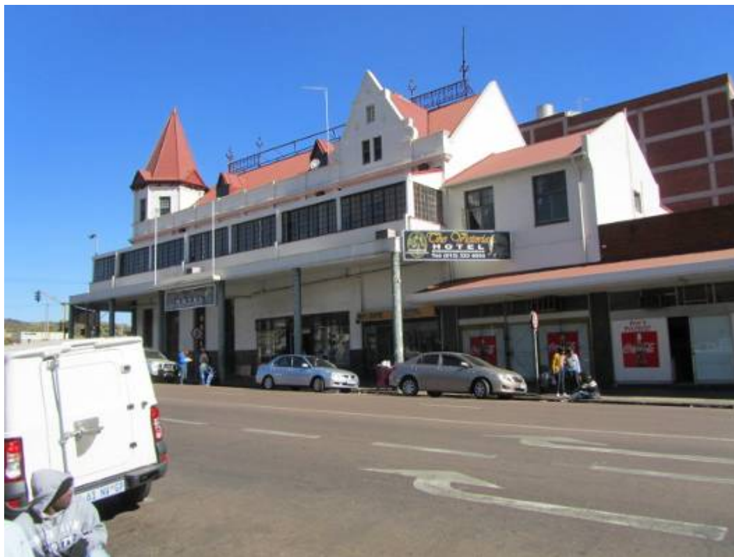
Figure 335. Protected building. (P 1113)
