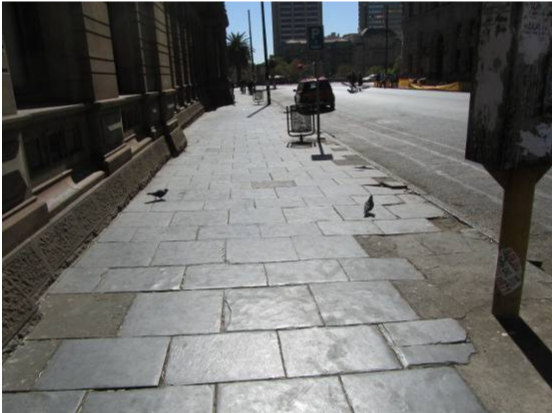
Figure 210. Historical slate paving adjacent to historical building. (P 1012).
