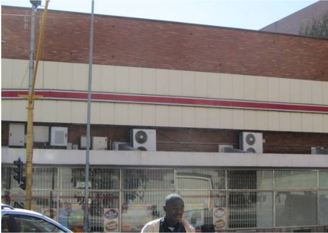
Figure 241. Provisionally protected building. (P 1039)
