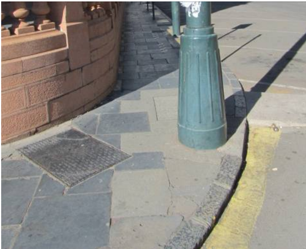
Figure 185. Historical slate paving adjacent to historical building. (P 989).
