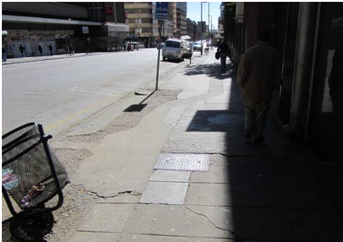
Figure 257. Variety of paving material. Note granite curbing. (P 1056)
