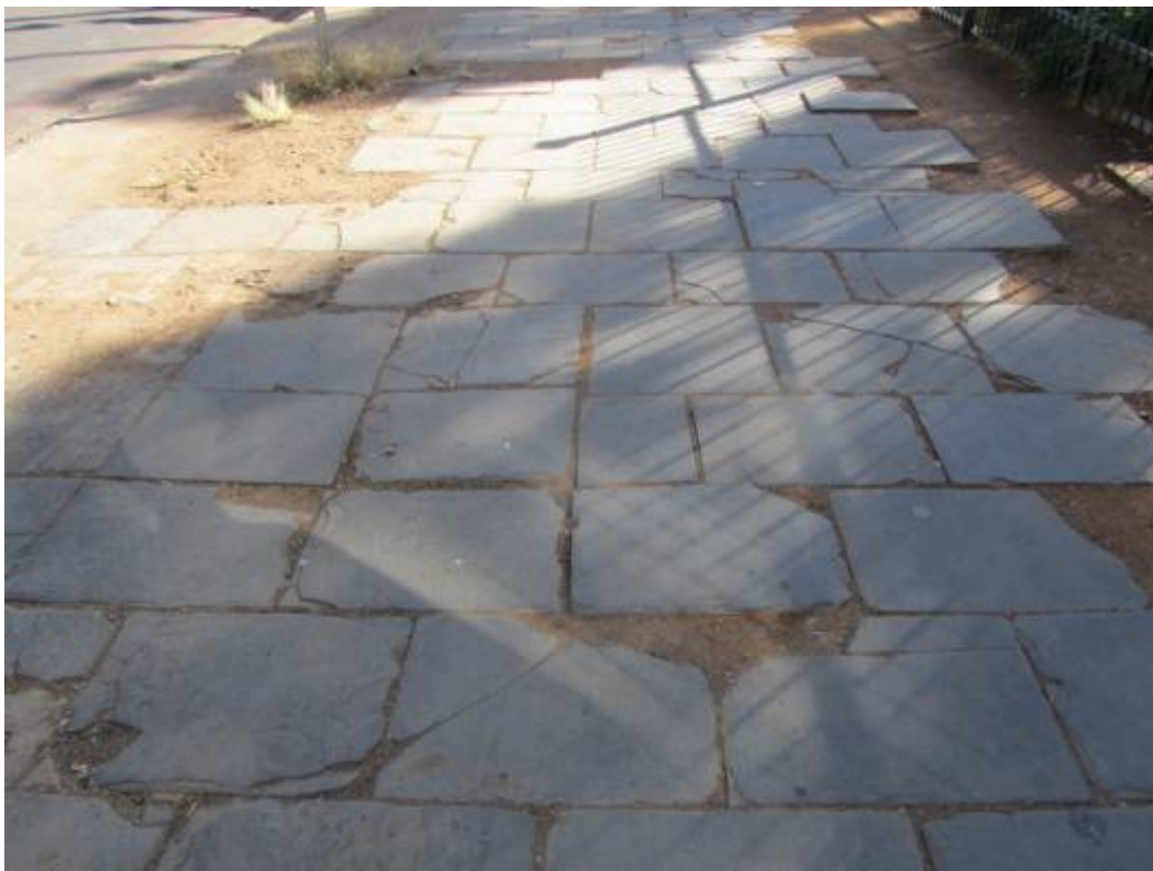
Figure 47. Historical slate paving. Protected building as noted in 1991 replaced by modern building to the right behind fencing. (P820)
