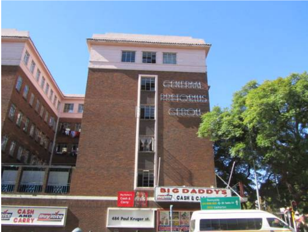
Figure 305. Protected building. (P 1133)
