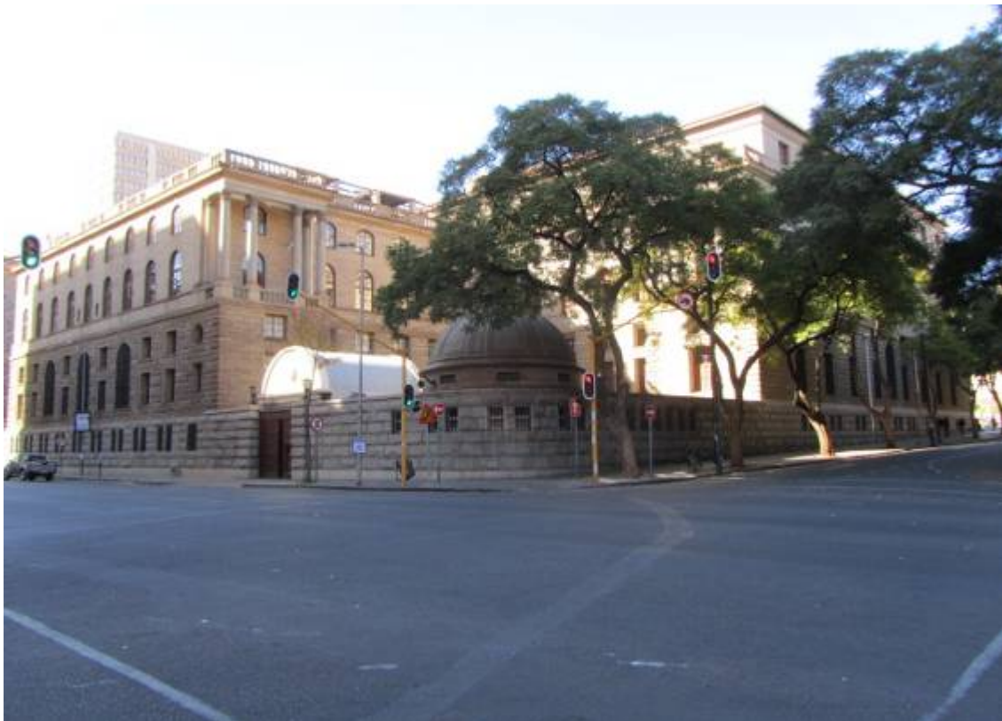
Figure 108. 'Protected building'. (P 906).
