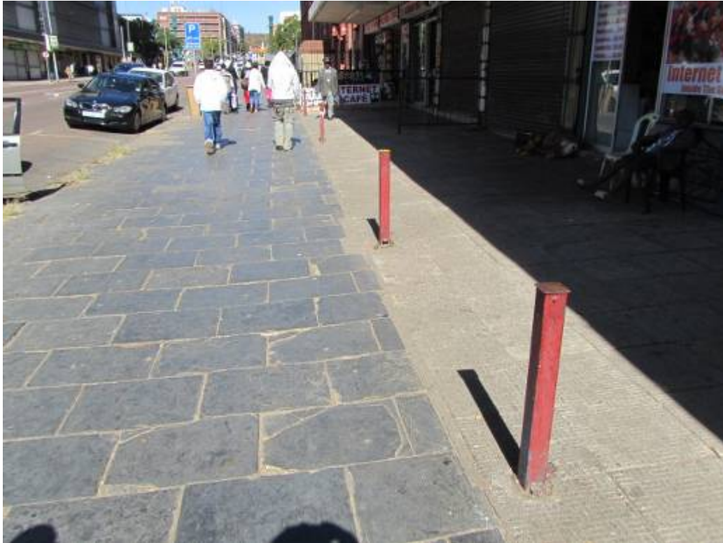
Figure 271. As mentioned before there is a distinct difference in private and public domain as illustrated here. Note that chain fence disappeared, as all things metal do in modern Tshwane. (P 1069)
