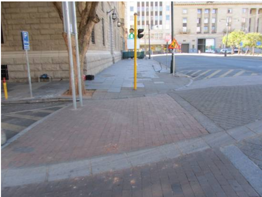
Figure 136. Historical slate paving adjacent to historical building. (P 944).
