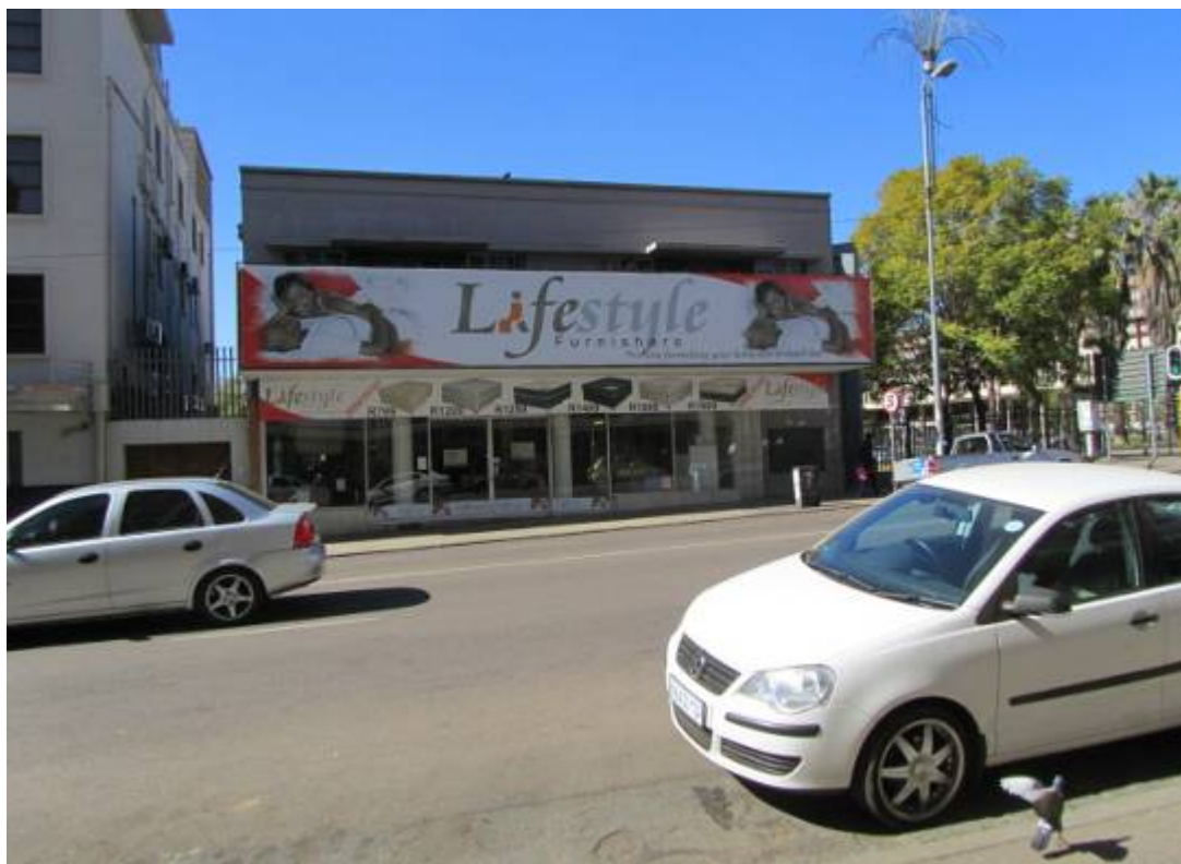
Figure 251. Provisionally protected building. (P 1049)
