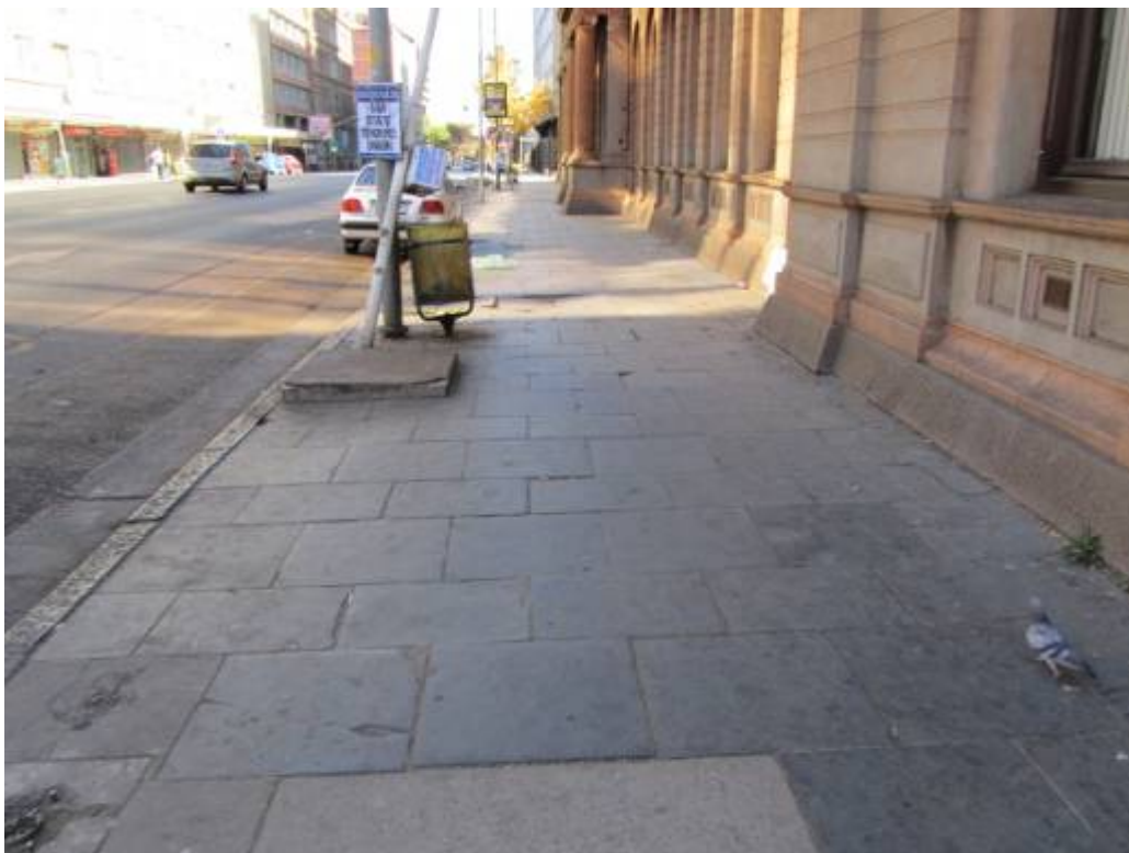
Figure 209. Historical slate paving adjacent to historical building. (P 1011).
