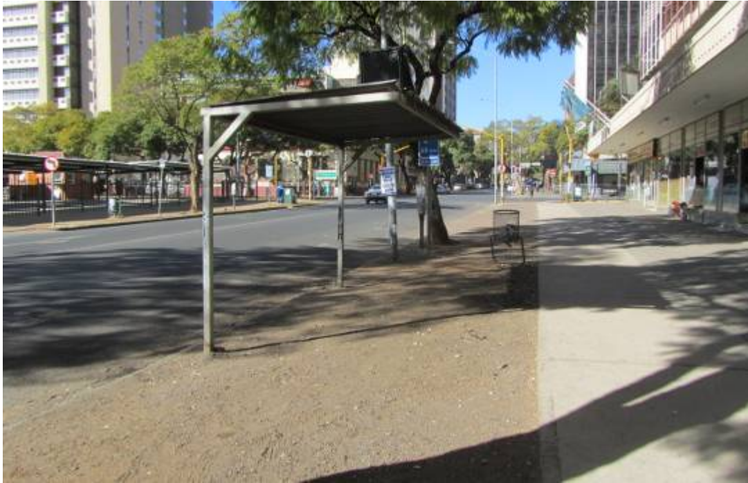
Figure 76. ‘. Strip concrete and bare earth sidewalk. Street furniture is endangered by illegal parking on sidewalks. Note fresh tire tracks on earth section. Note the extra set-off of this ‘modern’ building, widening an already wide sidewalk. (P 861).
