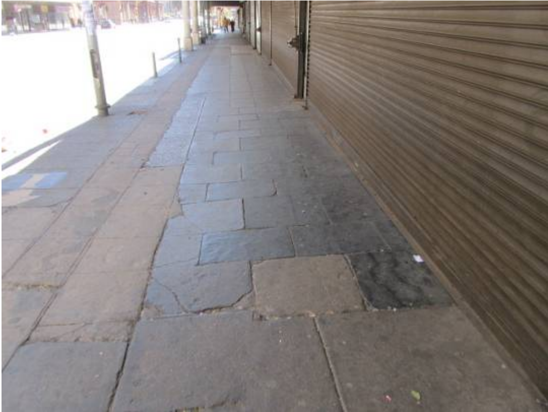
Figure 232. Cement block paving, remnants of historical slate paving and granite curbing defining old roadway. (P 1031)
