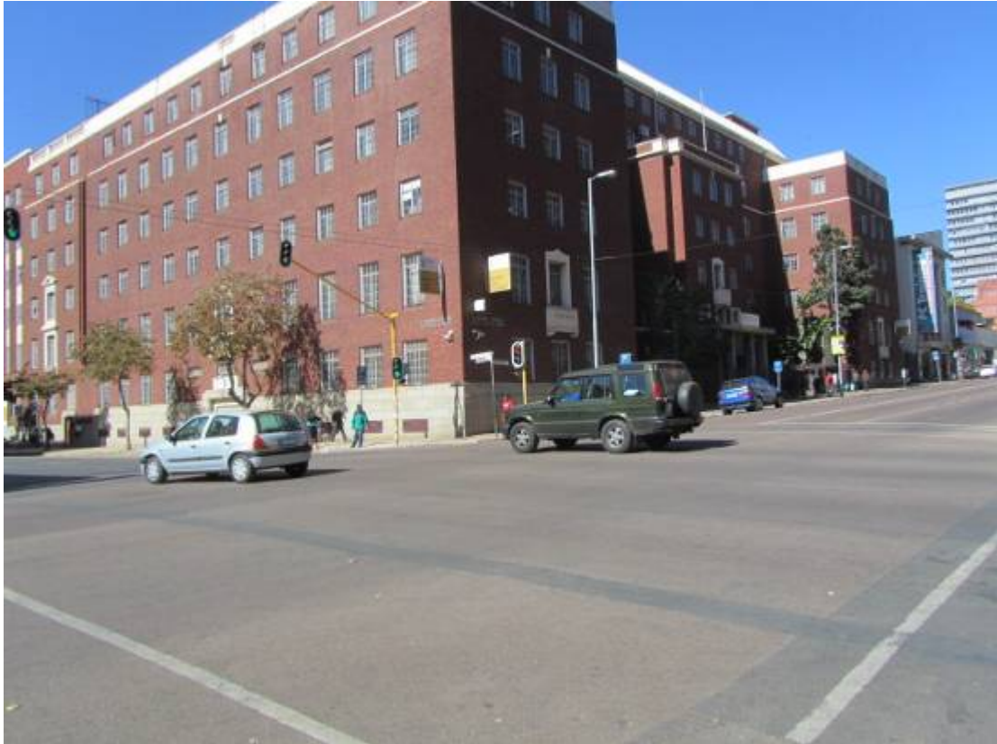
Figure 226. Protected buildings. (P 1026)
