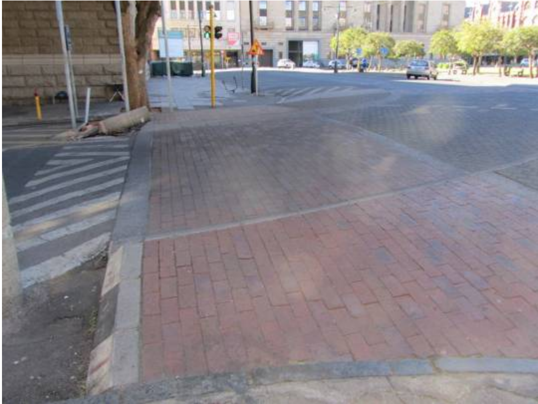
Figure 133. Modern traffic calming structure. (P 936).
