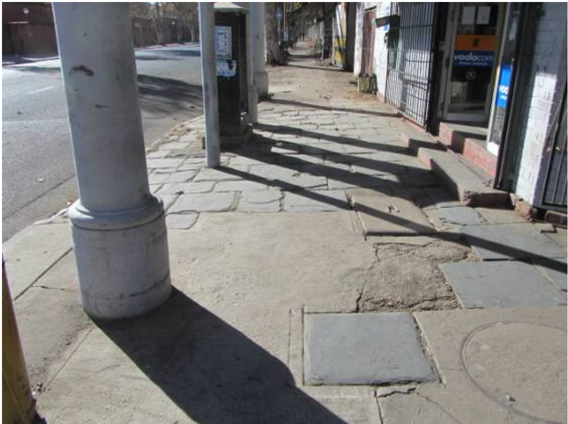
Figure 29. Historical slate sidewalk in front of 'protected building'. Granite curb stones, and pillars. (P802) Note services access.
