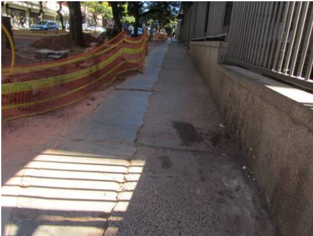
Figure 306. Services will be a continuous issue as will paving. The transition though from historic building to streetscape ought to be better than this. (P 1134)
