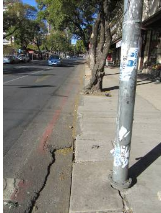
Figures 69 and 70. Granite curbing defining old roadway dimensions both on north eastern and north western sidewalks. Concrete strips are the main paving agent but offers little practical access to services. The exposed and uplifting roots of the Jacaranda trees may pose some design challenges for the paving application. (P850 and P 851).
