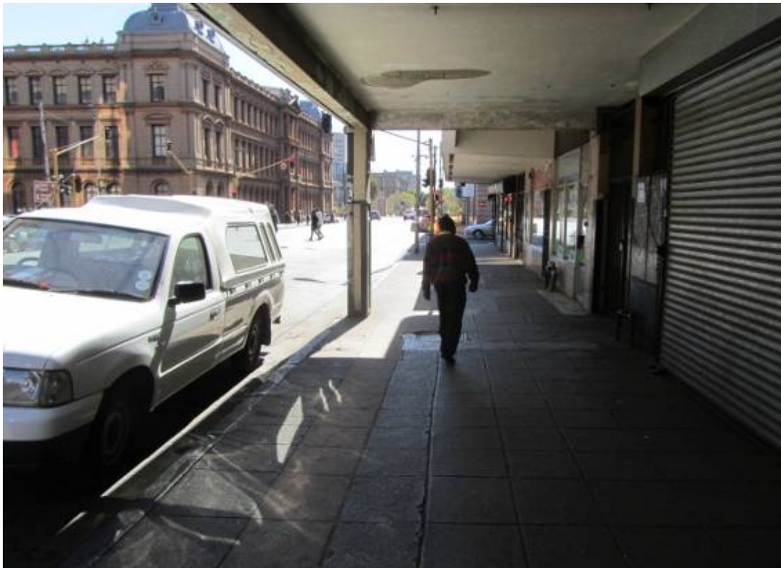
Figure 236. Variety of paving material and historical pillar footprint. Note Granite curbing. (P 1035)
