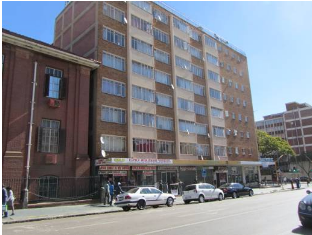
Figure 263. Provisionally protected building. (P 1060)
