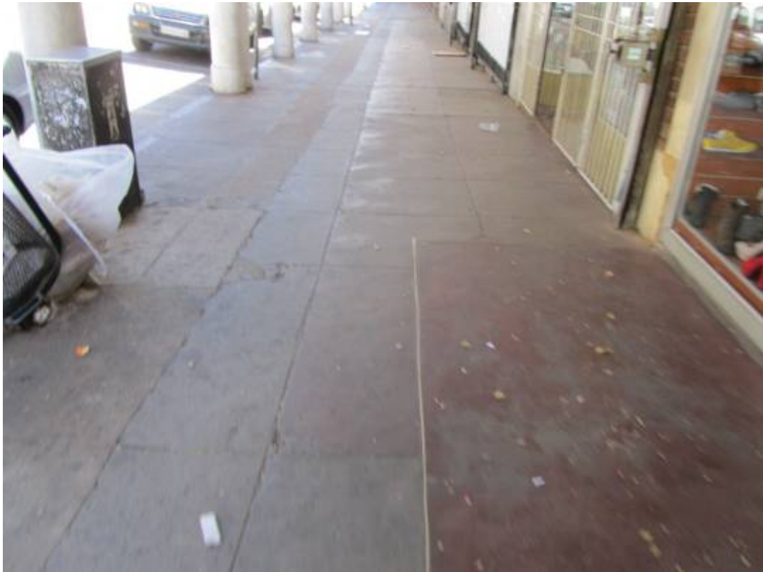
Figure 230. Variety of paving material and historical pillar footprint. (P 1029)
