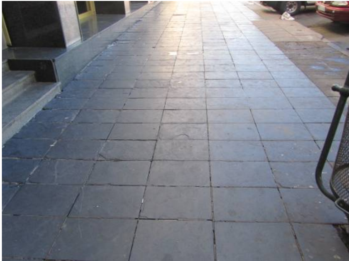
Figure 172. Well preserved slate paving in front of historical building. (P 975).
