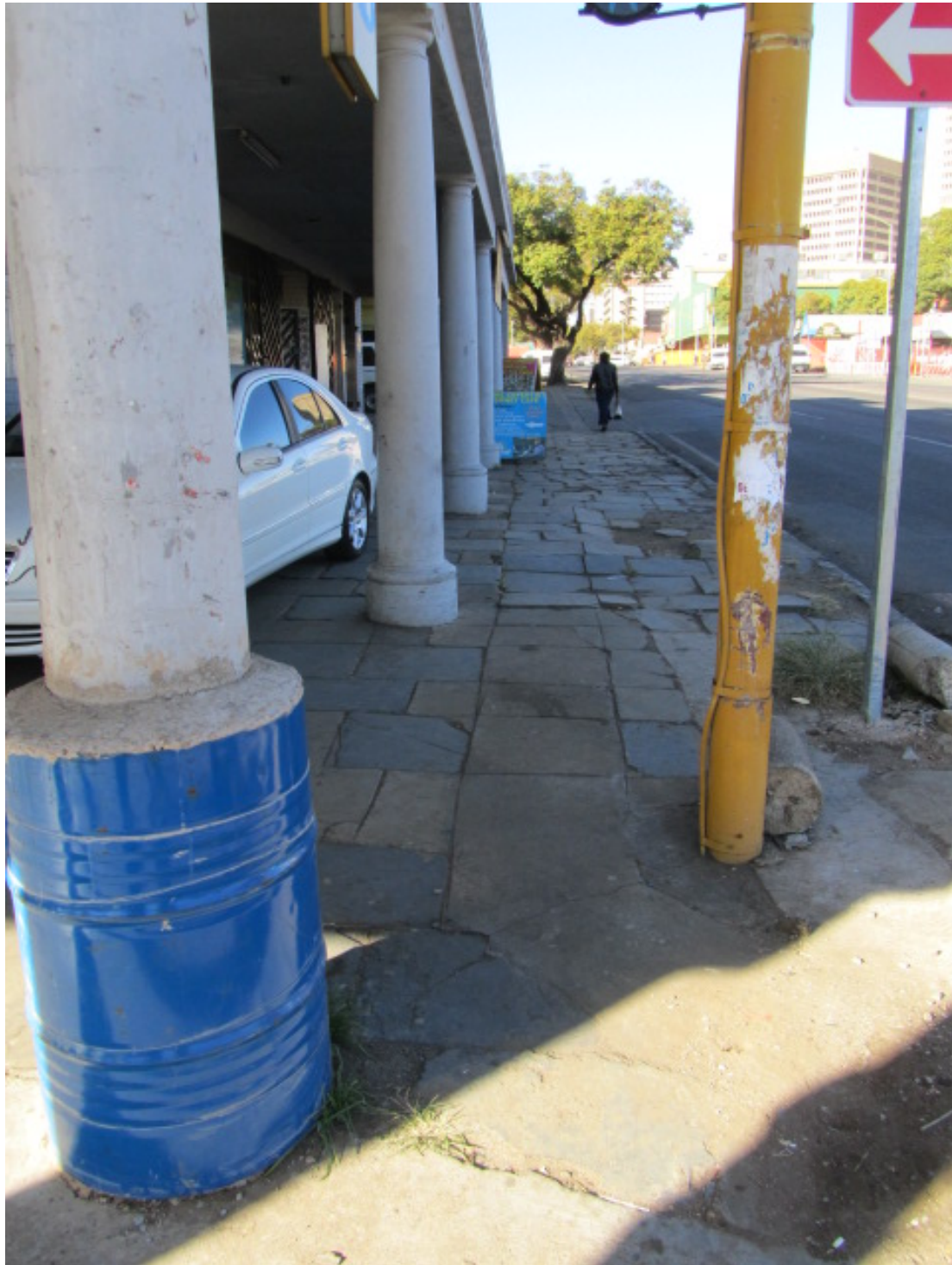
Figure 30. Historical slate sidewalk in front of ‘protected building’. Granite curb stones, and pillars. Note absence of greening. (P803).
