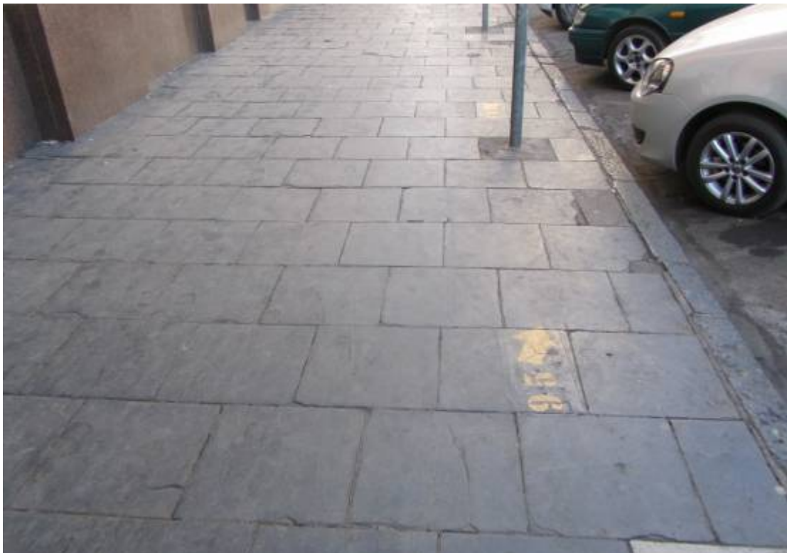
Figure 165. Well preserved historical slate paving adjacent to historical building. (P 968).
