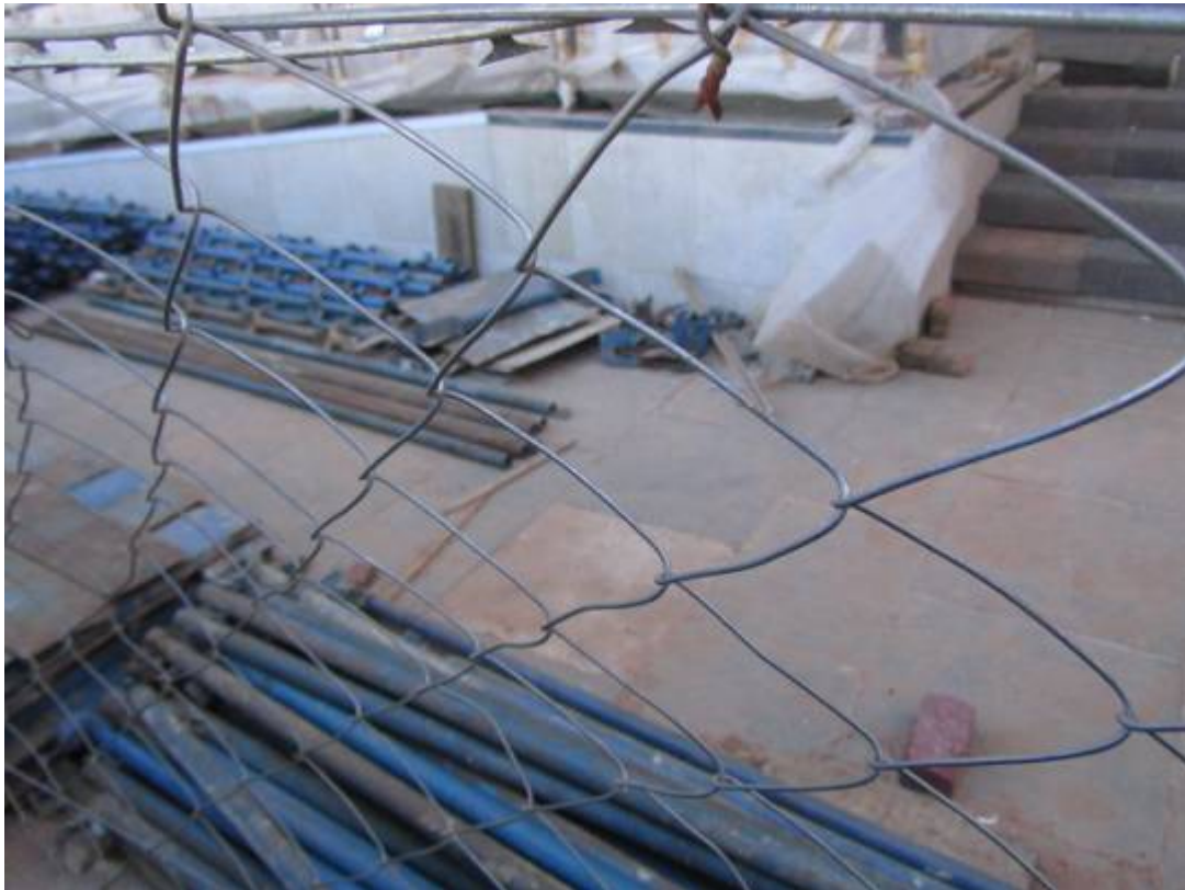
Figure 147. Construction work at historical building. (P 950).
