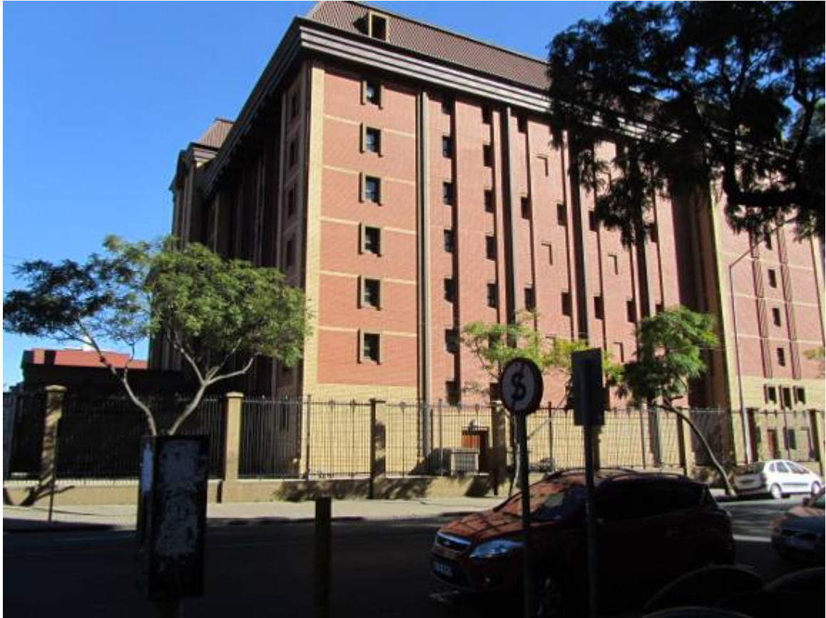
Figure 114. 'Provisionally protected building'. (P 913).
