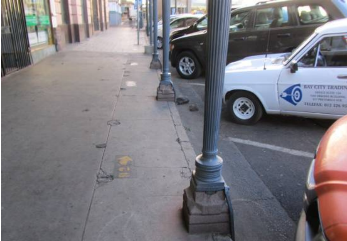
Figure 164. As mentioned in earlier documentation blocks, historical building's columns to support the canopy were mostly located on the street line as demonstrated here. (P 967).
