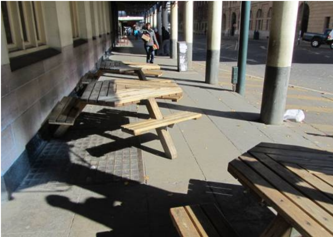
Figure 196. Large cement blocks as paving adjacent to historical building. Pillars defining sidewalk limit. (P 999).
