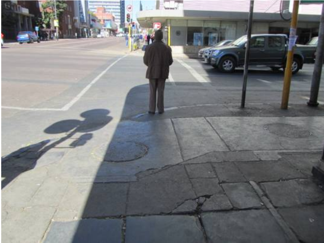
Figure 224. Cement block paving, remnants of historical slate paving and granite curbing defining old roadway. (P 1024)
