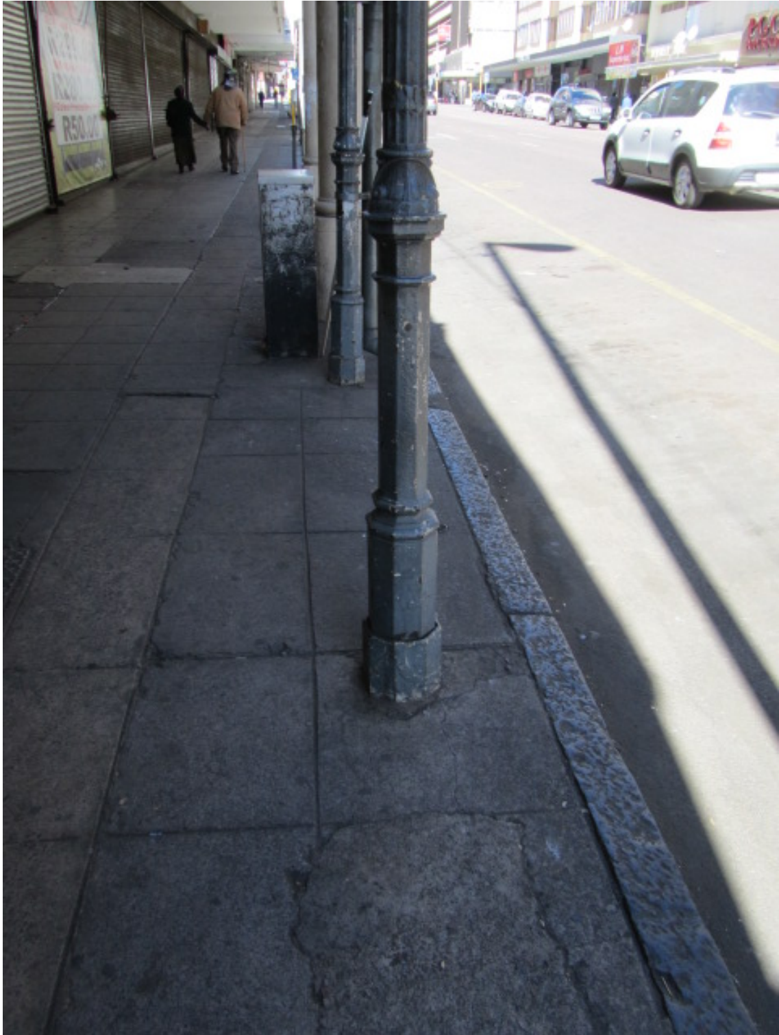
Figure 234. Variety of paving material and historical pillar footprint. Note Granite curbing. (P 1034)
