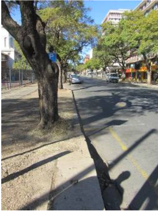
Figures 69 and 70. Granite curbing defining old roadway dimensions both on north eastern and north western sidewalks. Concrete strips are the main paving agent but offers little practical access to services. The exposed and uplifting roots of the Jacaranda trees may pose some design challenges for the paving application. (P850 and P 851).
