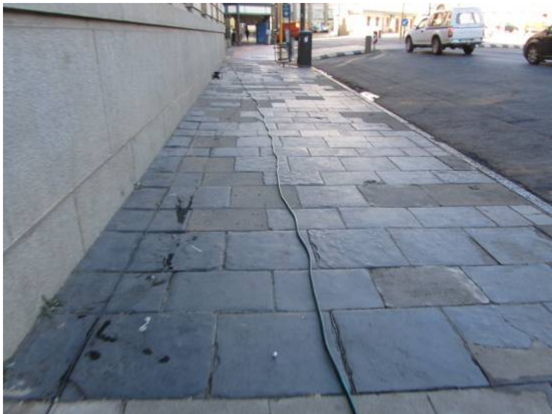
Figure 156. Well preserved slate paving in front of historical building. (P 959).
