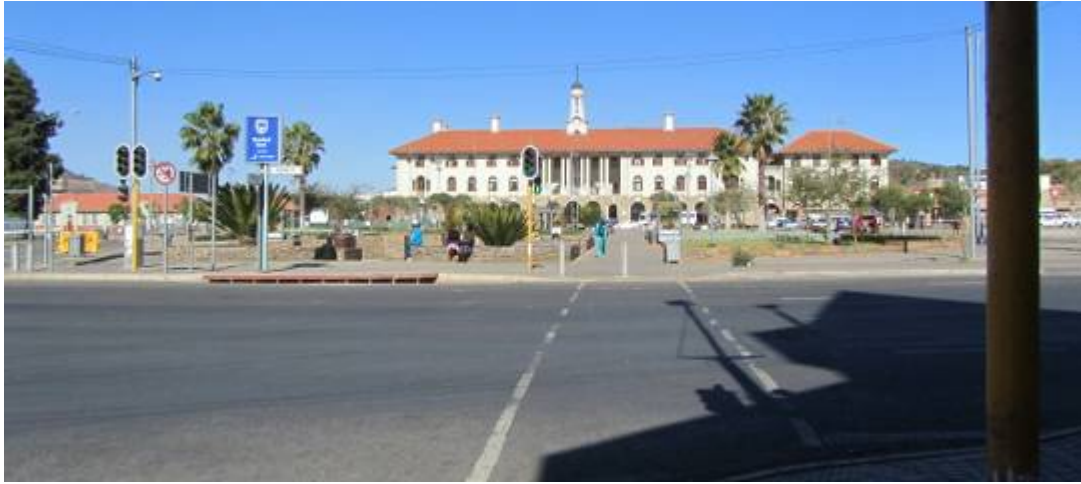
Figure 344. Protected building. (P 1103)
