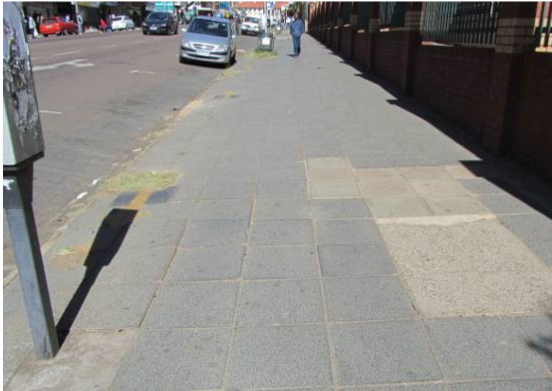
Figure 299. Granite curbing and unsightly paving. (P 1124)
