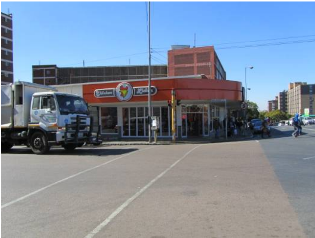
Figure 330. Provisionally protected building. (P 1104)
