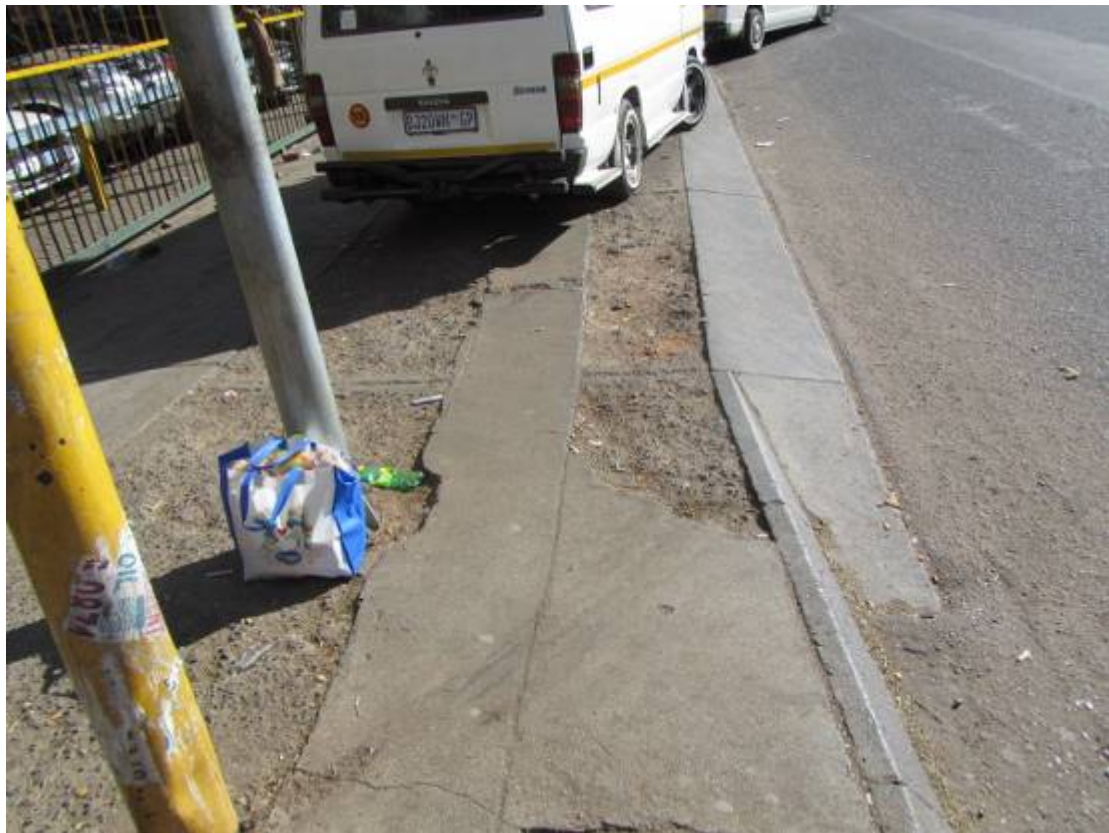
Figure 38. Modern sidewalk and curbing. (P813)
