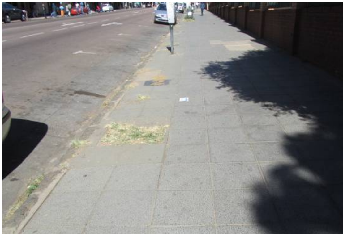
Figure 298. Cement block paving. (P 1123)
