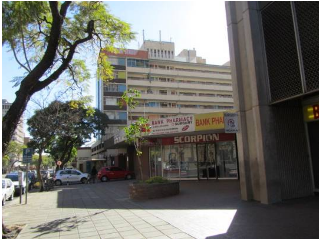
Figure 117. 'Provisionally protected building'. (P 915).
