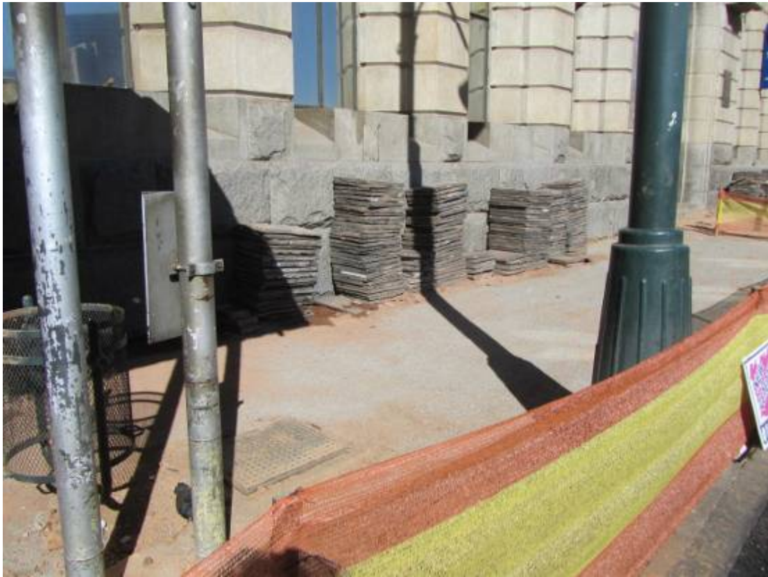
Figure 174. Slate paving in front of historical building being lifted. (P 977).
