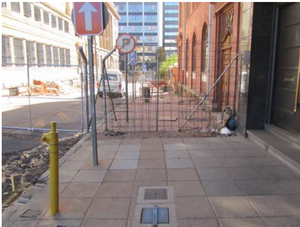
Figure 151. Cement block paving adjacent to historical building. (P 954).
