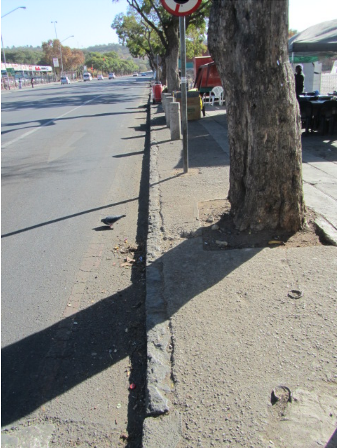
Figure 39. Original granite curbing. (P816)
