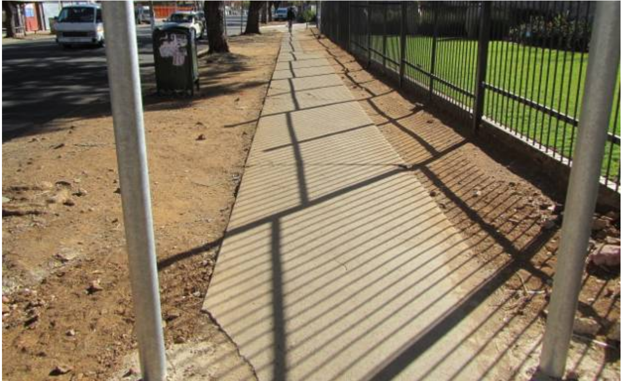
Figure 61. Modern strip concrete paving bordered with bare earth. Granite curbing still demarcates original dimensions. The modern building to the right has a well defined green landscape that is a feature that may be incorporated in the new design. (P 837)
