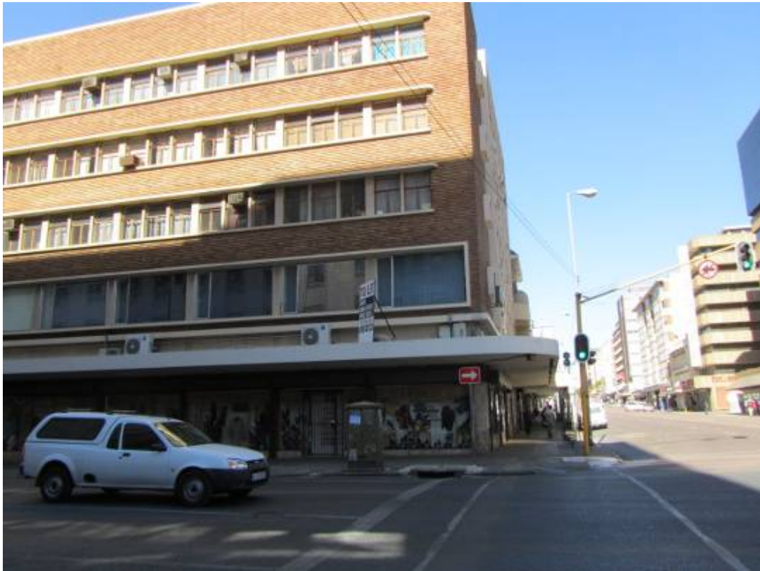
Figure 206. Provisional historical building. (P 1008).
