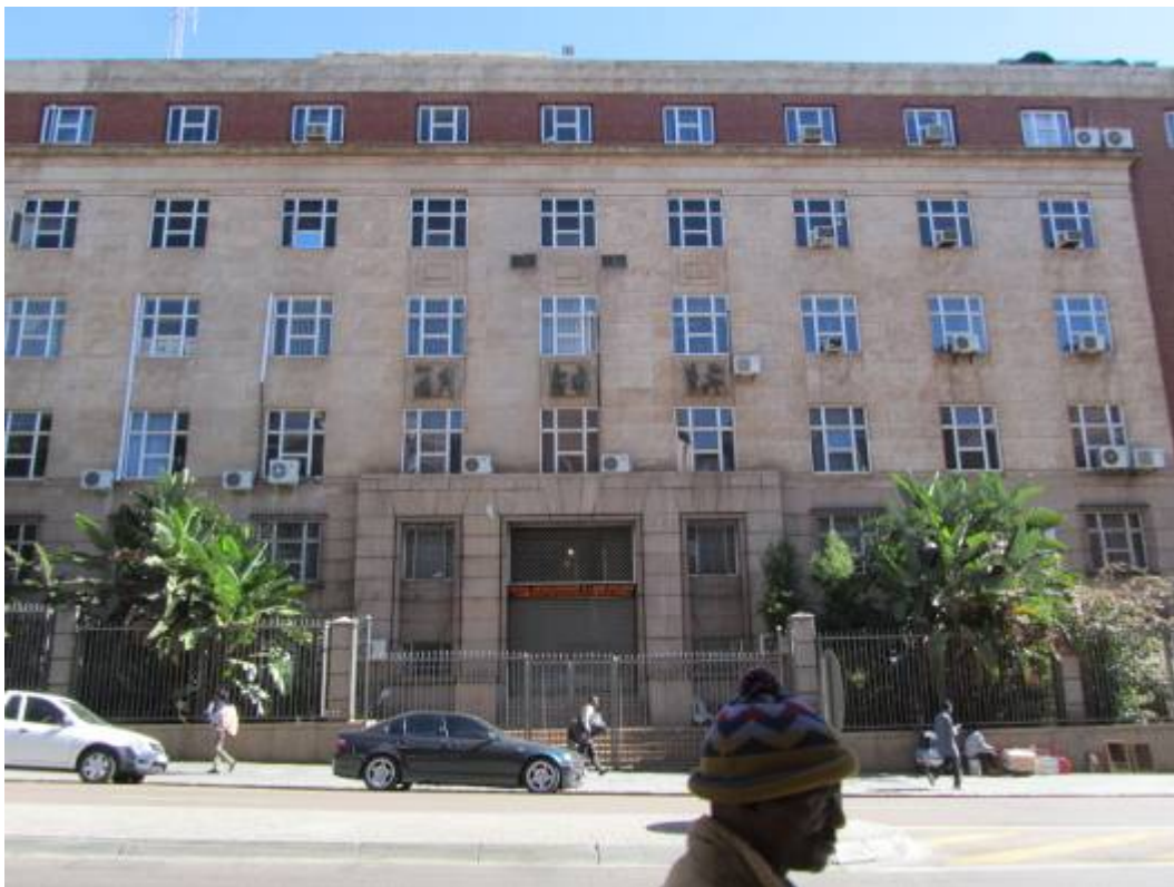
Figure 310. Protected building. (P 1138)
