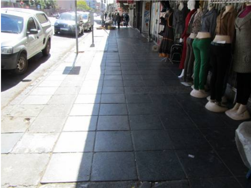
Figure 340. Cement block paving. (P 1116)
