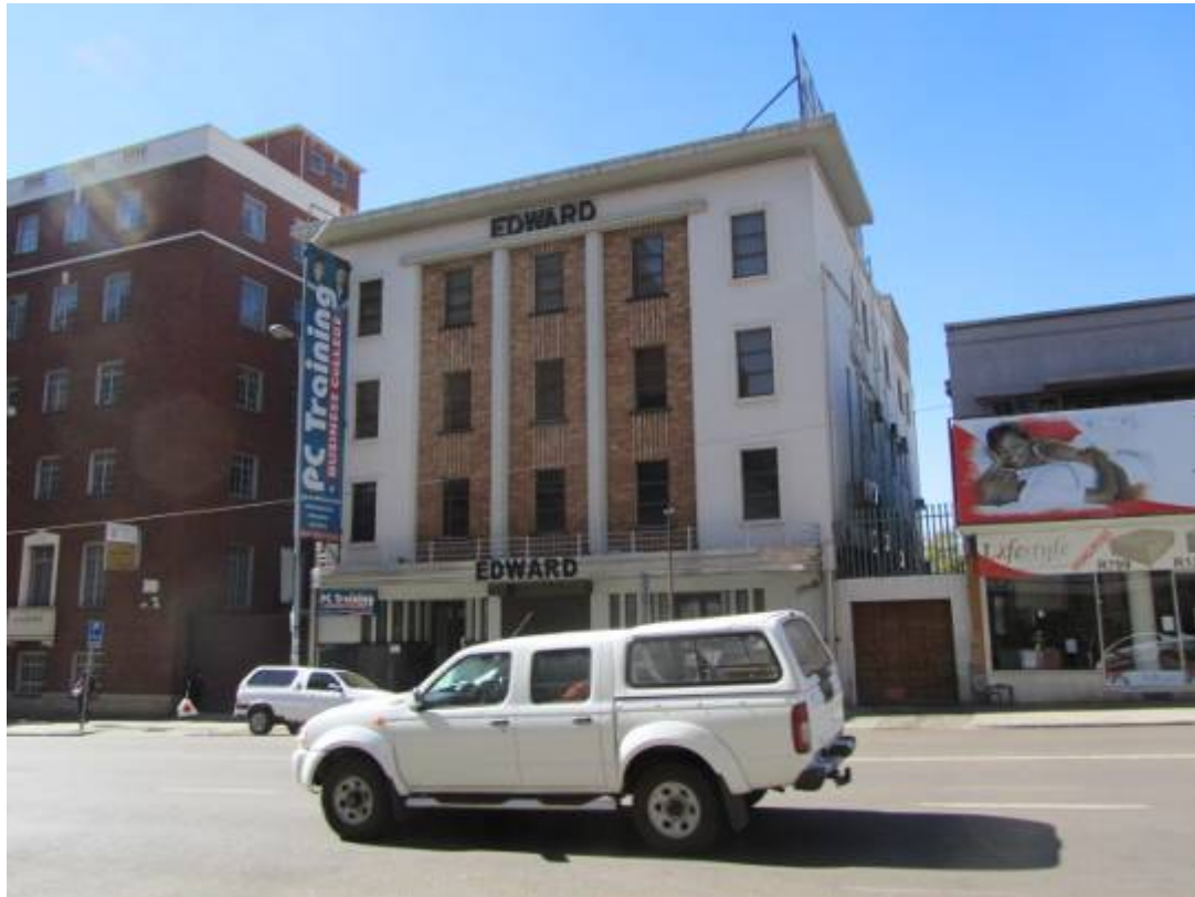
Figure 250. Protected building. (P 1048)
