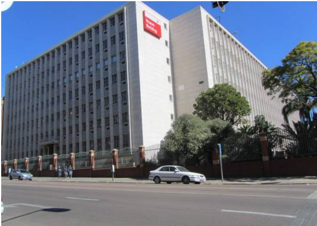
Figure 294. Protected building. Note again the separation of private and public domain regarding 'sidewalk'. (P 1119)
