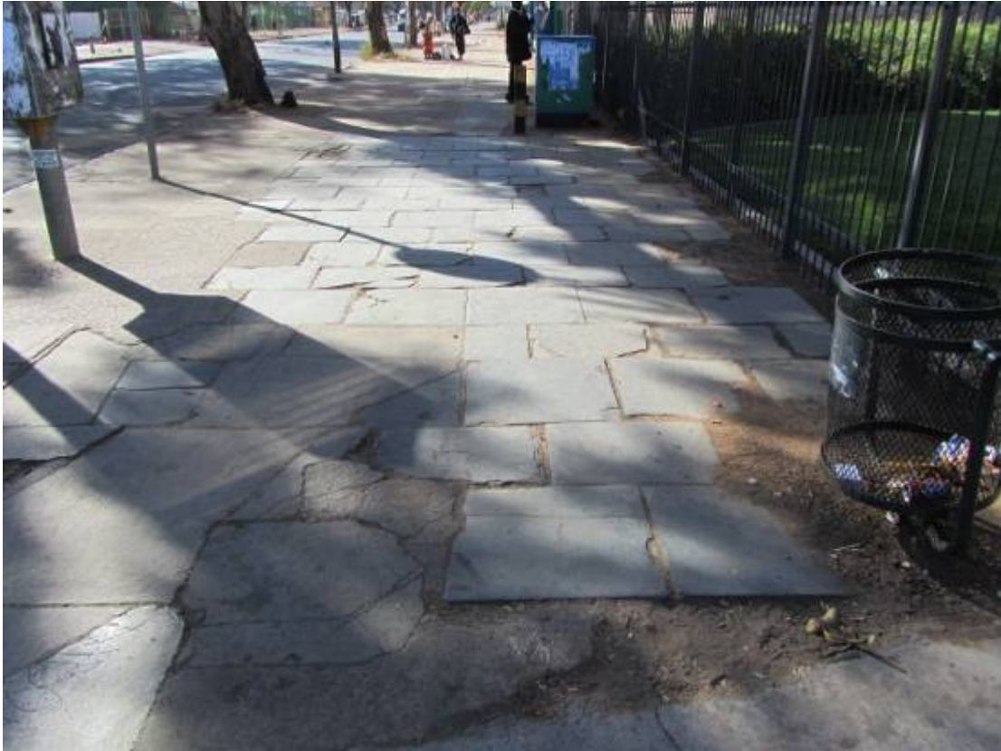
Figure 48. Historical slate paving. Protected building as noted in 1991 replaced by modern building to the right behind fencing. (P821)
