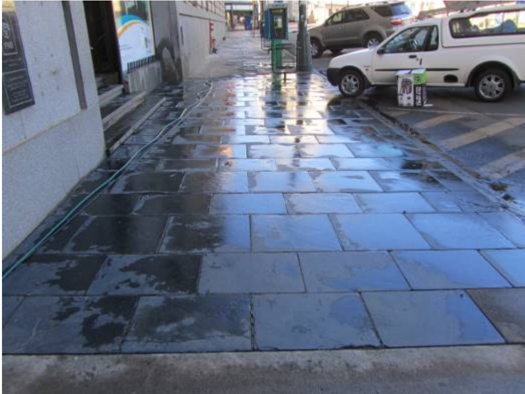
Figure 153. Pristine slate paving in front of historical building. (P 956).
