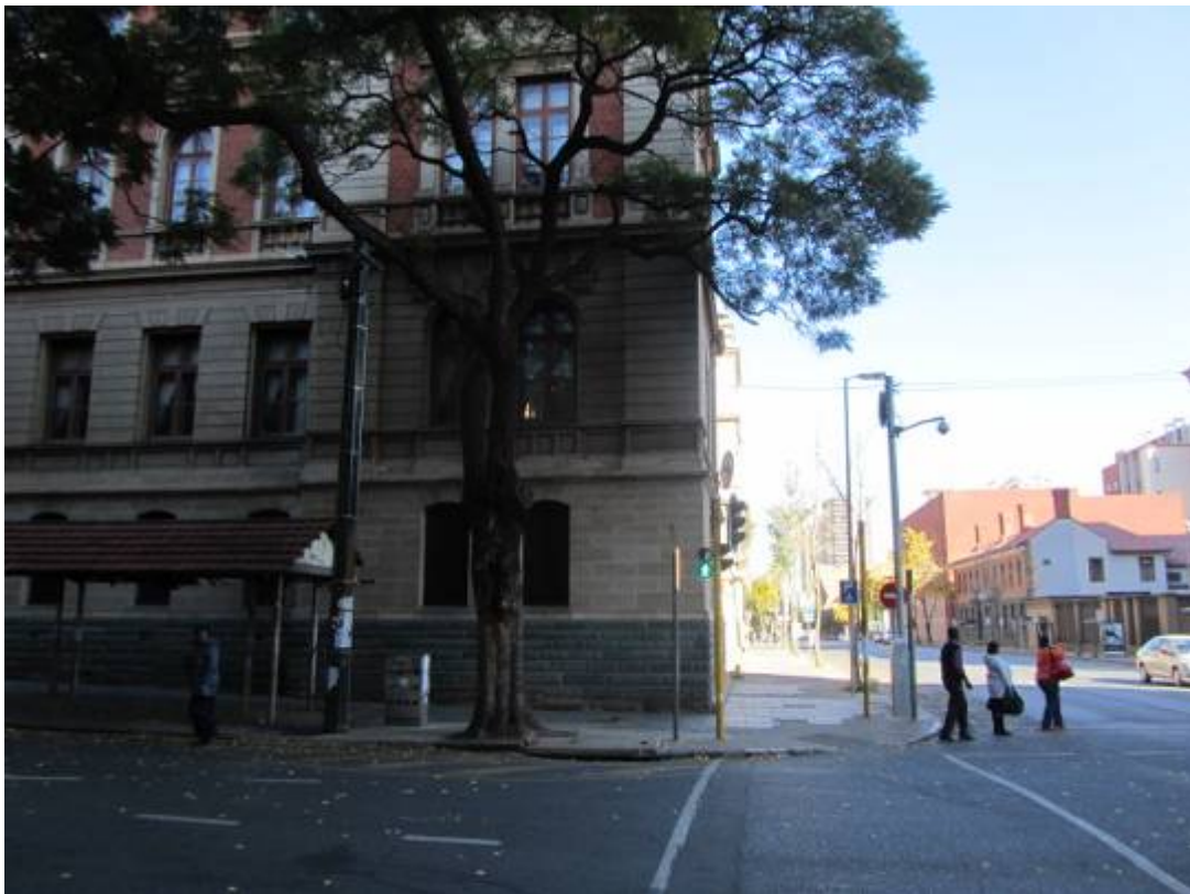
Figure 126. Historic building. (P 926).
