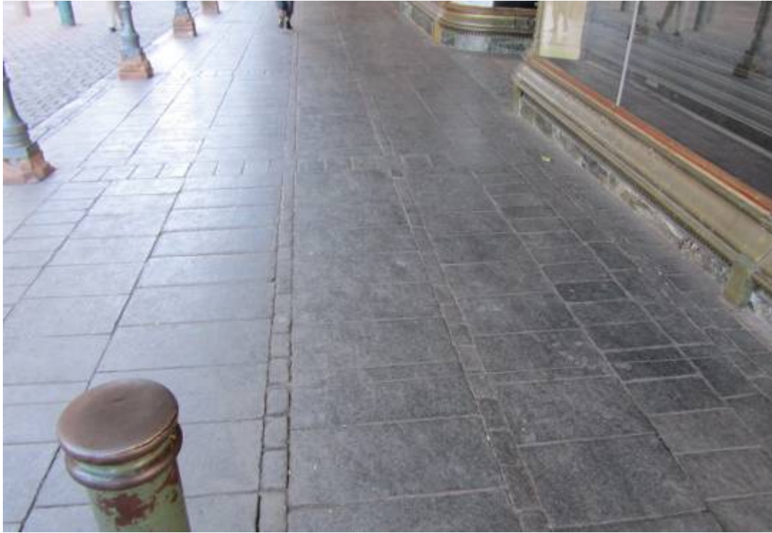
Figure 162. The refurbished paving in the Church Street Boulevard is excellent. Note the fact that the Sidewalk and roadway now interface on the same level forming a far better aesthetical design. (P 965).
