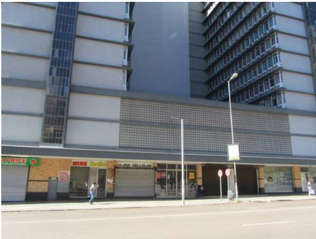
Figure 274. Provisionally protected building. (P 1072)
