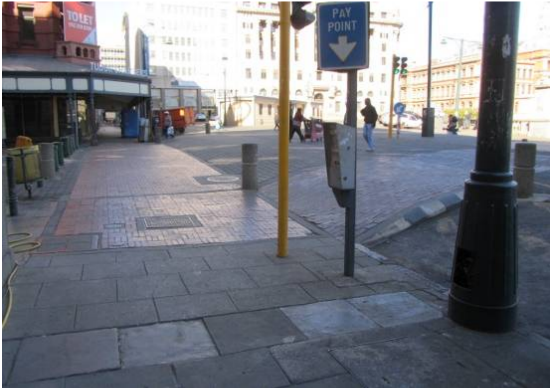
Figure 157. Mixed old and new paving at Church Street pedestrian boulevard. Note marked difference in road level. (P 960).
