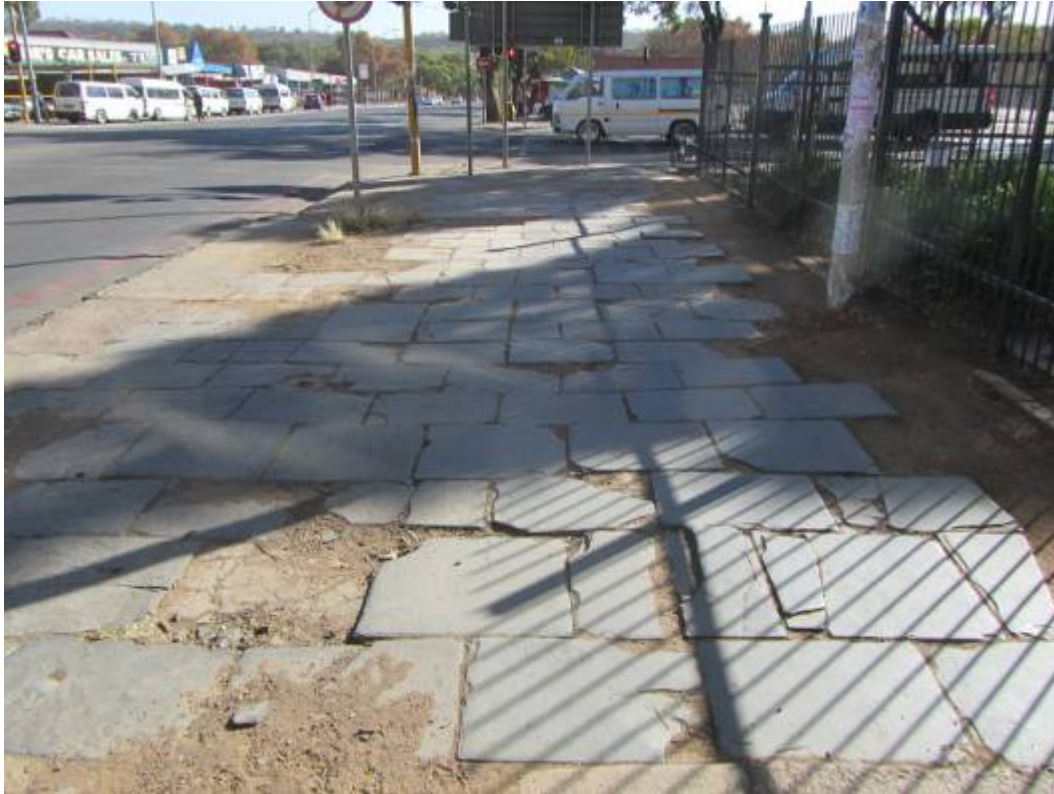
Figure 46. Historical slate paving. Protected building as noted in 1991 replaced by modern building to the right behind fencing. (P819)
