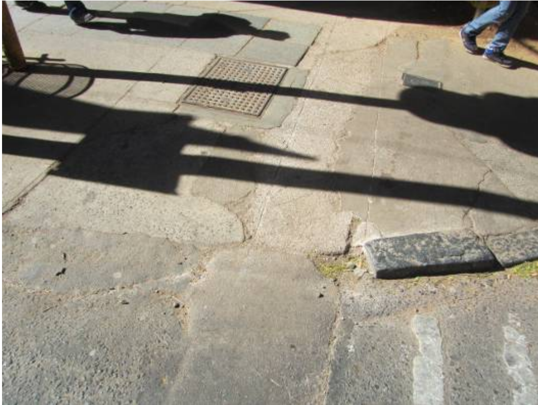
Figure 307. Paving, services and wheelchair access in combat. (P 1135)
