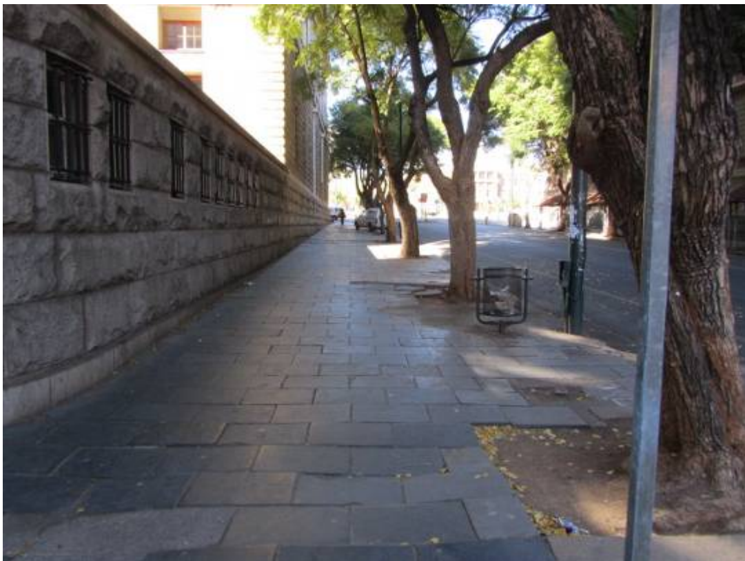
Figure 123. Discontinuation and interrupted occurrence of historical slate paving along foundations of historical buildings. (P 923).
