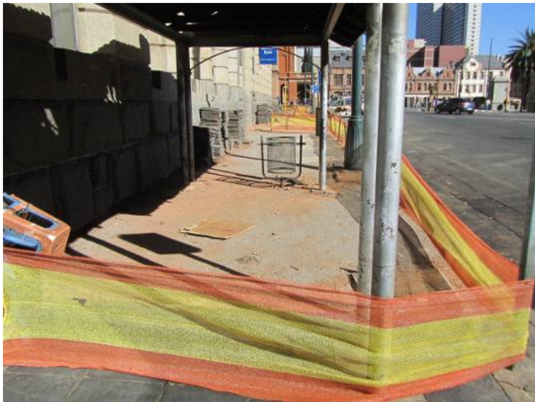
Figure 173. Slate paving in front of historical building being lifted. (P 976).
