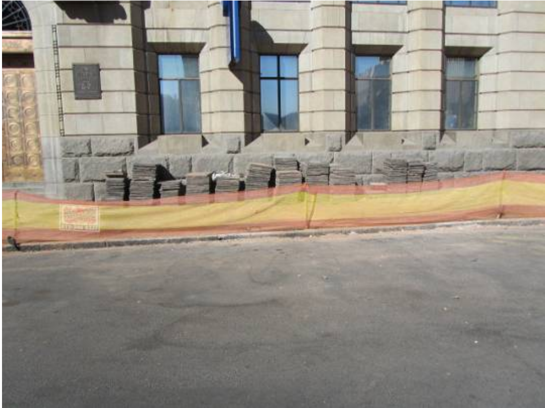
Figure 178. Slate paving in front of historical building being lifted. (P 981).
