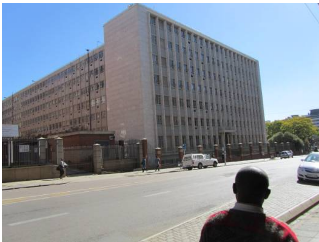
Figure 312. Protected building. (P 1140)
