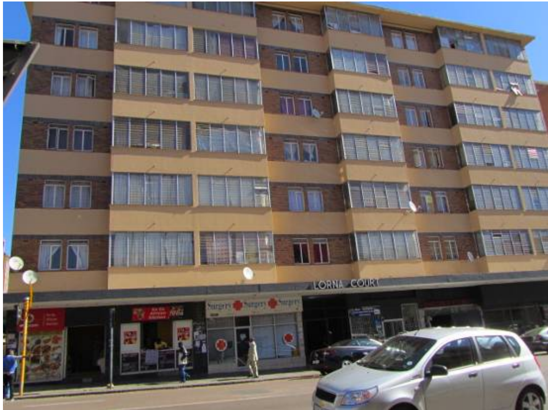
Figure 228. Provisionally protected building. (P 1028)
