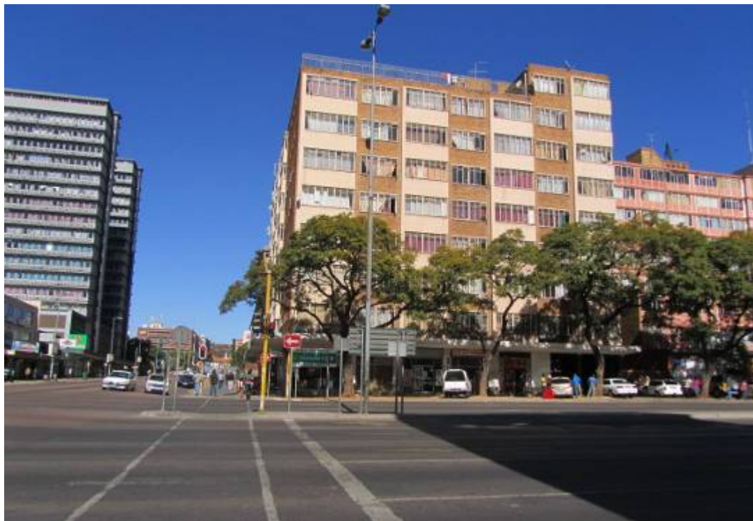
Figure 253. Provisionally protected building. (P 1051)
