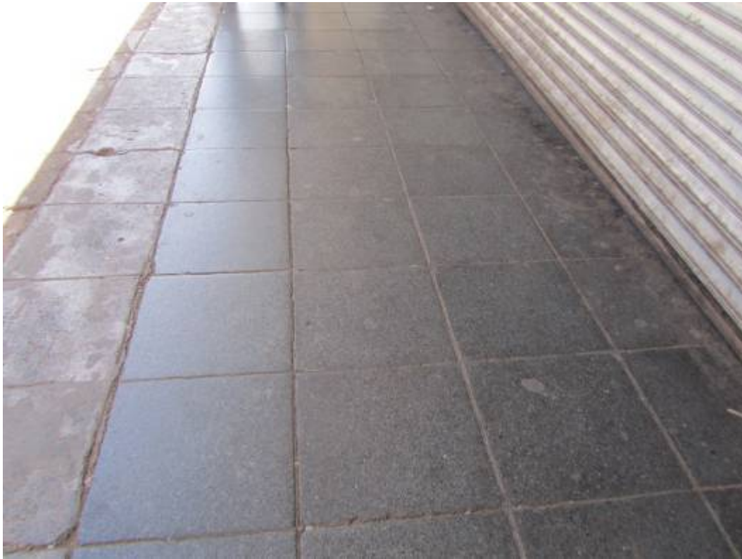
Figure 334. Cement block paving. (P 1109)
