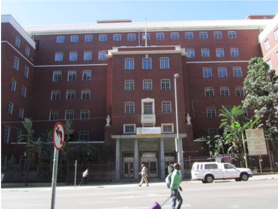
Figure 248. Protected building. (P 1046)
