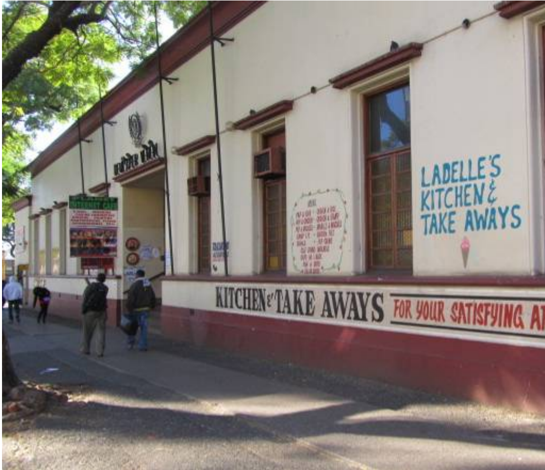
Figure 95. 'Protected building'. (P 879).
