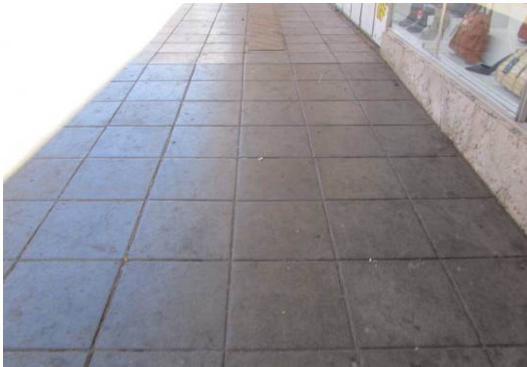
Figure 247. This 'glossy' cement blocks appears to be of an earlier application. (P 1045)
