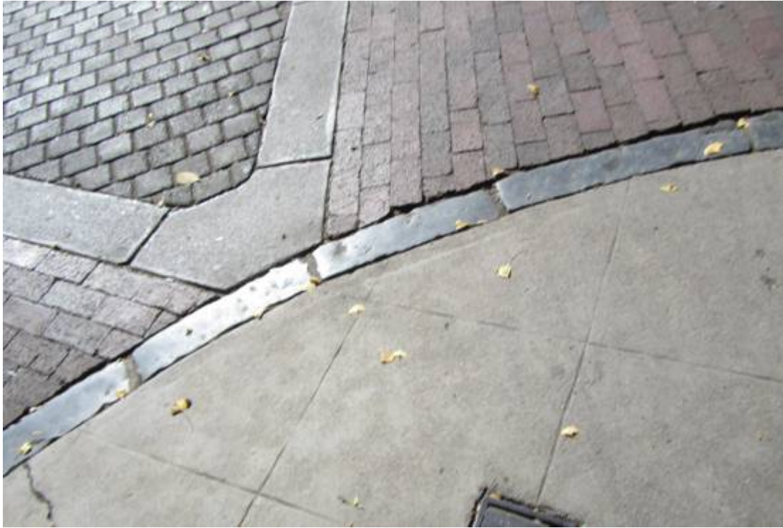
Figure 197. Although a number of different paving materials were used we find that the original curb stones are still in place. (P 1000).
