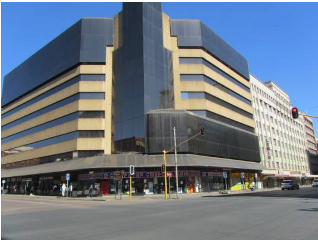
Figure 207. Provisional historical building. (P 1009).
