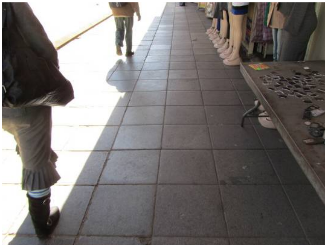
Figure 311. Cement block paving. (P 1139)
