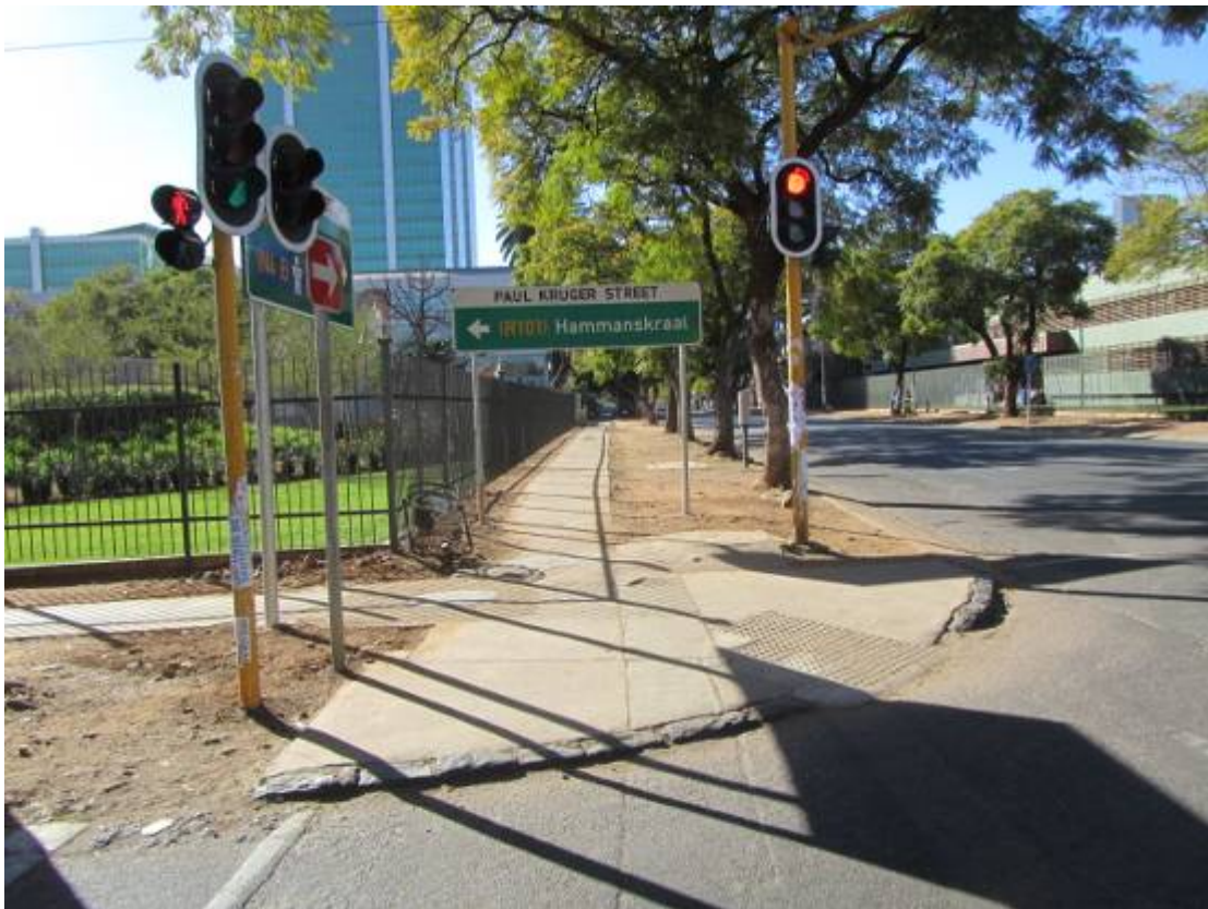
Figure 60. Granite curbing can and was adapted at street corners to accommodate disadvantaged people. (P 835)
