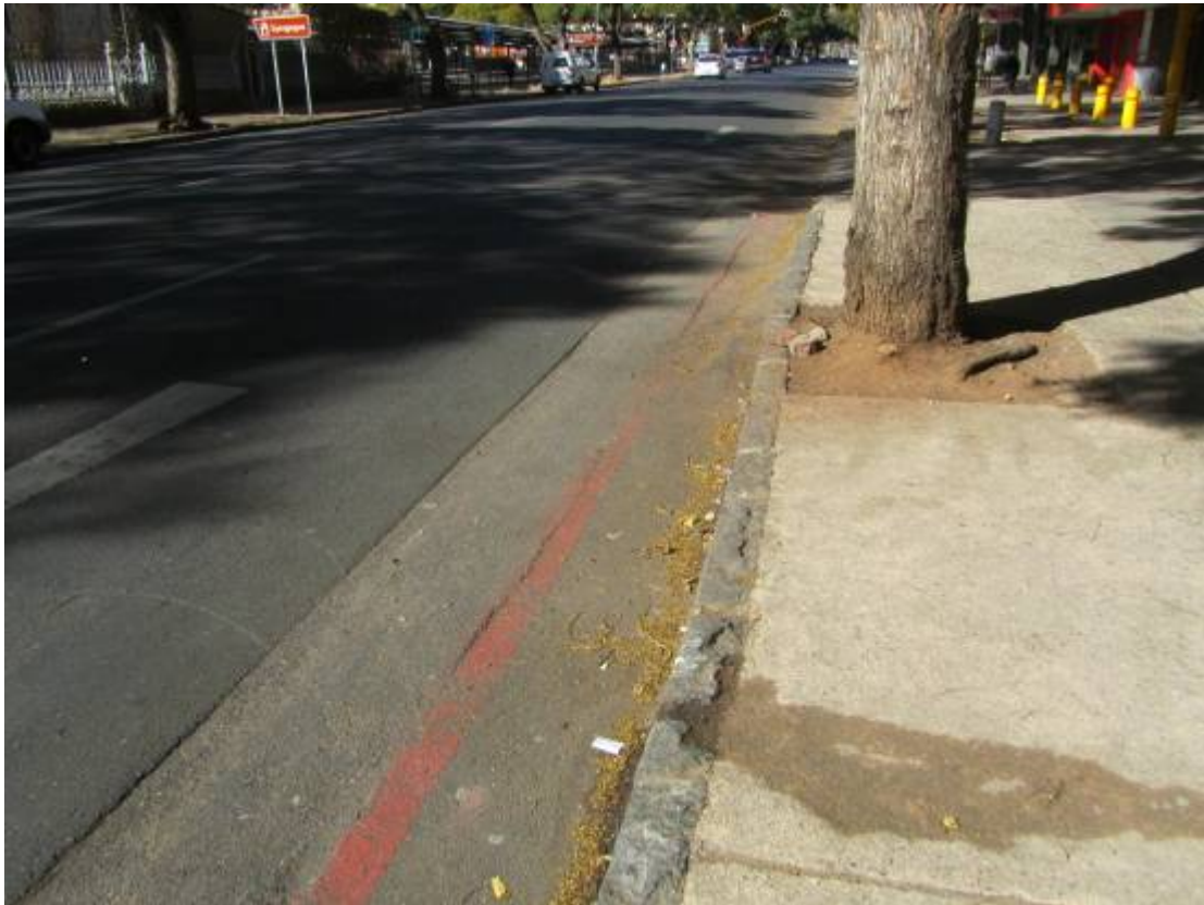
Figure 72. 'Granite curbing'. (P 854)
