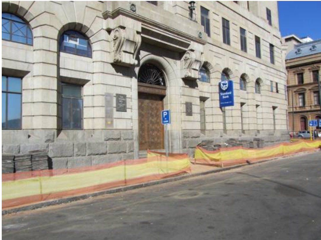
Figure 176. Slate paving in front of historical building being lifted. (P 979).
