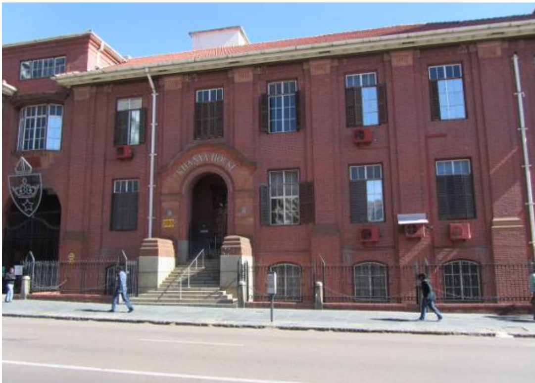
Figure 262. Protected buildings. (P 1059)
