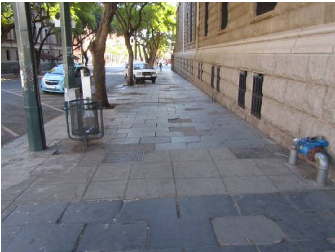
Figure 138. Historical slate paving adjacent to historical building. (P 946).
