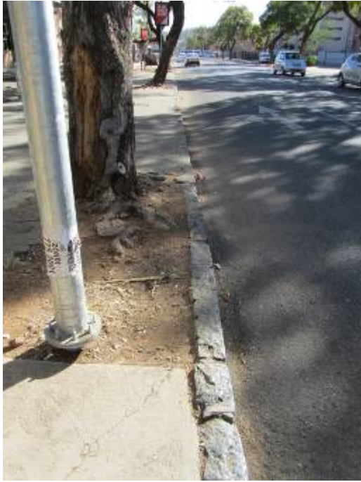
Figures 58 and 59. Granite curbing. The exposed and uplifting roots of the Jacaranda trees may pose some design challenges for the paving application. (P834 and P 836).
