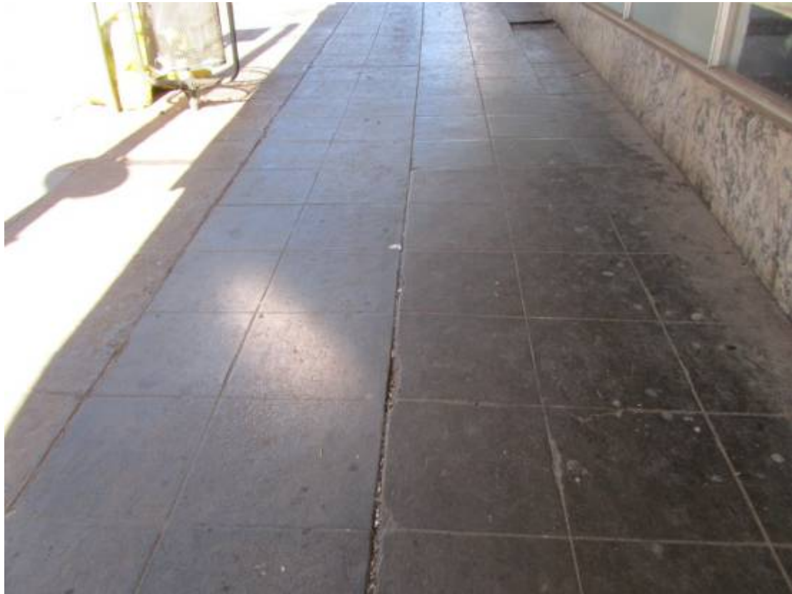
Figure 246. Variety of paving material. This 'glossy' cement blocks appears to be of an earlier application. (P 1044)
