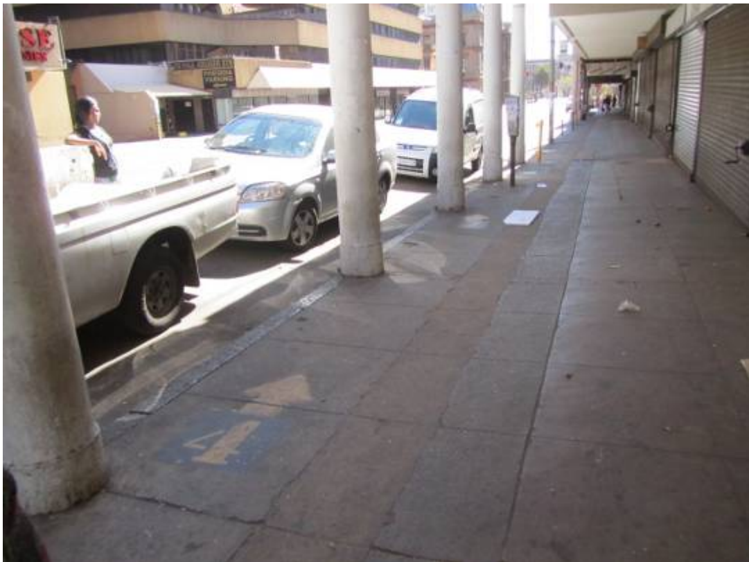
Figure 231. Variety of paving material and historical pillar footprint. (P 1030)
