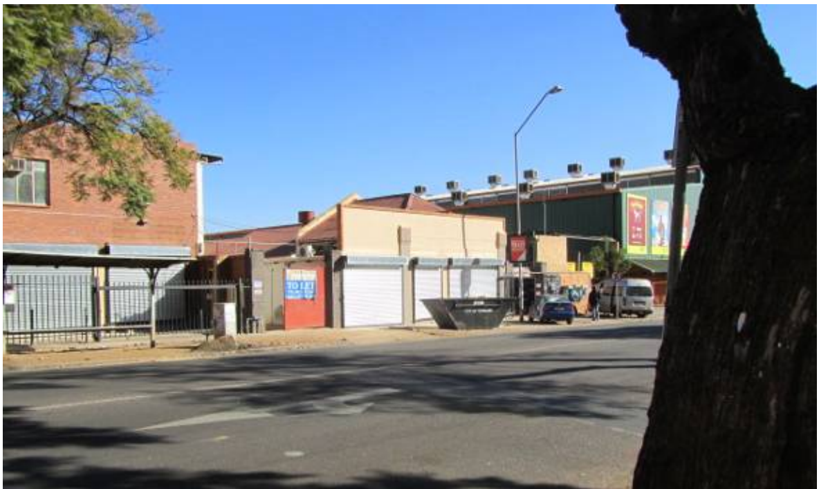
Figure 62. 'Protected building' flanked by modern structures. (P 840)
