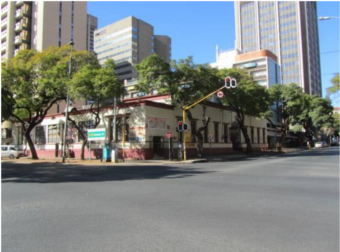
Figure 82. 'Protected building'. (P 869).
