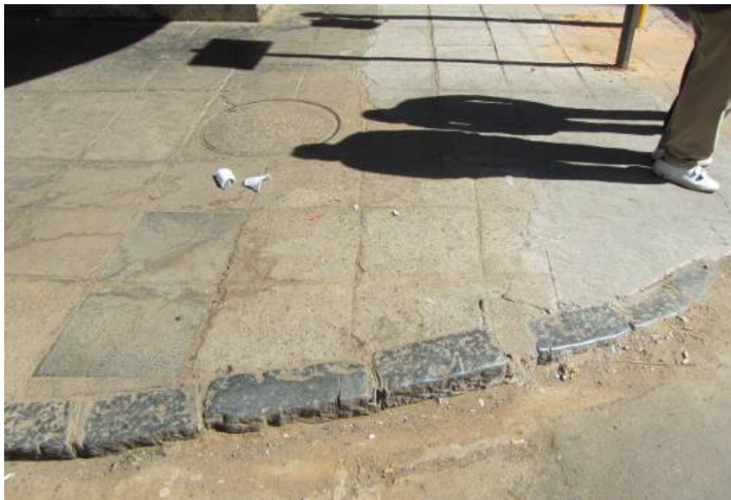
Figure 245. Variety of paving material and granite curbing. (P 1043)
