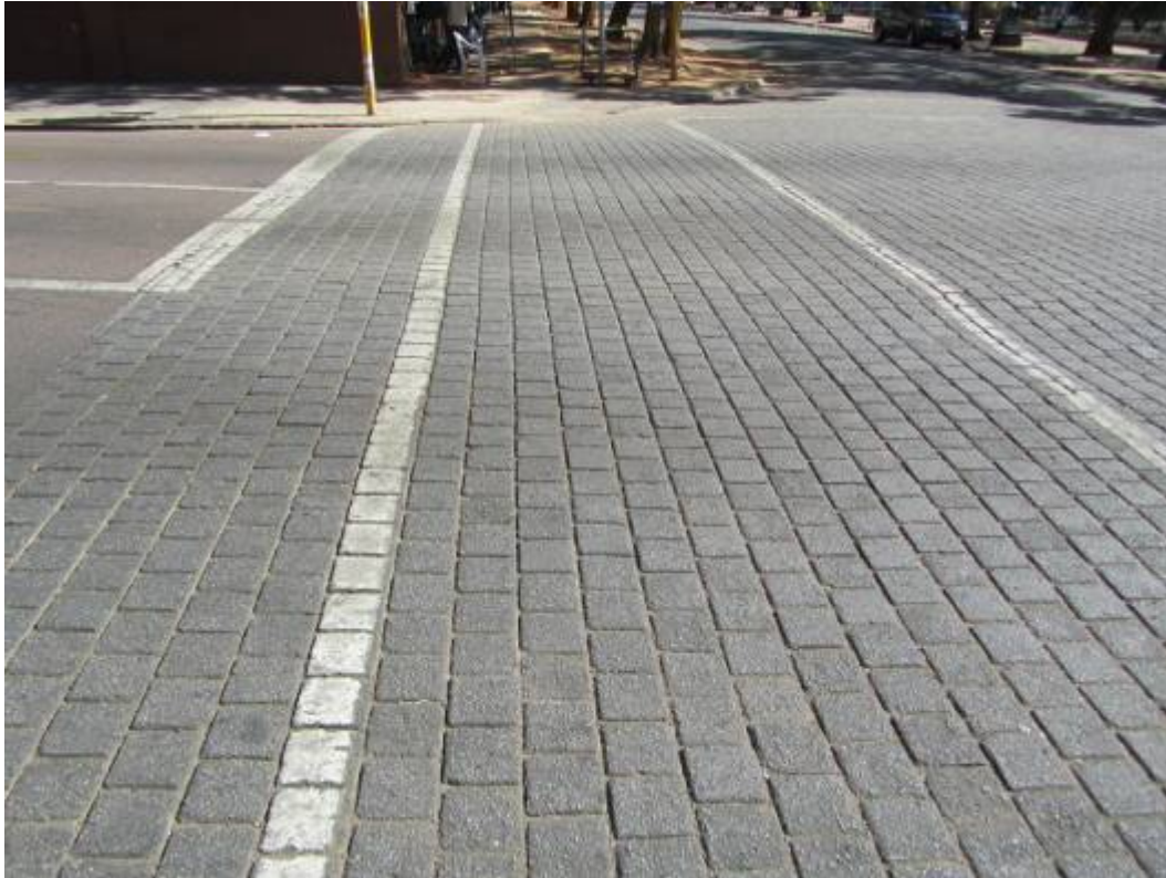
Figure 295. New road paving as part of 'Museum walk' renovation. (P 1120)
