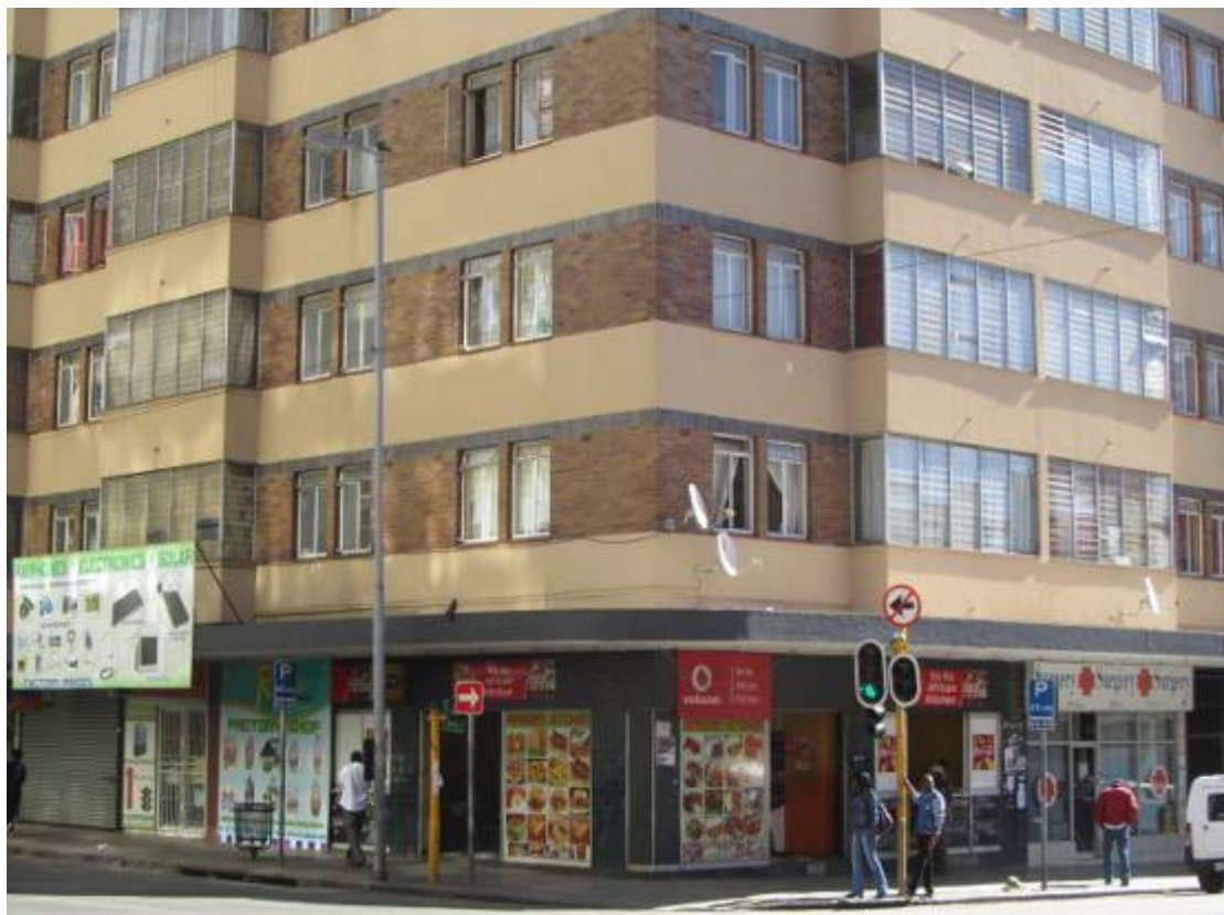
Figure 229. Provisionally protected building. (P 1038)
