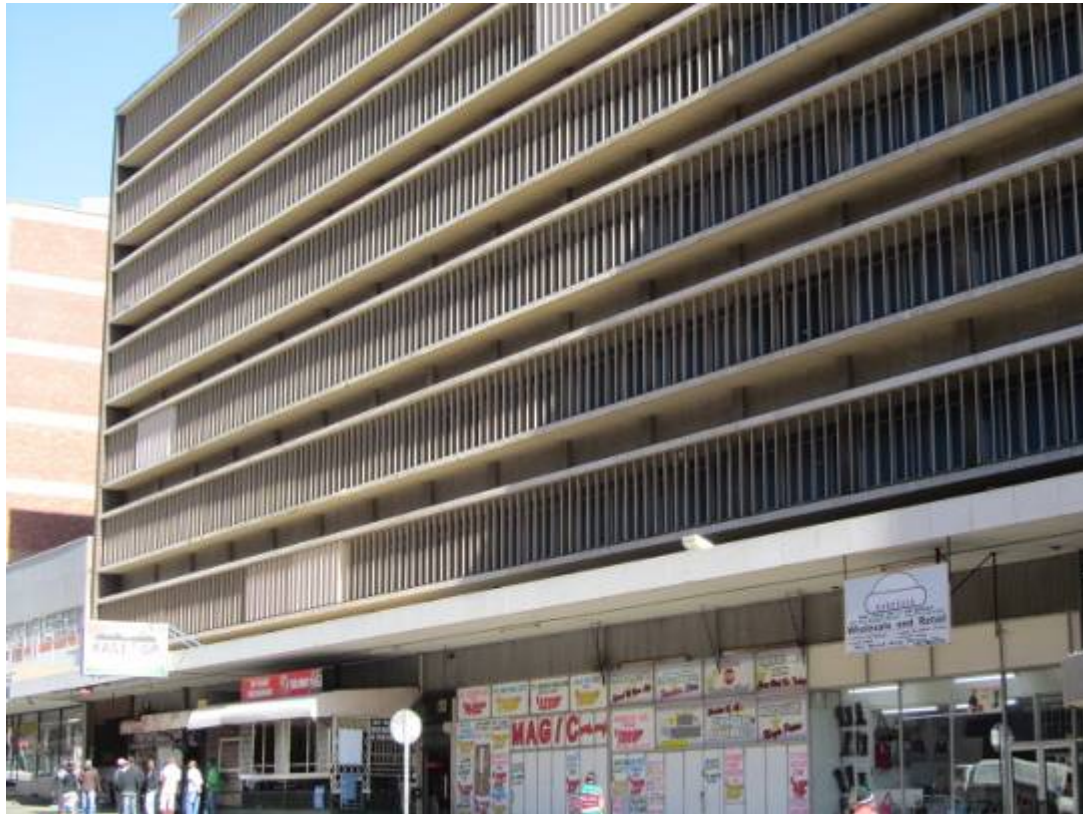
Figure 244. Provisionally protected building. (P 1042)
