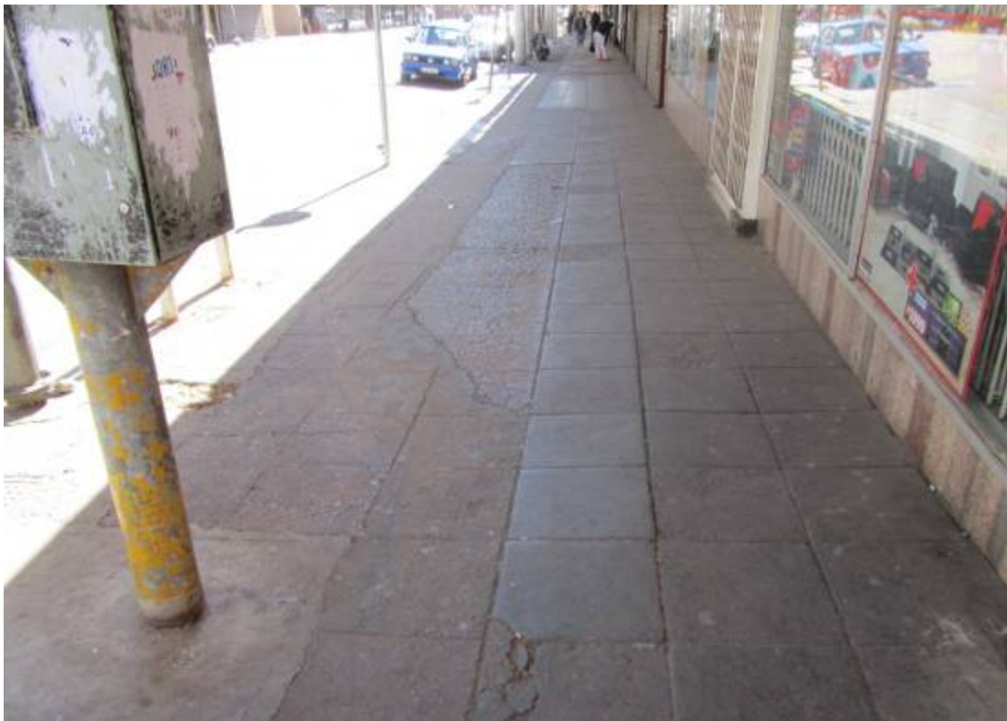
Figure 227. Cement block paving and granite curbing defining old roadway. (P 1027)
