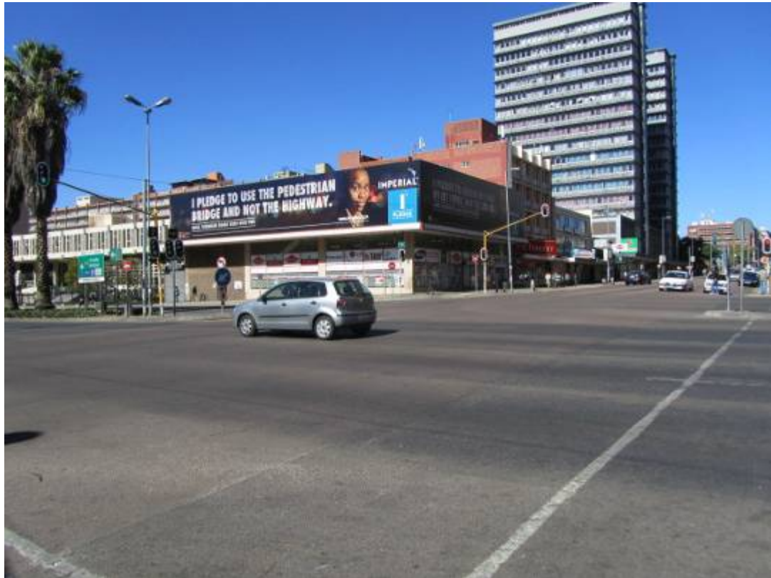
Figure 254. Provisionally protected building (P 1052)
