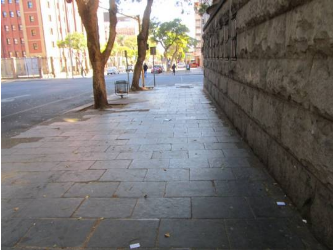
Figure 121. Historical slate paving adjacent to historical building. (P 920).
