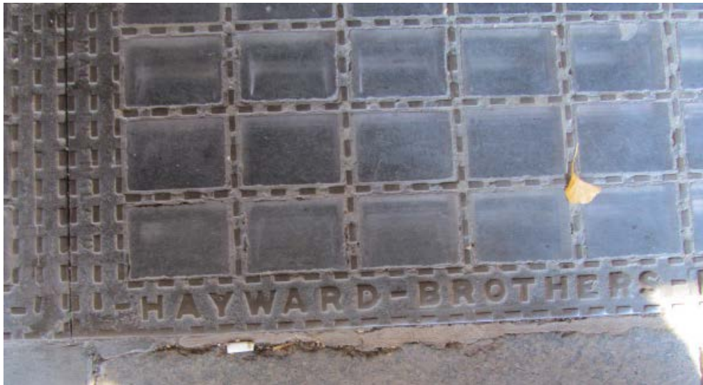
Figure 194. Manufacturer of cellar window for historical building. (P 997).
