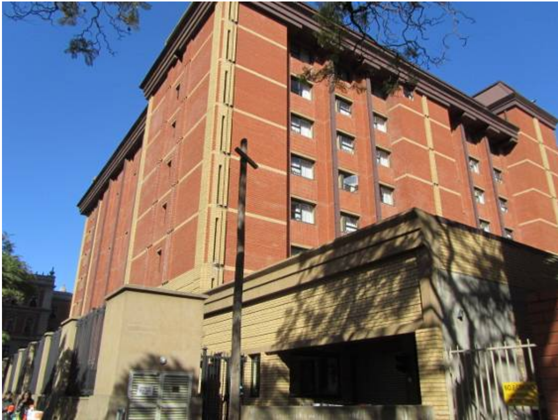
Figure 104. 'Provisionally protected building'. (P 899).
