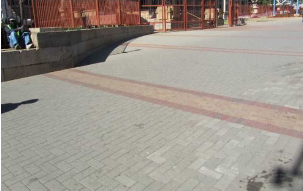
Figure 287. With the renewal of the building some years ago the original paving was removed and replaced. Although attractive and well placed, it is the last option where original paving exist. (P 1085)
