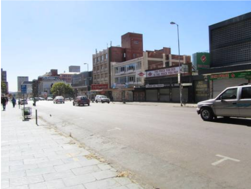
Figure 273. Note extreme variation in height between sidewalk and roadway. Note Granite curbing. (P 1071)
