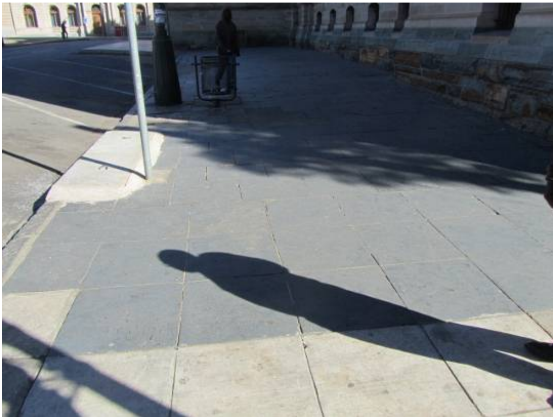
Figure 134. Historical slate paving adjacent to historical building. Note roadway definition with steps of historical building. (P 942).
