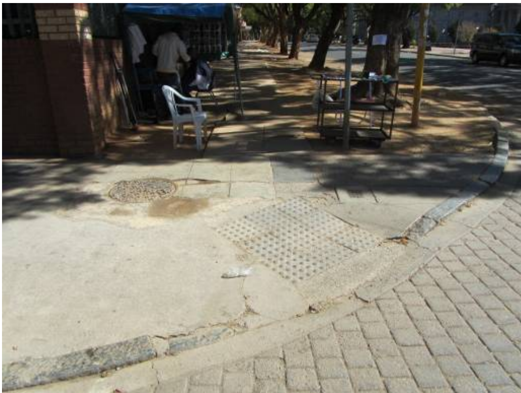
Figure 296. Granite curbing and unsightly paving. (P 1121)
