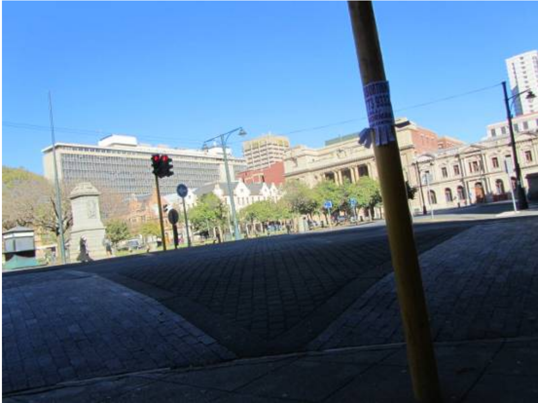
Figure 137. Modern traffic calming structure. Note immense build-up of road surface This may be attributed to the tram lines that is suspected to be still in place. (P 945).
