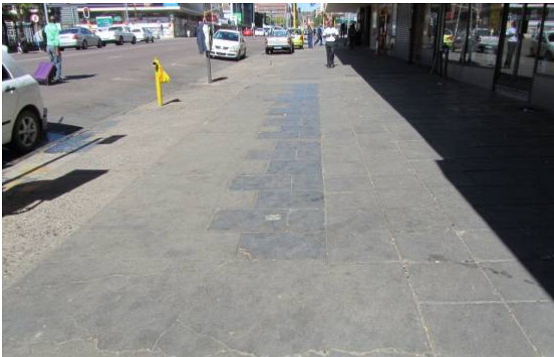
Figure 249. Variety of paving material with remnant of slate paving. (P 1047)
