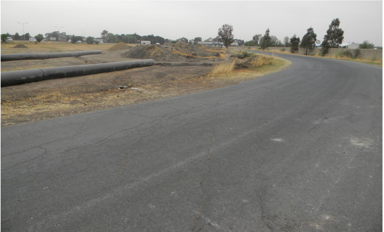
Plate 8: Shows section where they are already installing the pipes.
