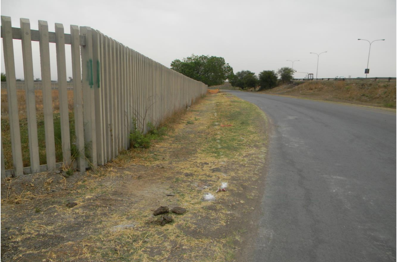
Plates 7: Shows pipeline route
