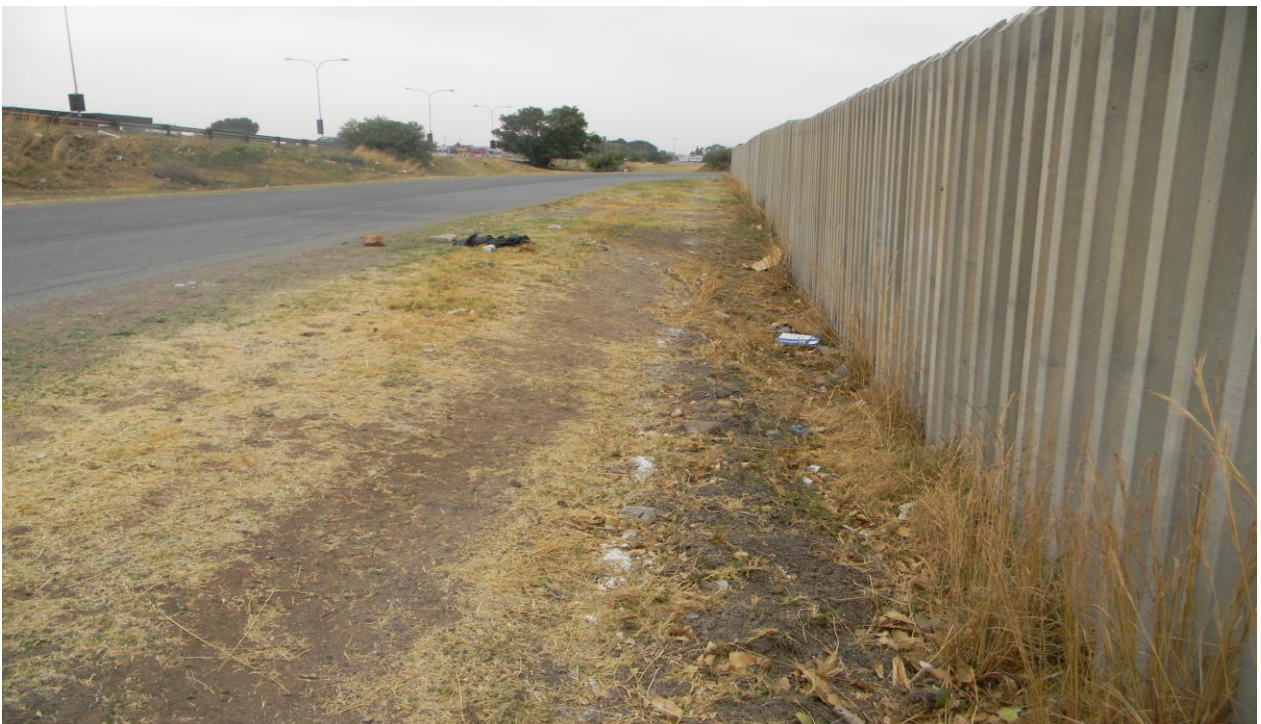
Plates 5: Shows the pipeline route running between road and boundary fence.
