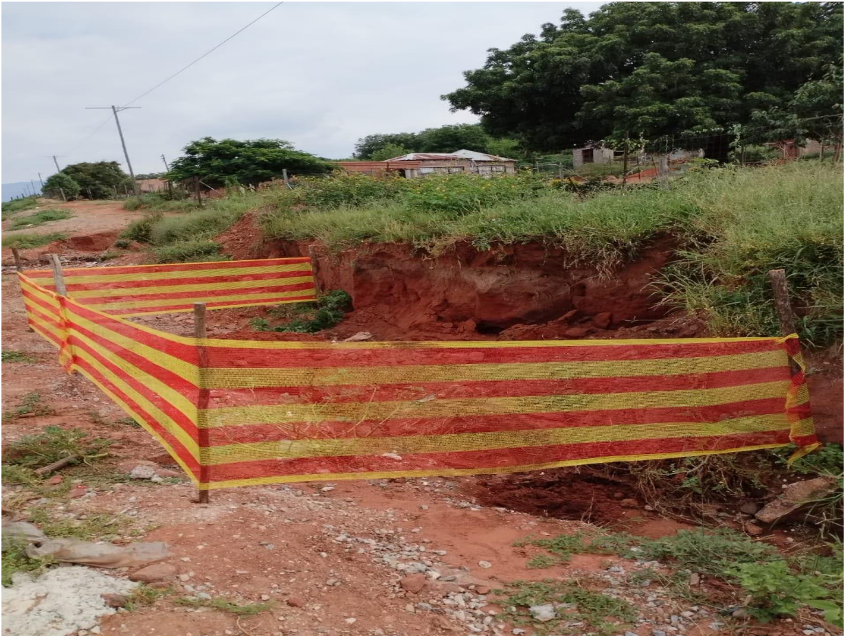
Plates 3: Shows site where human remains were exposed during construction.
