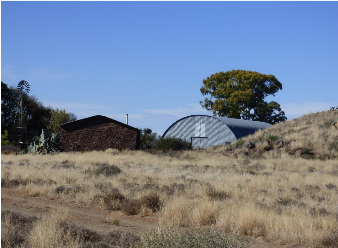
Figure 26: A view of the structures at Site 001 (courtesy Ubique Heritage Consultants).
