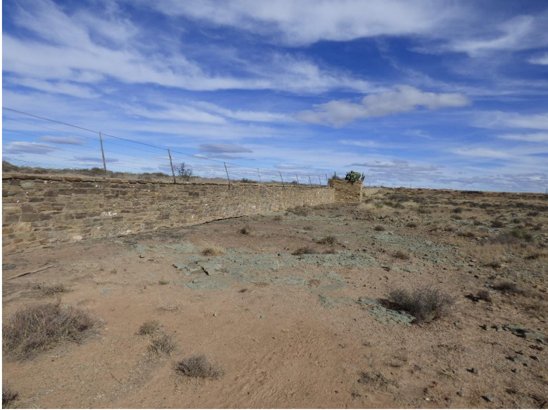
Figure 37: Part of the Site 016 retaining wall (courtesy Ubique Heritage Consultants).
