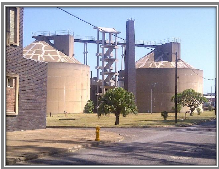
FIGURES 4-7 TYPICAL STRUCTURES WITHIN THE PROPOSED DEVELOPMENT AREA.
