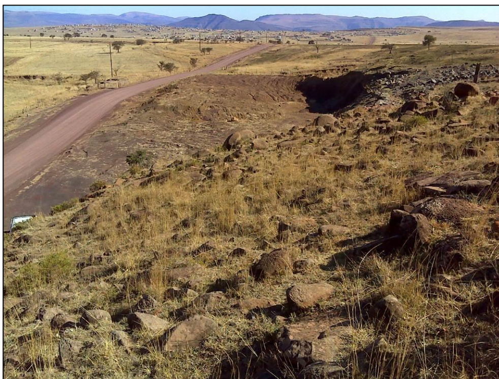
Figure 27. View of the existing Borrow Pit 186 (BP186).
