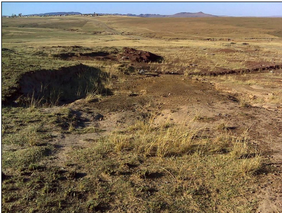
Figure 40. View of the existing Borrow Pit 192 (BP192).
