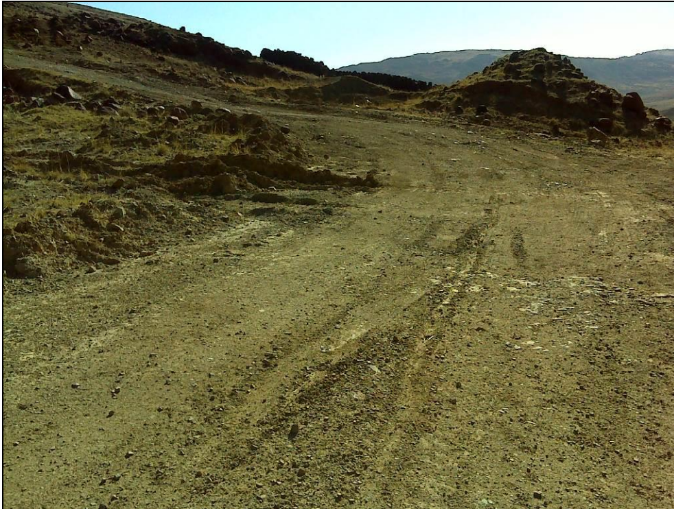
Figure 31. View of the existing Borrow Pit 190 (BP190).
