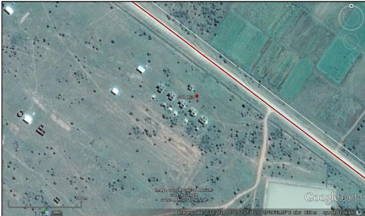
Figure 70. Close-up aerial view of the location of the abandoned structures situated on the property St Marks Mission.
