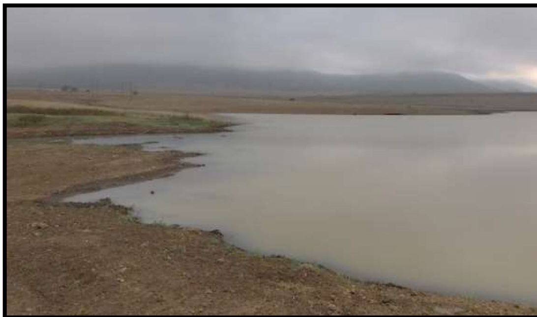
Figure 11. View over Glen Gray Dam.
