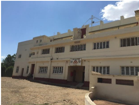
South (front) elevation of ANTOS
