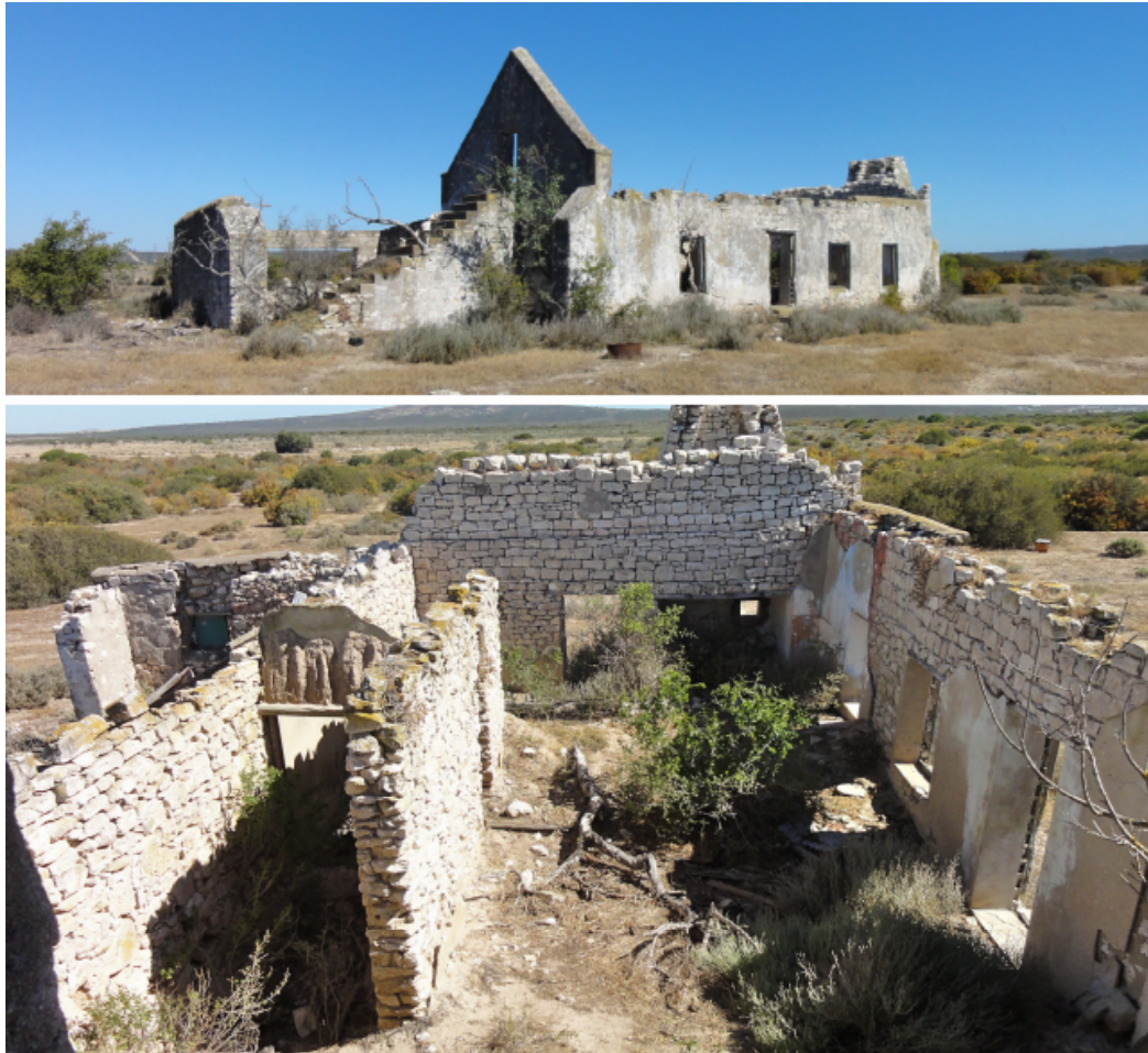
FIGURE 7: Top: the Ondervloer farm homestead located close to the site boundary but off the site. The building is most likely older than 100 years. Bottom: Image taken from the loft door opening looking down into the interior towards the kitchen hearth. The walls are constructed from semi-dressed calcrete of good quality. This structure is regarded as an interesting (historical) archaeological site and could quite probably be graded 3B in these terms. It has not been graded as an architectural heritage resource.
