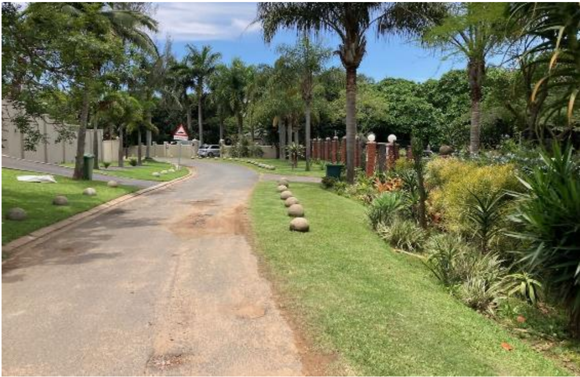
Figure 6: Section of Garden Road with boundary walls visible
