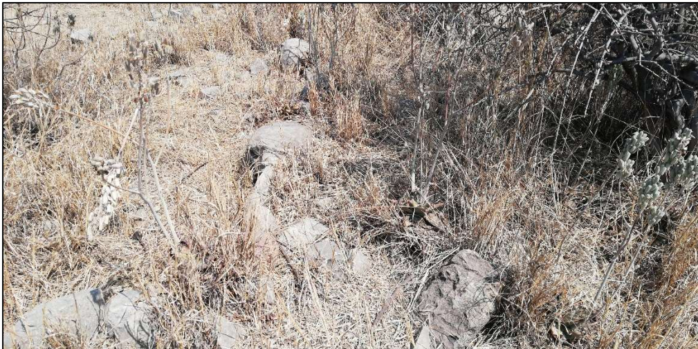
Figure 21: Unclear stone walling at Site B01.
