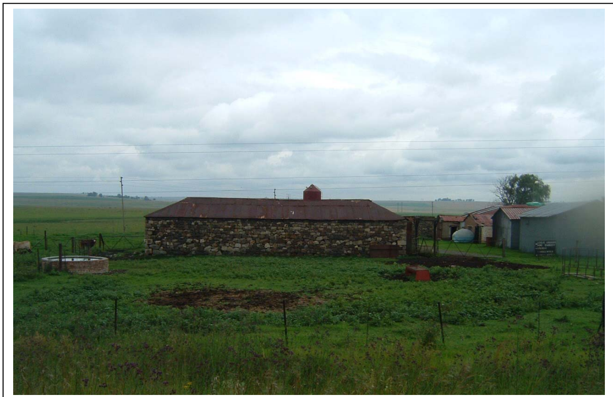
Figure 10- A wagon shed constructed with sandstone on Rietkuil 531IR next to the Leandra-Balfour road (above).
