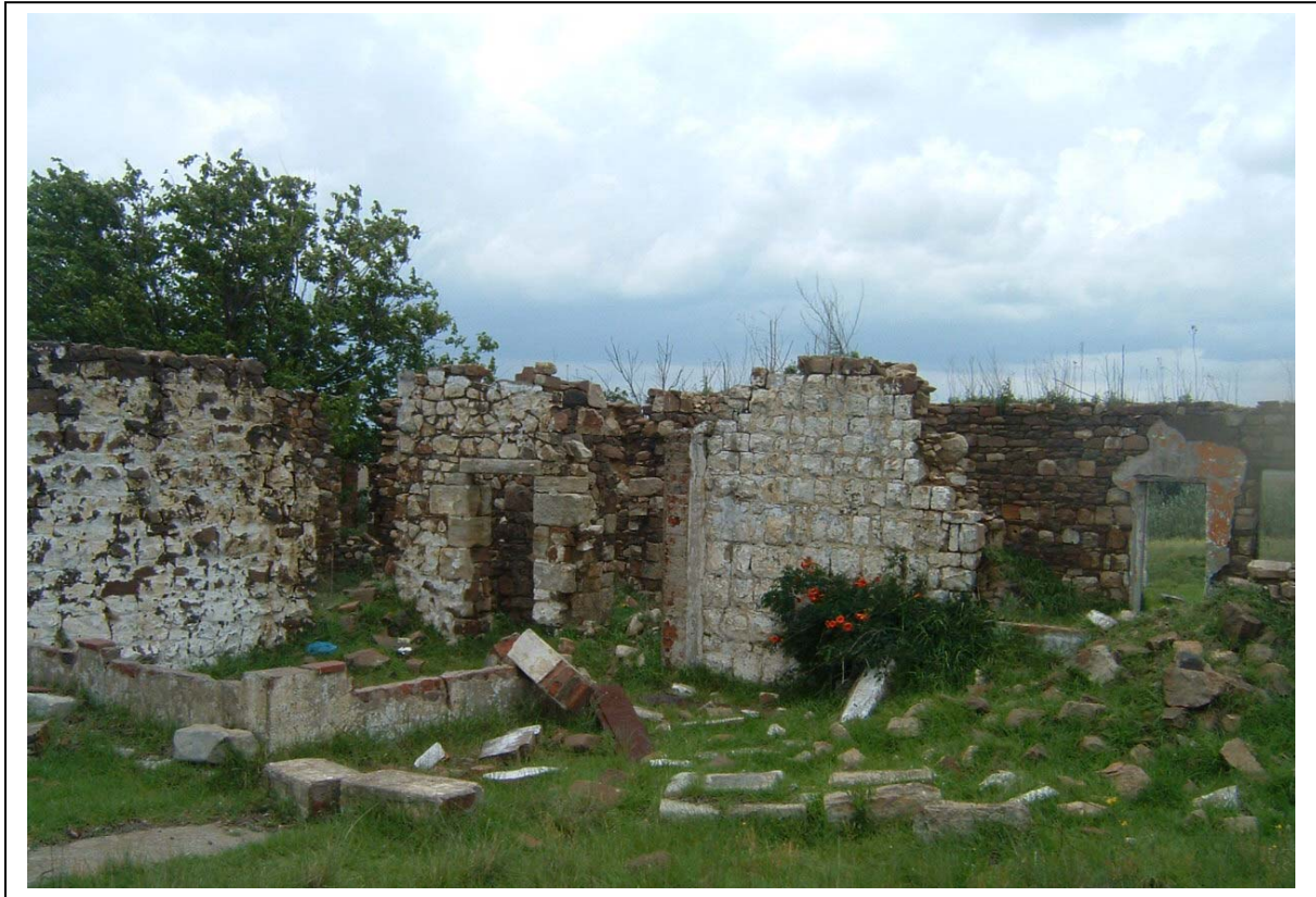
Figure 4- The main residence in FC01 on Kromdraai 128IS consists of a residence which was built with sandstone bricks and dolerite stone (above).
