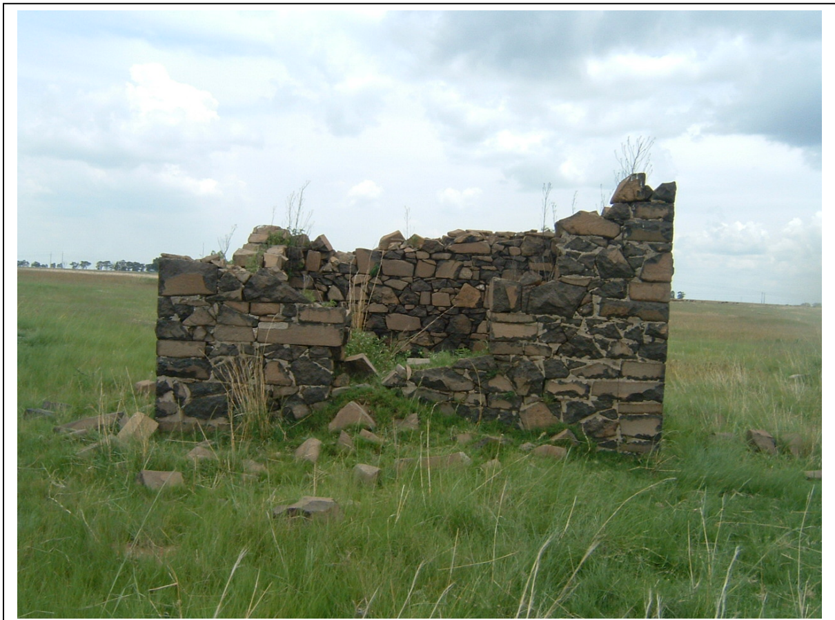
Figure 7- A possible 'bywonershuis' or a cool room ('koelkamer') in FC03 on Witkleifontein 181IS which was constructed with dolerite stone (above).
