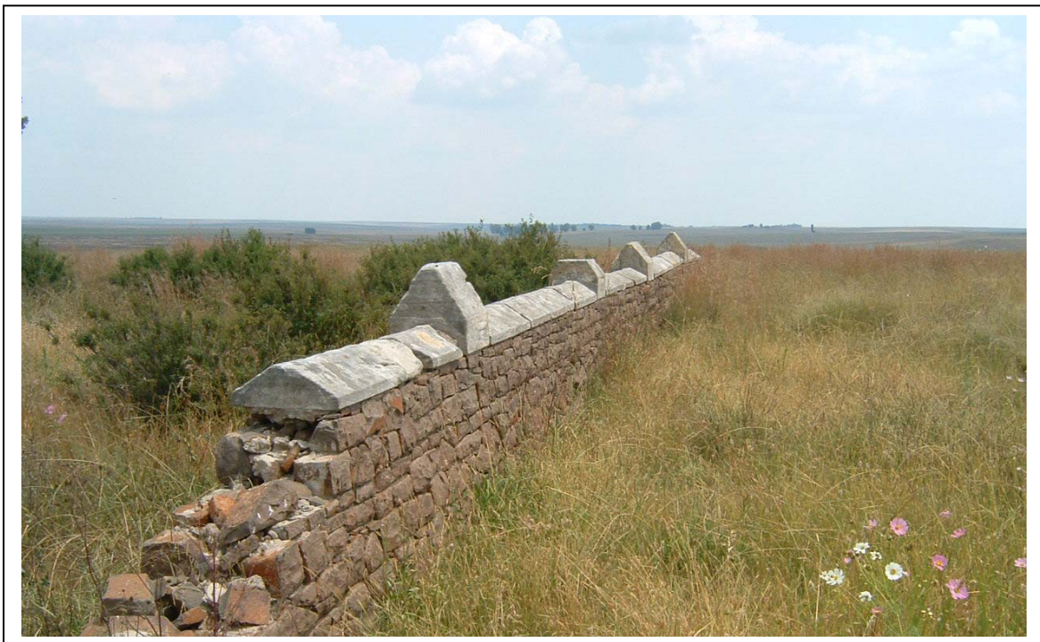
Figure 23- The wall around GY20 is constructed with dolerite which is capped with sandstone trimmings (above).
