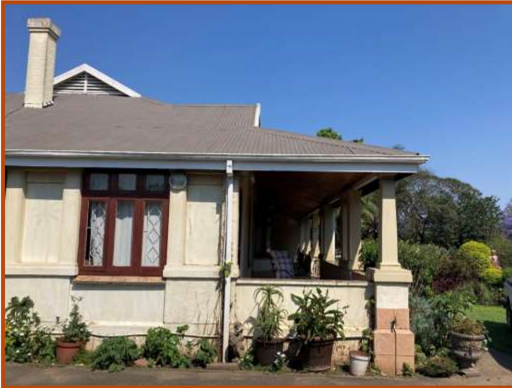
Figure 12: This is a side view of the property revealing more architectural detail. Notice the vent gables on the high steep roof close to chimney. These were intended to well ventilate houses by allowing in a lot cool air and letting out hot air. These were particularly significant in corrugated iron roofs that absorb a lot of heat. Such vent gables were a key characteristic of Victorian buildings.
