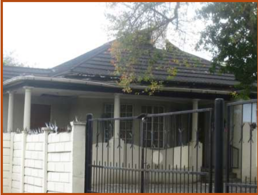
Figure 6: A view of the property clearly revealing the Hip and Gable traits on the roof
