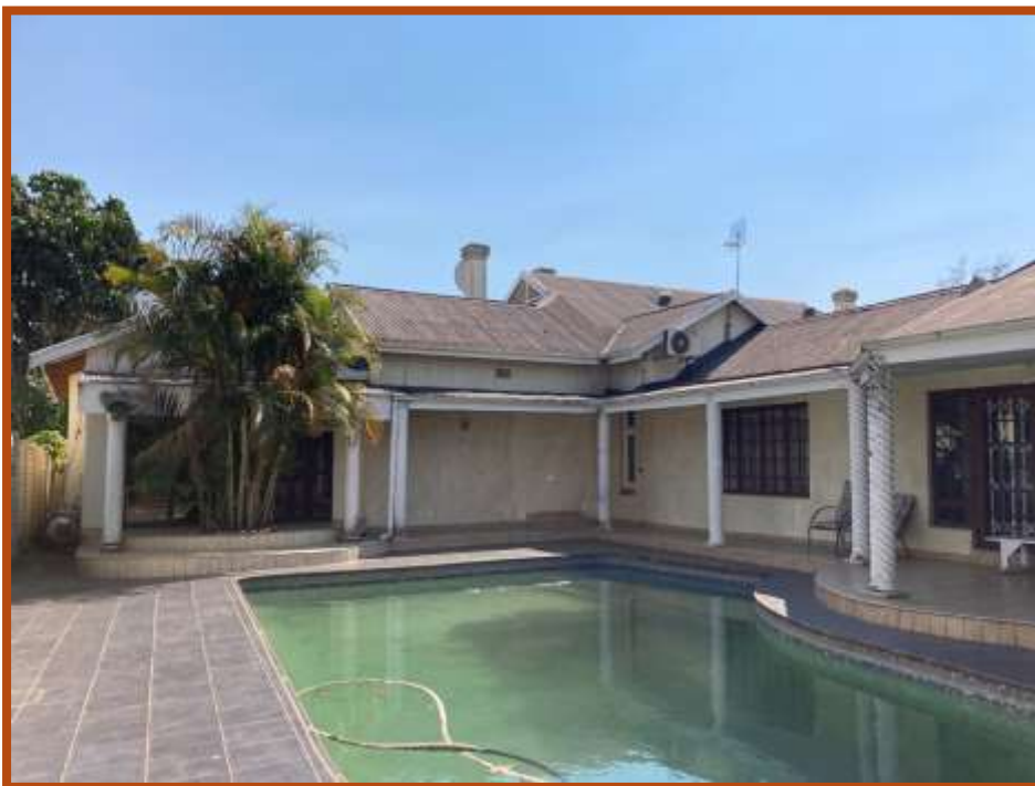
Figure 14: Property on 70 New England Road. Notice the steep roof near the chimneys on either side. The façade of the house is strongly reminiscent of Victorian period houses in Pietermaritzburg.
