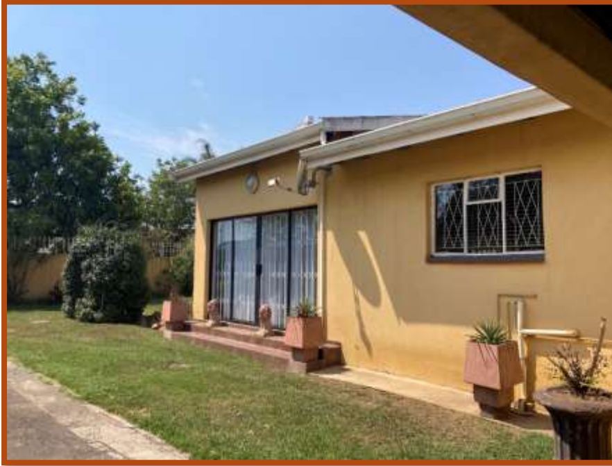
Figure 21: This elevation of the property does not show any feature of architectural significance. Notice modern window seals and an extensive glass door. This suggests recent retouching of the property.
