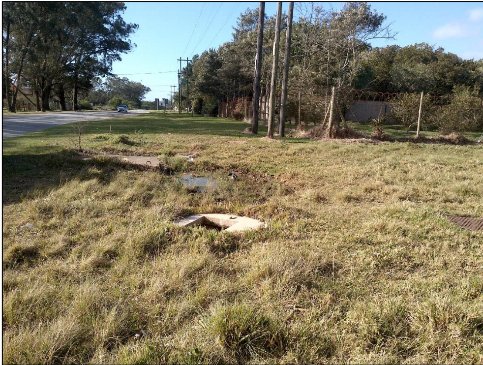
Figure 6. View of the route for the proposed infrastructure north of the N2 national road facing north.
