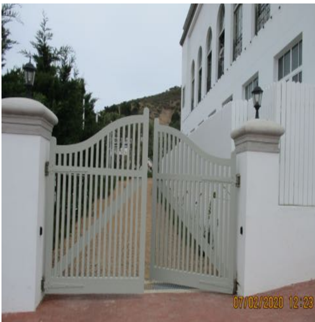
Figure 7: gate and pillars spanning Signal Street
