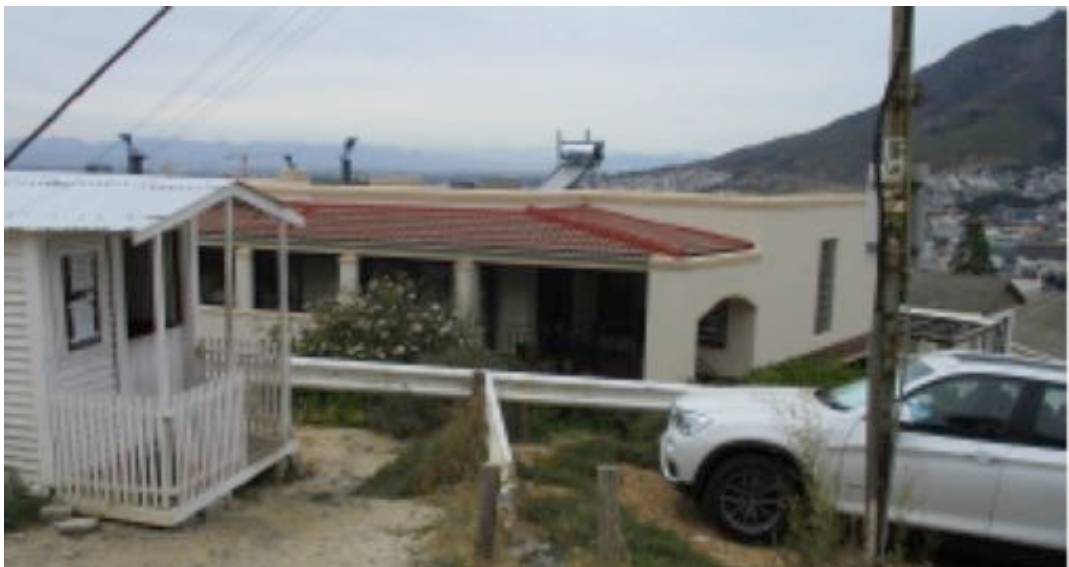
Figure 10: side elevation of the building to LHS in Figure 9
