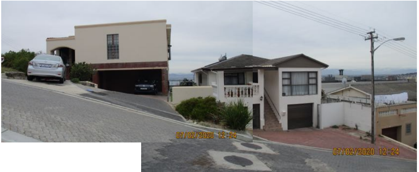
Figure 9: composite photograph showing the buildings directly across the road from the new building
